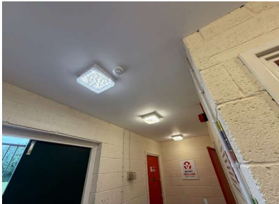
View of the existing light fittings. 1 no light fitting has been replaced for LED.
