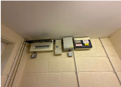
View of the existing electrical distribution board.
