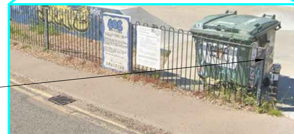
Finishing post of redecoration and replacement works to the bow top fence.
