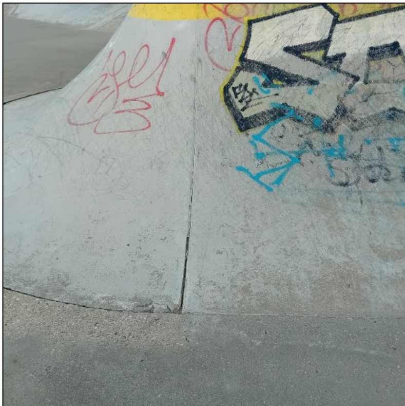
6 · Cracked Curved Ramp Base Allowed quantity: 20m
