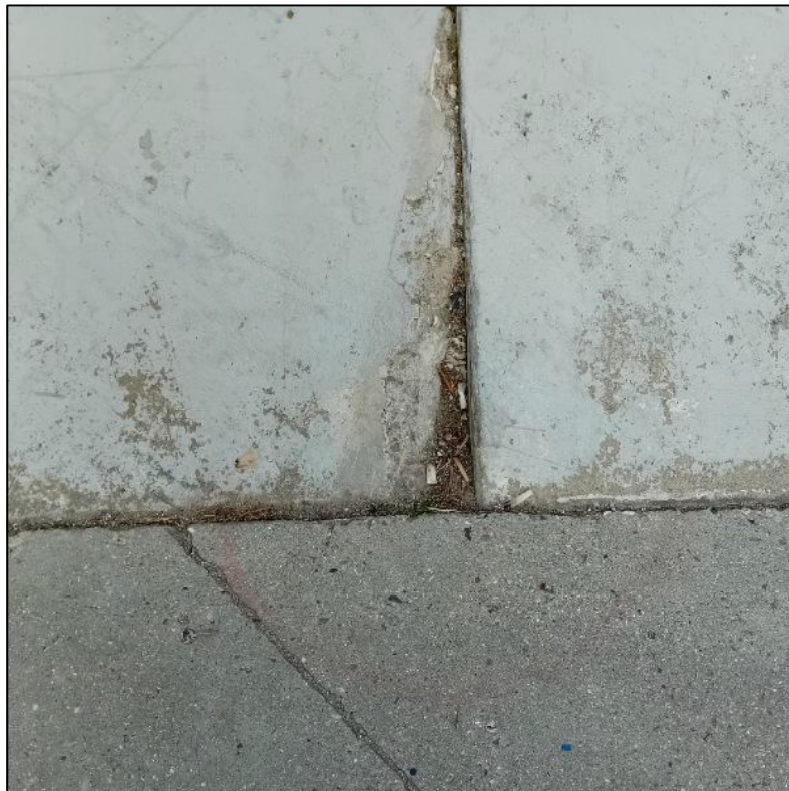
3 · Cracked Joint Between Slabs Allowed quantity: 40m
