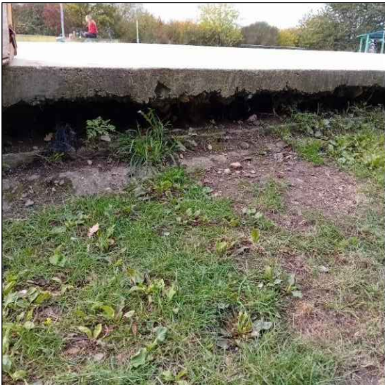
5 · Edge Ground Bearing Slab Eroding Away Allowed quantity: 30m
