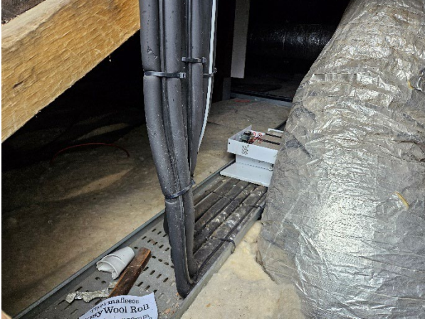
Image: Town Hall Roof Void
