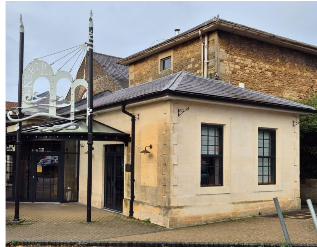
View of the entrance to Neeld hall showing the various volumes that make up the venue. In the foreground is the 1996 extension with Ashlar stone, with historic masonry structures beyond. The gable wall and slate pitched roof of the hall itself is visible beyond.
