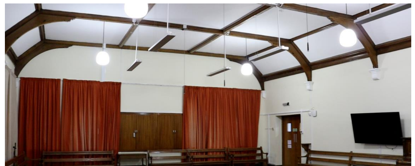
Examples of electric radiant heating in a church (above) and a village hall (below). Images courtesy of Herschel.
