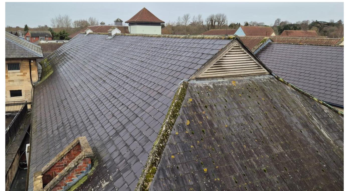
Neeld hall roof with louvres at ridge level and at the gable. It's not known if these are used.
