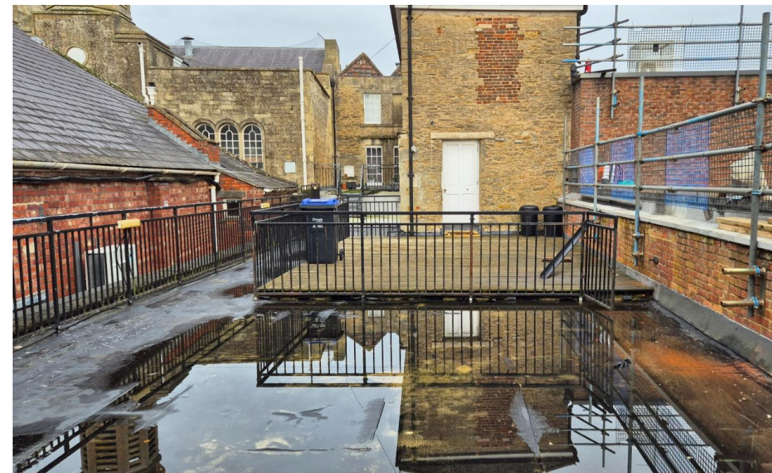
Roof above the old bar. The Neeld Hall is visible to the left and the Town Hall in the distance (left)
