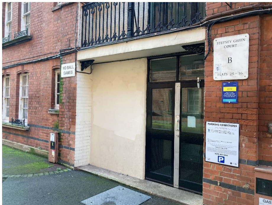
Typical block entrance from courtyard area
