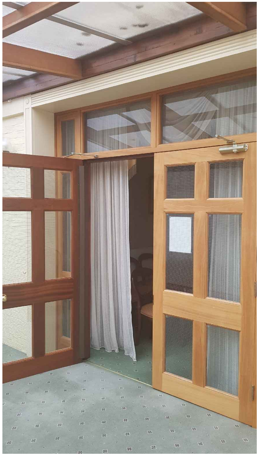
Photo of Existing GF06 Ceremony Room Door
