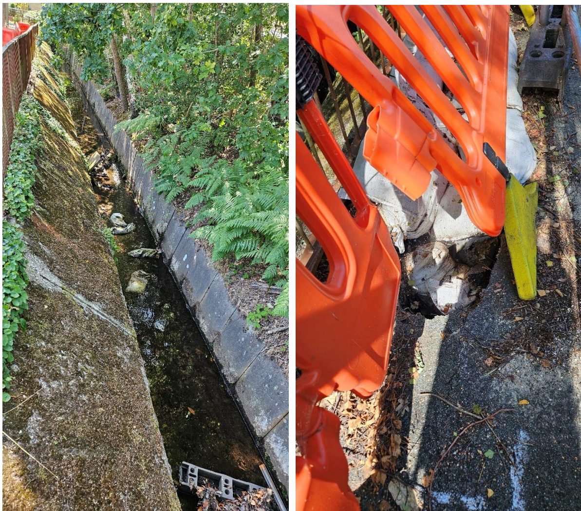
Plate 8-9 showing Section 3 of down-stream after footpath undercut
