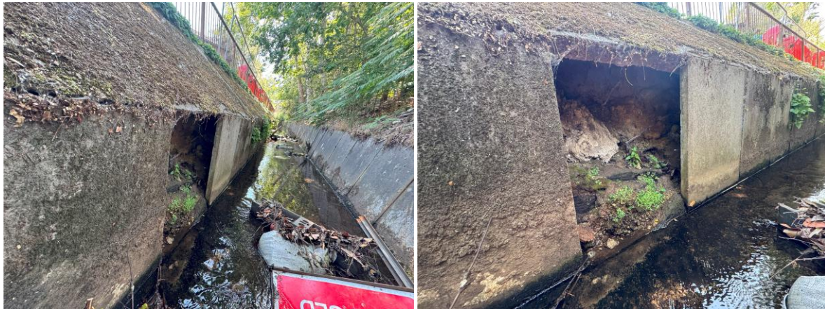
Plate 10-11 showing Section 4 of down-stream after footpath undercut
