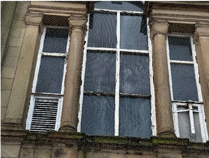
Photo 45 - Dampness and weathering to stone
