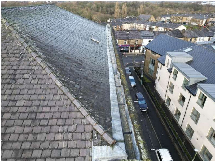
Photo 13 – Lead lined gutter behind parapet wall
