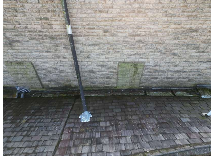
Photo 8 – Rainwater pipe penetrates roof to front block
