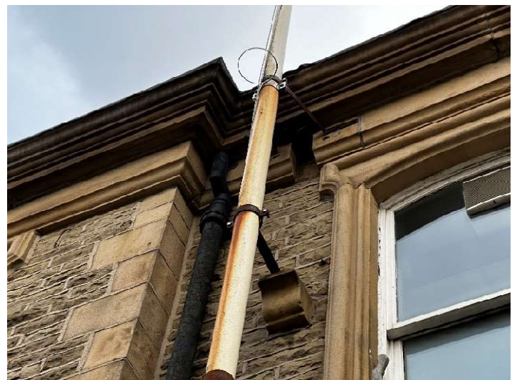
Photo 6 – Paintwork to cast iron rainwater pipe in poor condition
