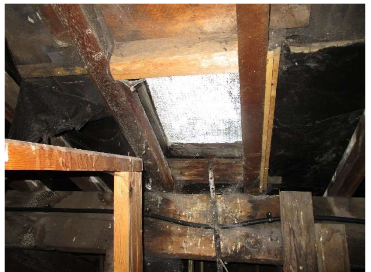
Photo 82 – Visible moisture to rafters
