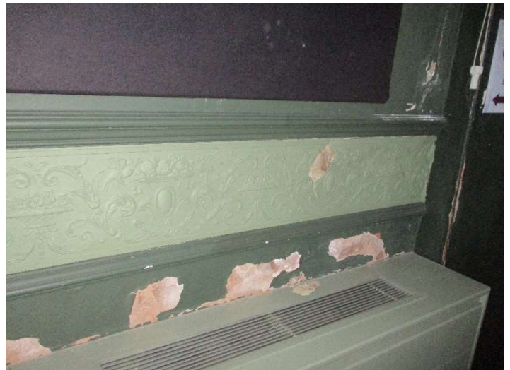
Photo 88 – Rear block - dampness to wall to right side elevation
