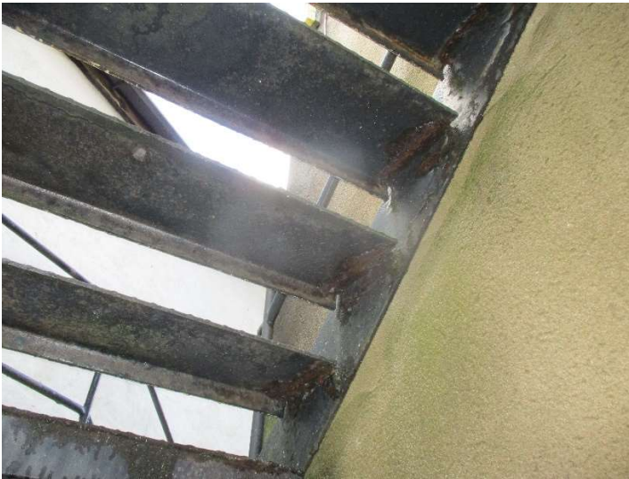
Photo 98 – External staircase corrosion to treads
