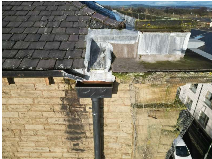
Photo 14 – Lead spitter to hopper
