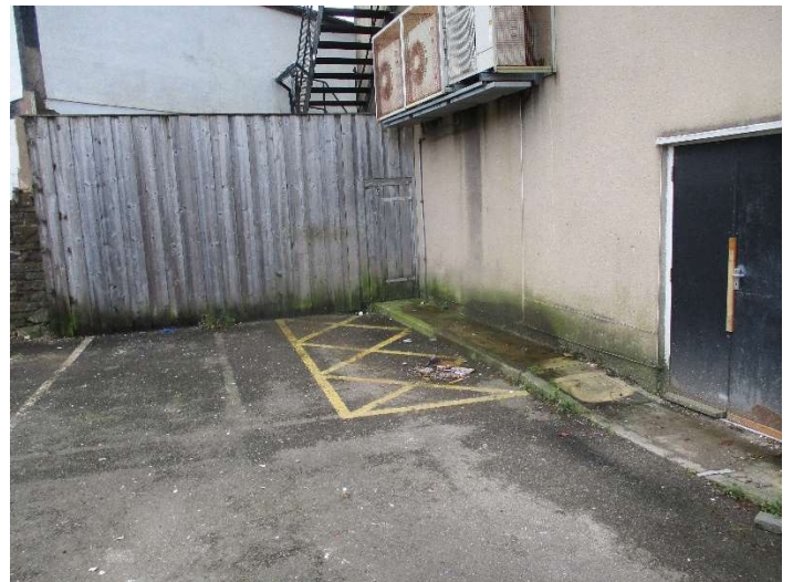
Photo 111 – Timber fencing damp at low level
