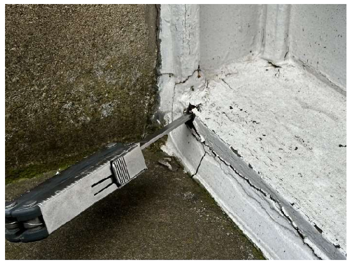
Photo 60 – Wet rot timber decay to window frame
