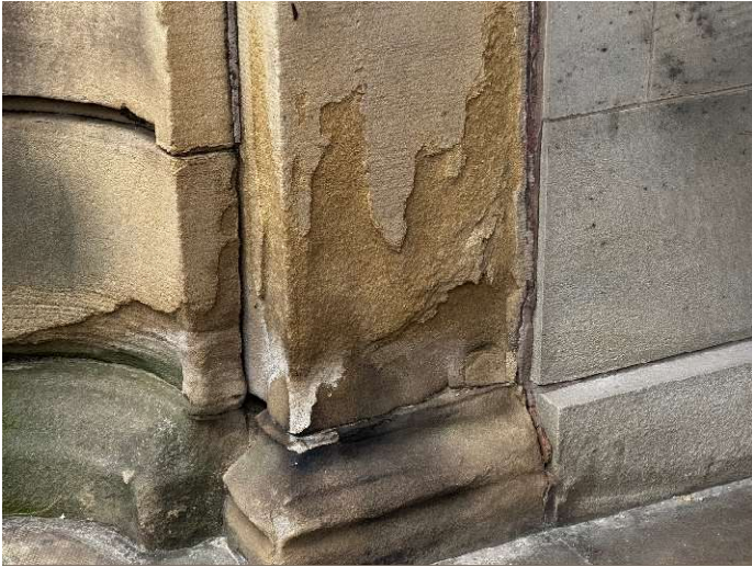
Photo 25 – Weathered dressed stone
