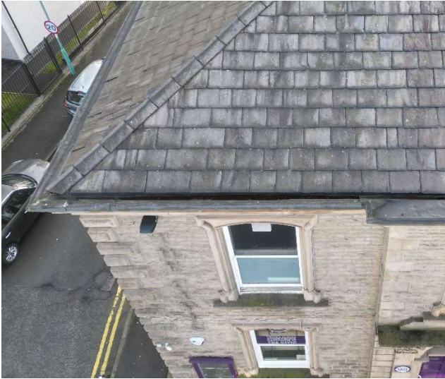
Photo 1 – Bitumen felt lining to gutters
