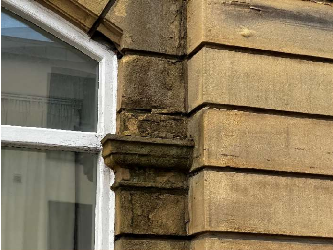
Photo 45 - Dampness and weathering to stone
