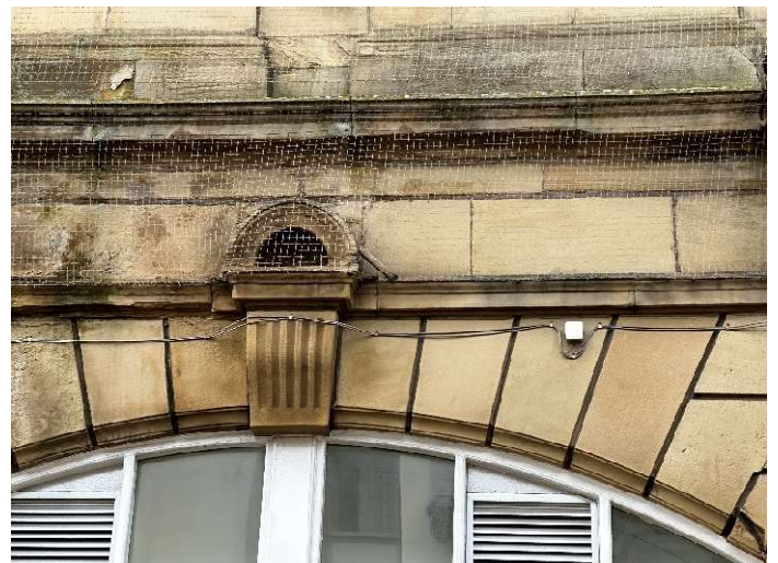
Photo 44 - Dampness and weathering to stone
