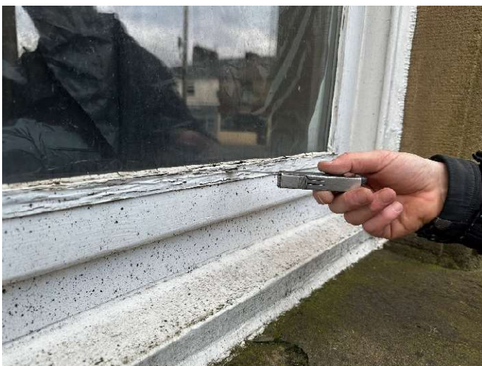
Photo 59 – Wet rot timber decay to beading
