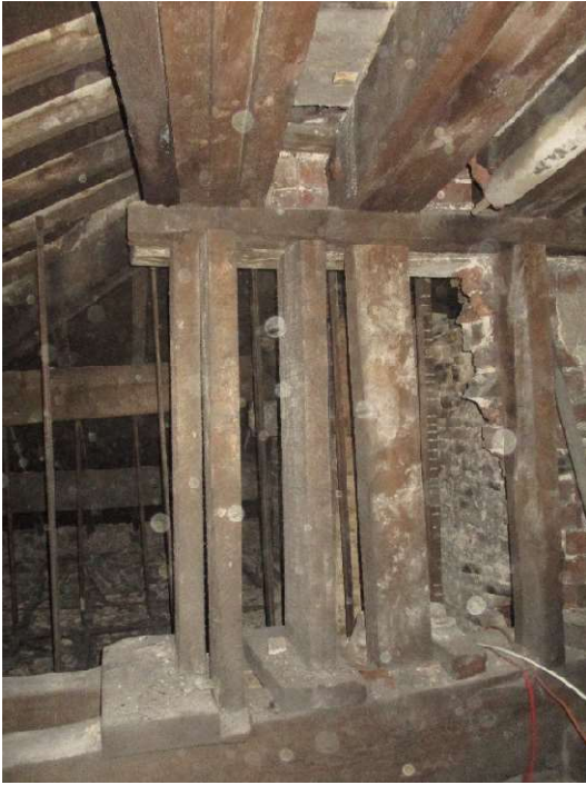
Photo 73 – Front Block - flat roof structure
