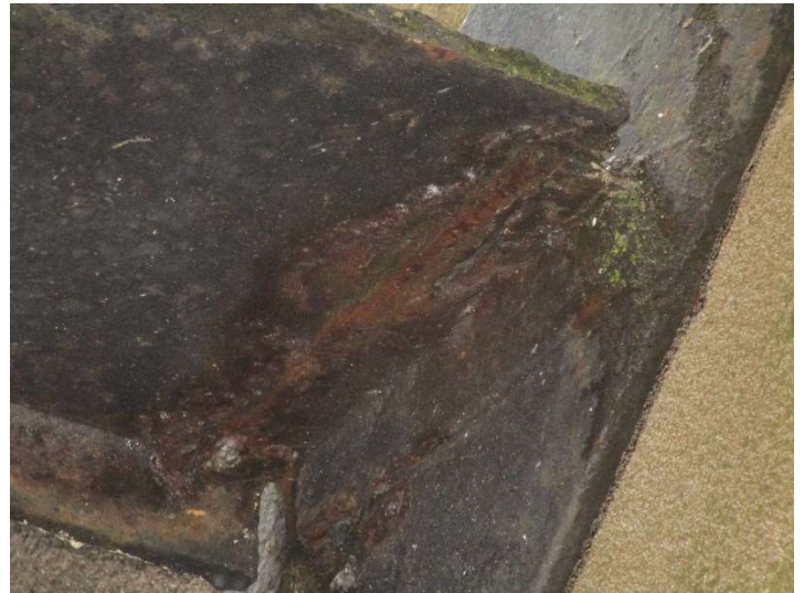
Photo 99 – External staircase corrosion to treads
