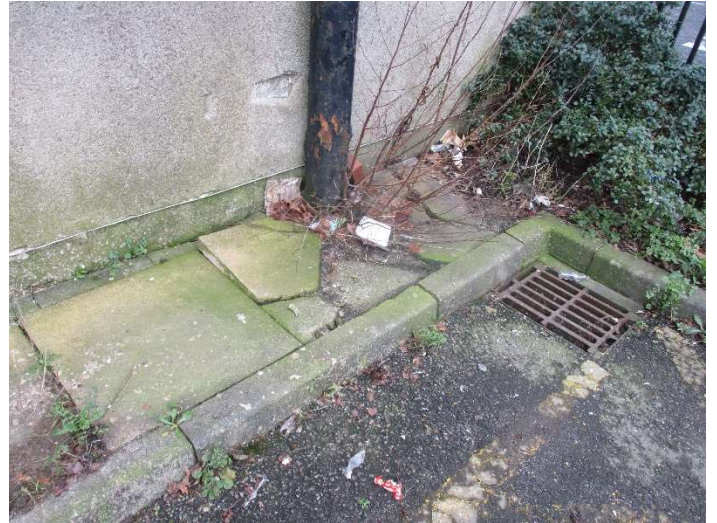
Photo 109 – Concrete paving slabs, vegetation to remove
