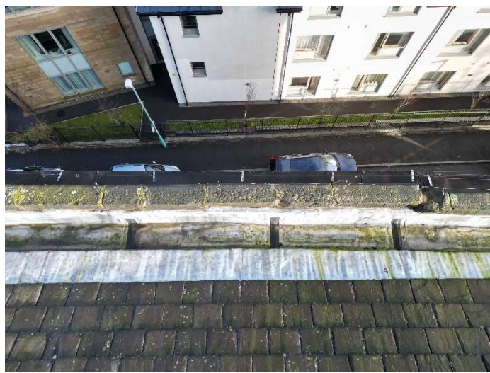
Photo 16 – Joints to leadwork sealed with bitumen strips
