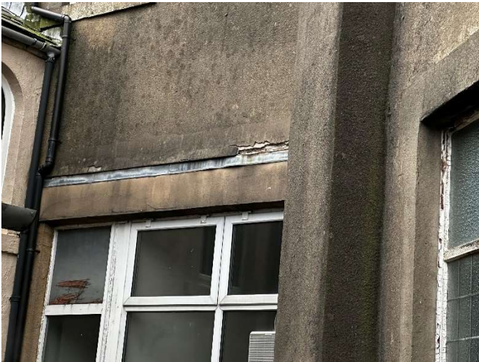
Photo 33 – Defective render to rear of front block
