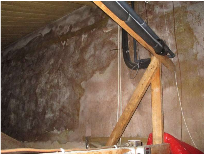
Photo 87 - Rear block - dampness to wall to rear elevation
