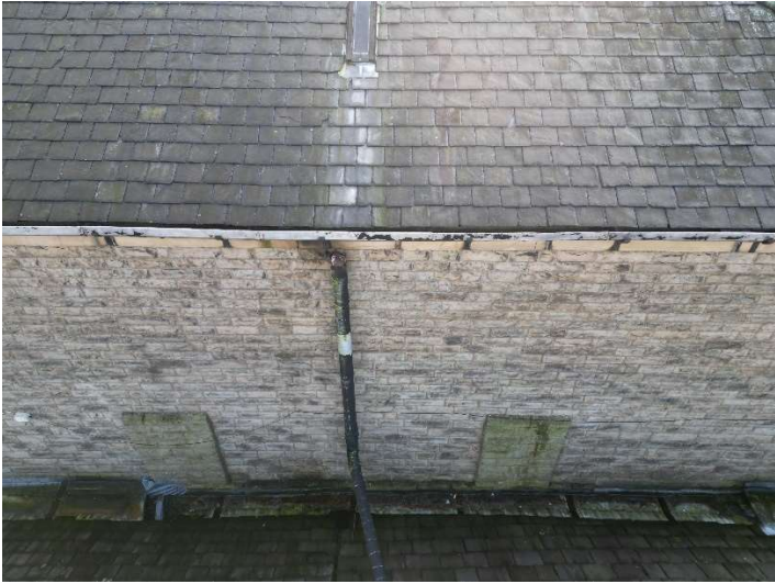
Photo 7 – Paintwork to aluminium gutter in poor condition
