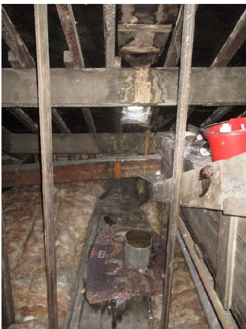
Photo 83 – Water ingress above roof light
