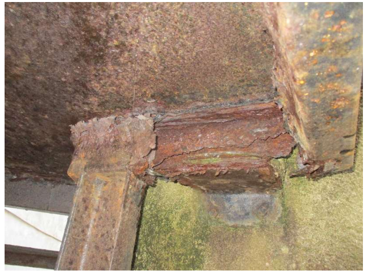
Photo 98 – External staircase corrosion to framework
