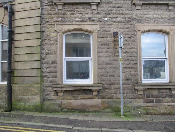
Photo 31 – Structural movement at junction between front block and rear block stone window sill and head cracked
