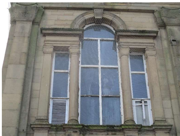
Photo 66 - Painted timber first floor windows to main frontage
