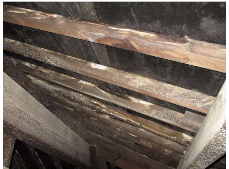
Photo 82 – Visible moisture to rafters
