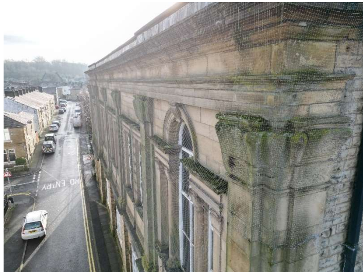
Photo 38 – Dampness and weathering to stone at high level
