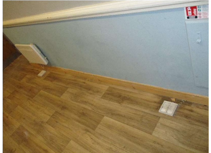
Photo 86 – Surface mounted floor vents to rear corridor
