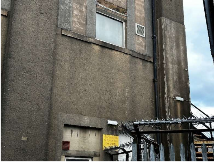
Photo 55 – Cracking to render
