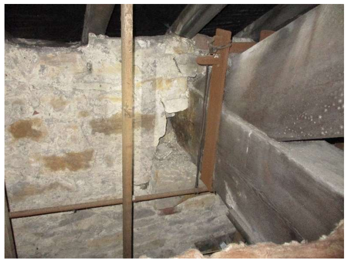
Photo 78 – Bearing ends of trusses appear discoloured and damp
