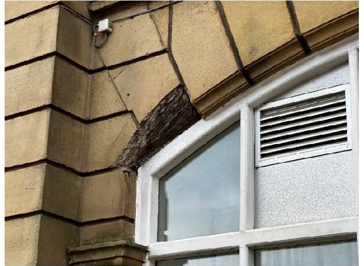
Photo 46 – Damaged section of stone
