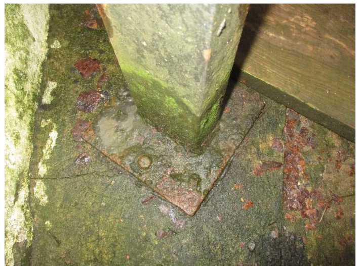
Photo 96 - External staircase corrosion to base plate
