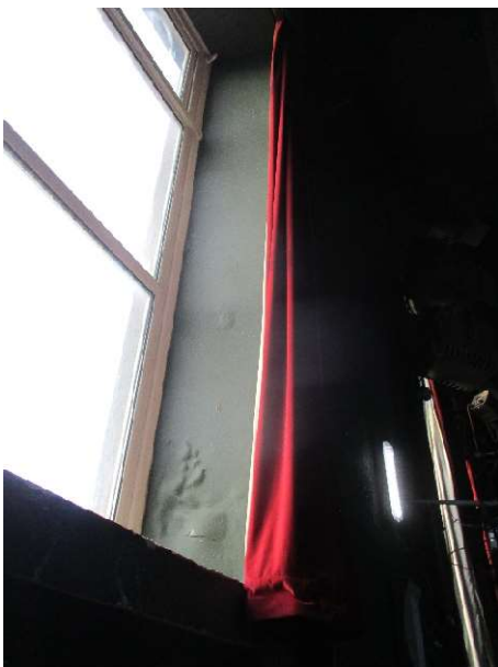
Photo 89 - Rear block - dampness to wall at window reveals
