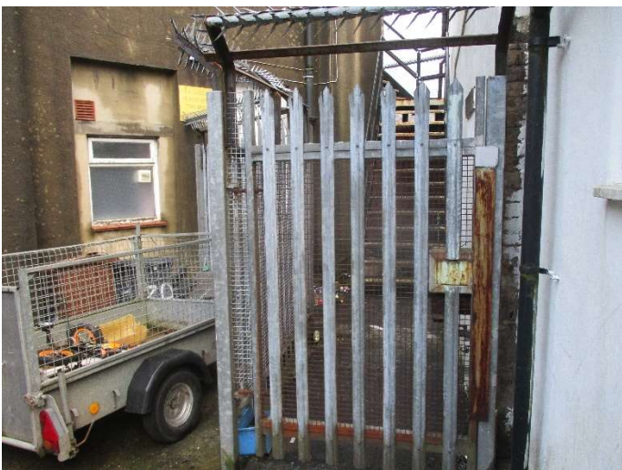
Photo 112 – Steel palisade fencing
