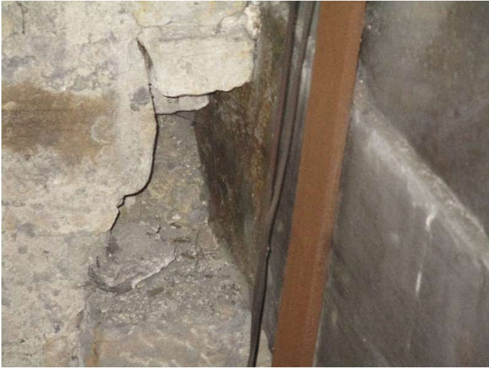
Photo 79 - Bearing ends of trusses appear discoloured and damp
