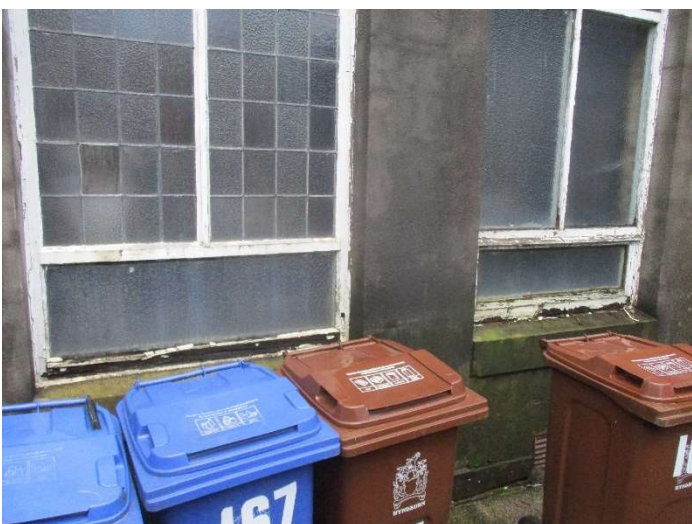
Photo 63 – Rotten windows to right side elevation
