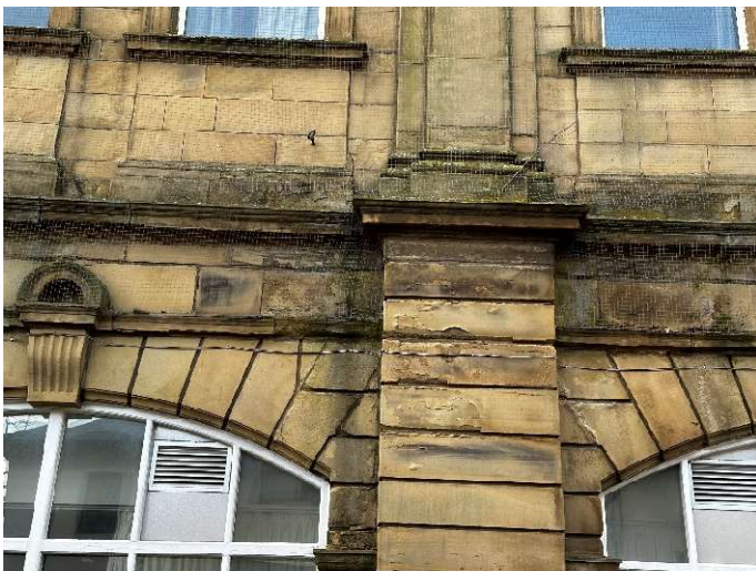
Photo 43 – Dampness and weathering to stone
