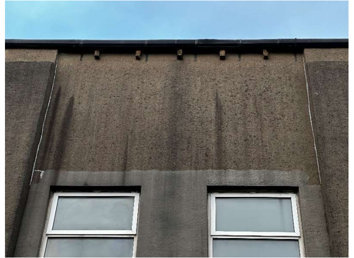
Photo 56 – Buttresses sealed at junction with main wall
