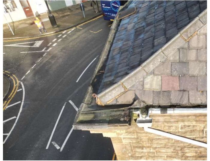
Photo2 – Corroded cast iron visible underneath bitumen roofing felt
