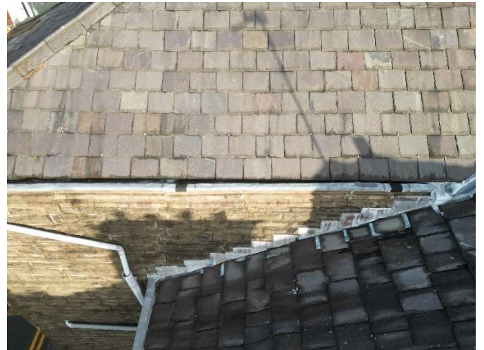
Photo 4 – Leadwork lining to gutter
