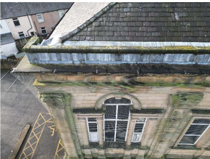
Photo 47 - Dampness and weathering to stone
