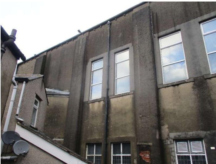
Photo 55 – Cracking to render
