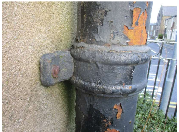
Photo 12 – Defective fixing for cast iron rainwater pipe
