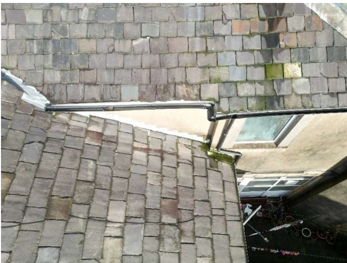
Photo 5 – uPVC gutter with failed joint
