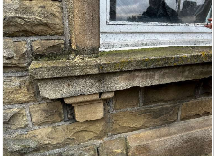
Photo 32 – Stone window sill cracked
