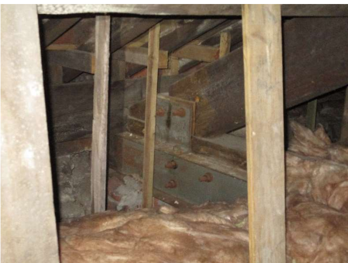
Photo 77 – Steel plates added to bearing ends of rafters
