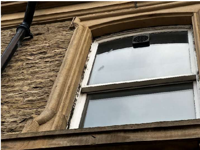
Photo 61 – Failed sealant to window perimeter
