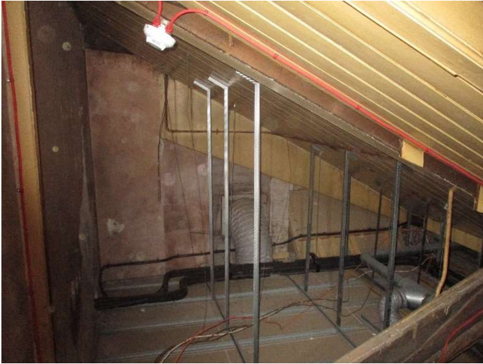
Photo 85 – Timber trusses supporting balcony seating area
