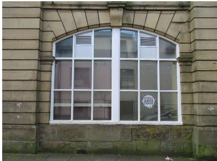
Photo 62 – Painted timber ground floor windows to main frontage
