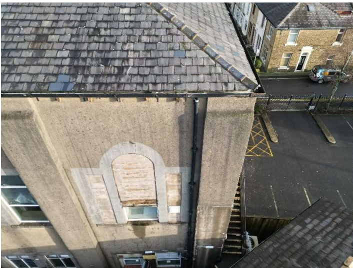
Photo 9 – Painted aluminium gutter
