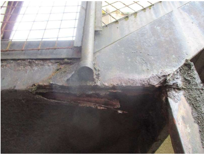
Photo 97 – External staircase corrosion to landing
