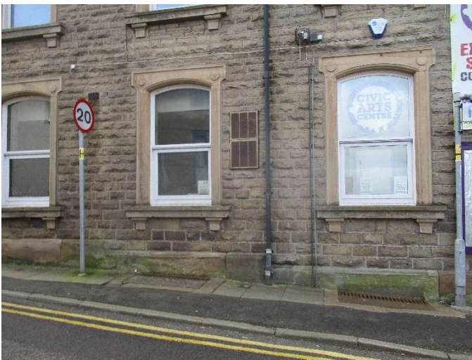
Photo 21 – Damp and weathered stone plinth
