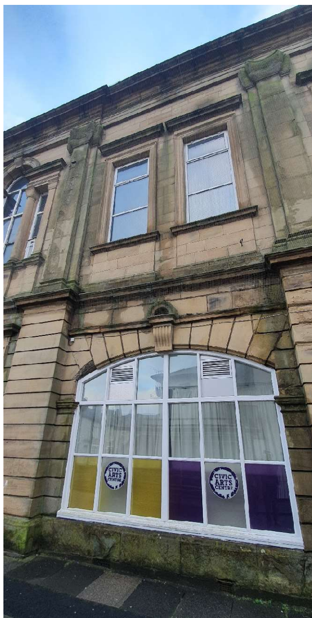
Photo 40 - Dampness and weathering to stone
