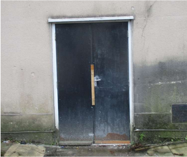
Photo 67 – Painted timber double doors in poor condition
