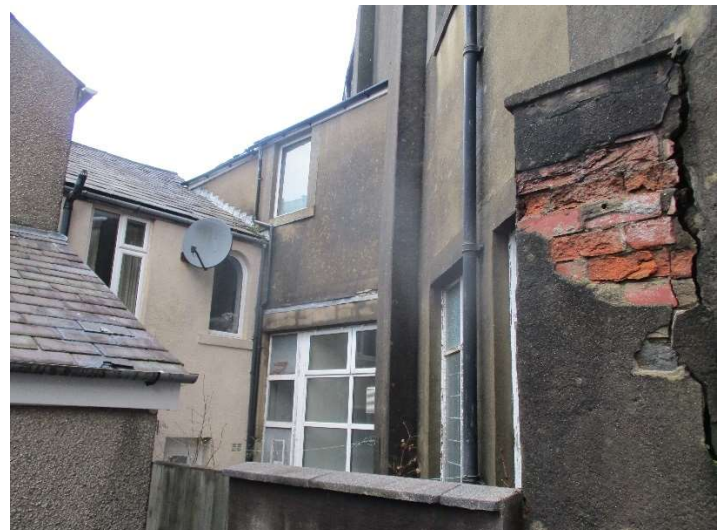
Photo 56 – Buttresses sealed at junction with main wall
