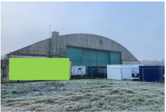
Eastern Elevation of L2 Hangar – Waterproof membrane to be applied to the solid surfaces including the parapet down to ground level including the door reveal. This must be complete by 2<sup>nd</sup> June 2025 to allow for Hangar door contractor to commence on site.
