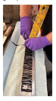
14) Ensure adhesive is visible at all joint edges, filling the bolt holes and all gaps. Remove some of the excess adhesive from each end using a plastic scraper. Leave some adhesive behind to bond and seal the end plates. Remove excess adhesive and masking tape from the bolt holes.
