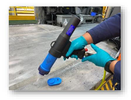
12) Apply TEROSON MS 9320 SF into the sill plate's central channel, ensuring sufficient product is applied to completely fill all voids and allow for any excess to flow up the sides and out of either end, providing a complete witness around the Treadmaster covering strip. Try to avoid large gaps in the adhesive pattern which could trap air beneath the covering.
