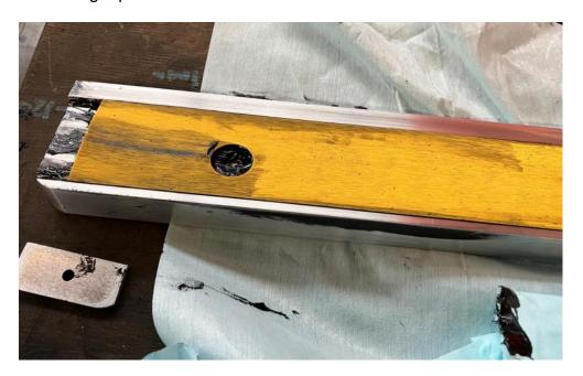
15) Place the prepared end/retaining caps on top of the remaining excess adhesive and slide these into place against the end of the covering strip, ensuring the adhesive squeezes out between the covering and aluminium plate and forms a visible witness. Fit and torque bolts as per TfL specification.
