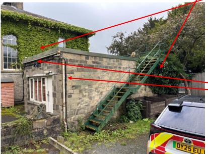
Remove the redundant cast iron protect the armoured power cables running above the windows and behind the downpipe.
