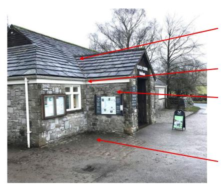
Carefully remove and set aside cut valley slates for re-use on the relocated porch roof.
