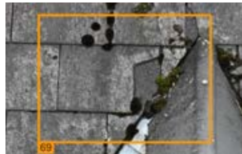
# 69 Damaged slate
