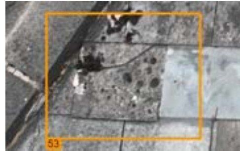
# 53 Damaged slate
