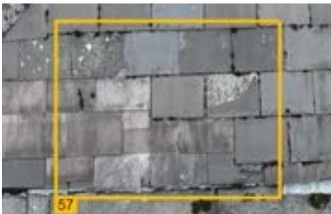
# 57 Damaged slate
