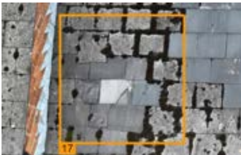
# 17 Damaged slate
