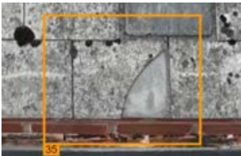
# 35 Damaged slate
