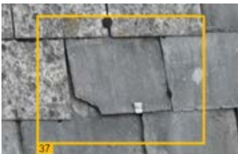
# 37 Damaged slate
