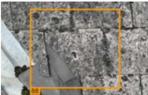
# 88 Damaged slate
