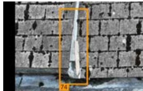
# 74 Missing mortar to verge
