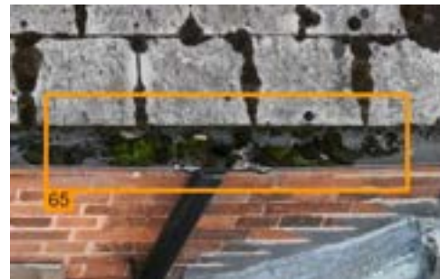
# 65 Blocked gutter/outlet
