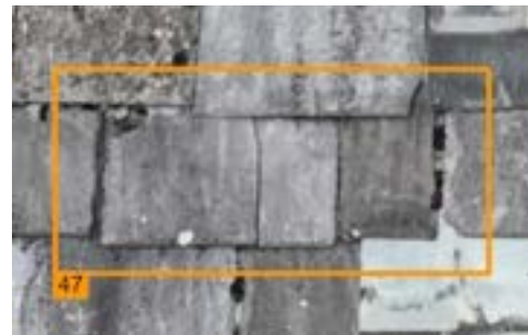
# 47 Damaged slate
