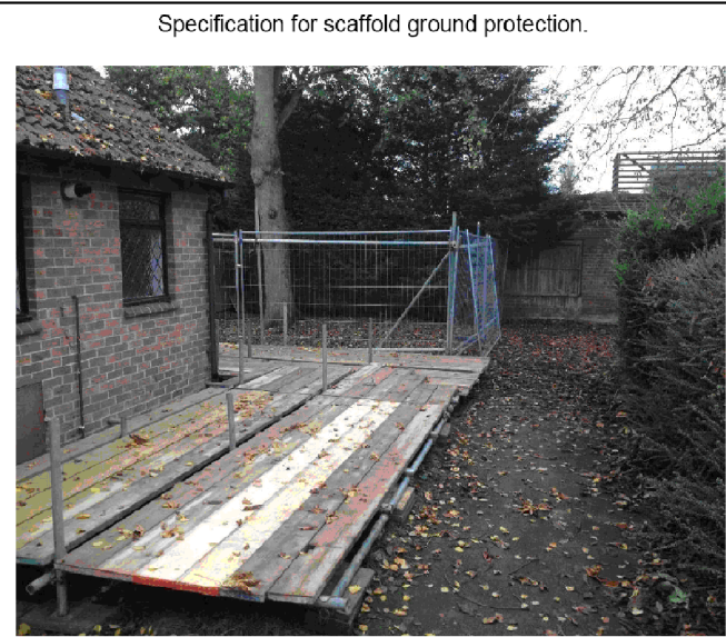
a) Stabilizer strut with base plate secured with ground pins
