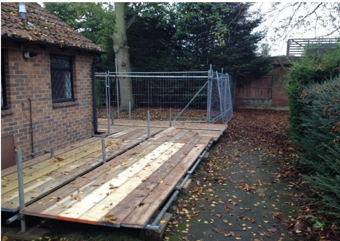
Figure 7 – Specification for scaffold ground protection.
