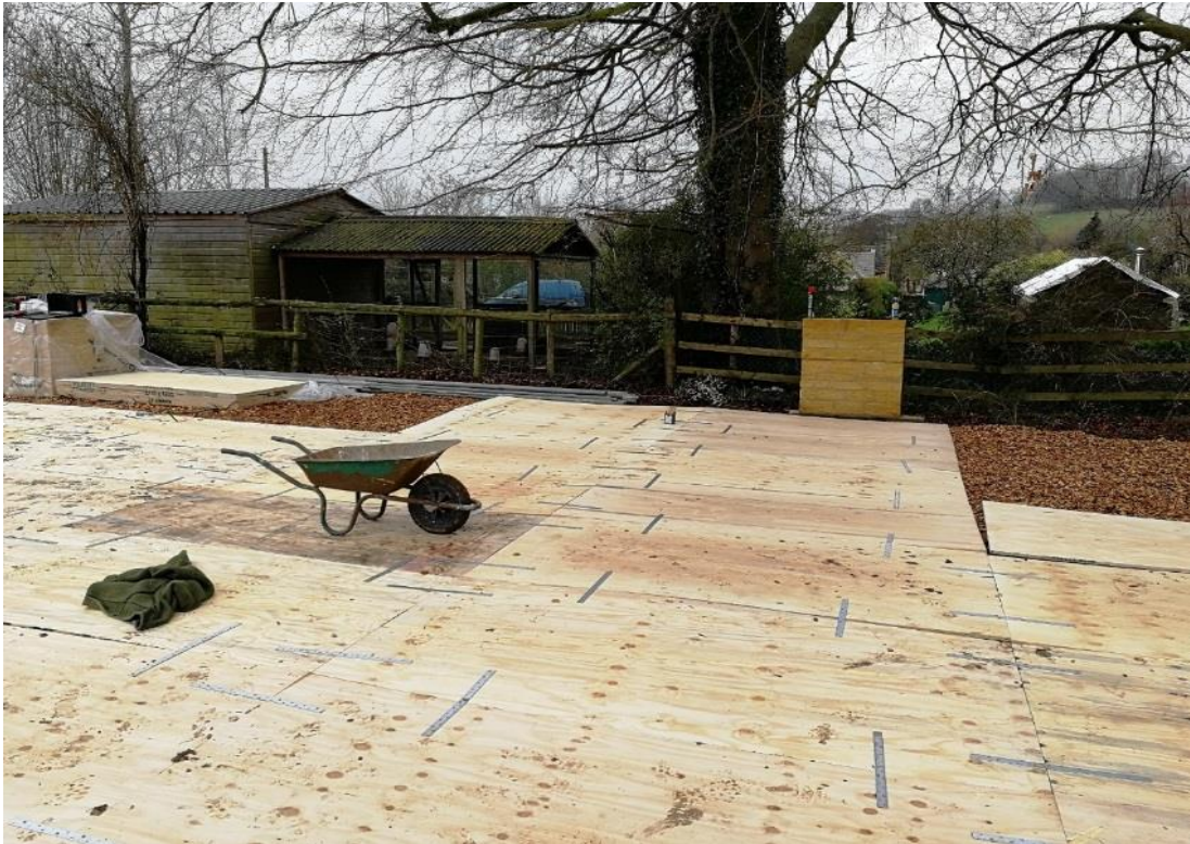
Figure 6 – Plywood sheeting used as ground protection.
