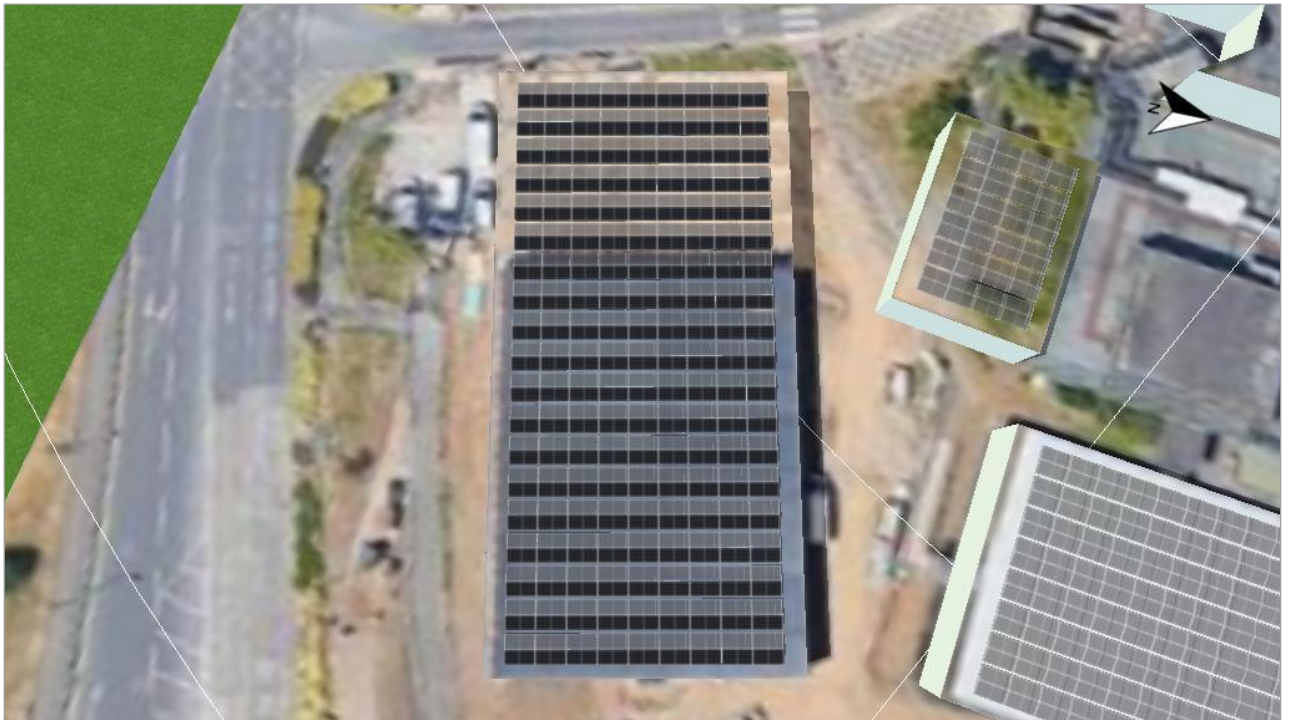
Figure: 7. Module Area - Building 01-Module Area East
