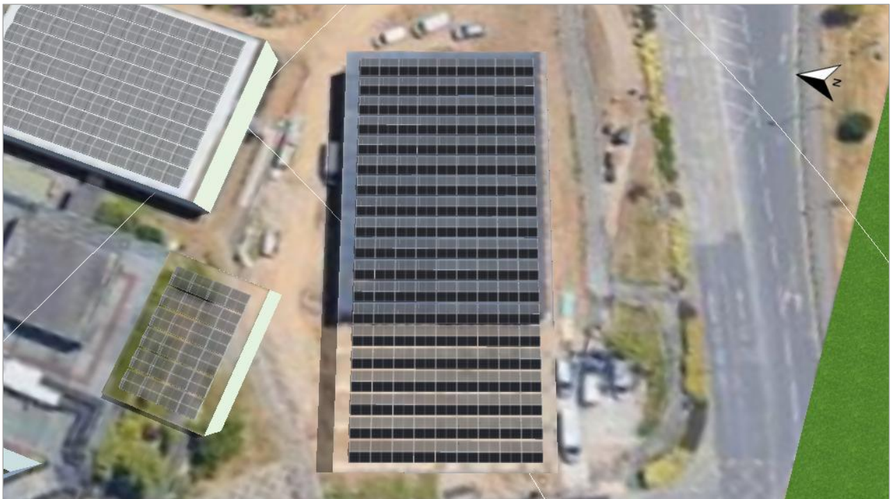
Figure: 8. Module Area - Building 01-Module Area West
