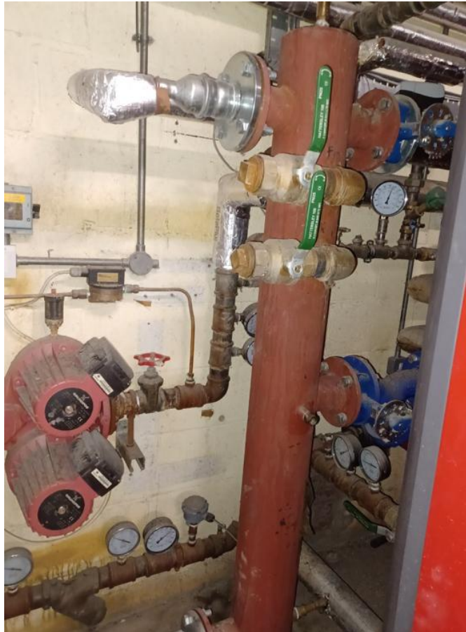
Figure 12: Pipe and valve insulation to be installed
