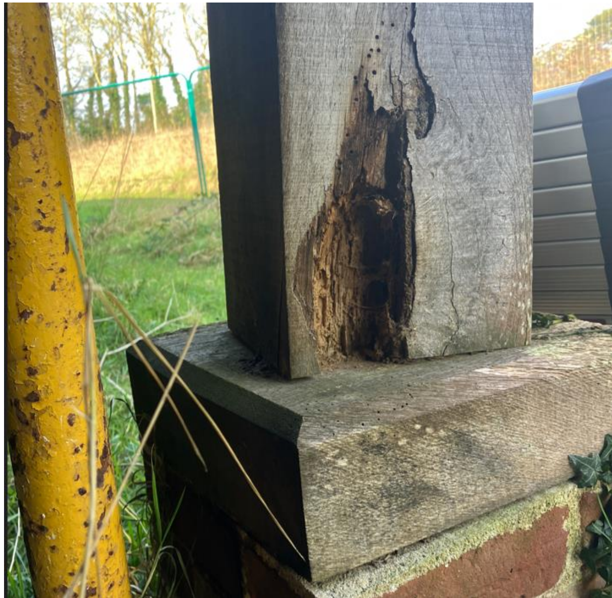
Photo 4 – Decay to base of post to Truss I
