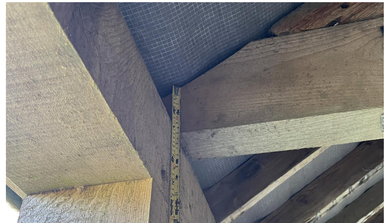
Photo 11 – Shallow end bearing to truss end
