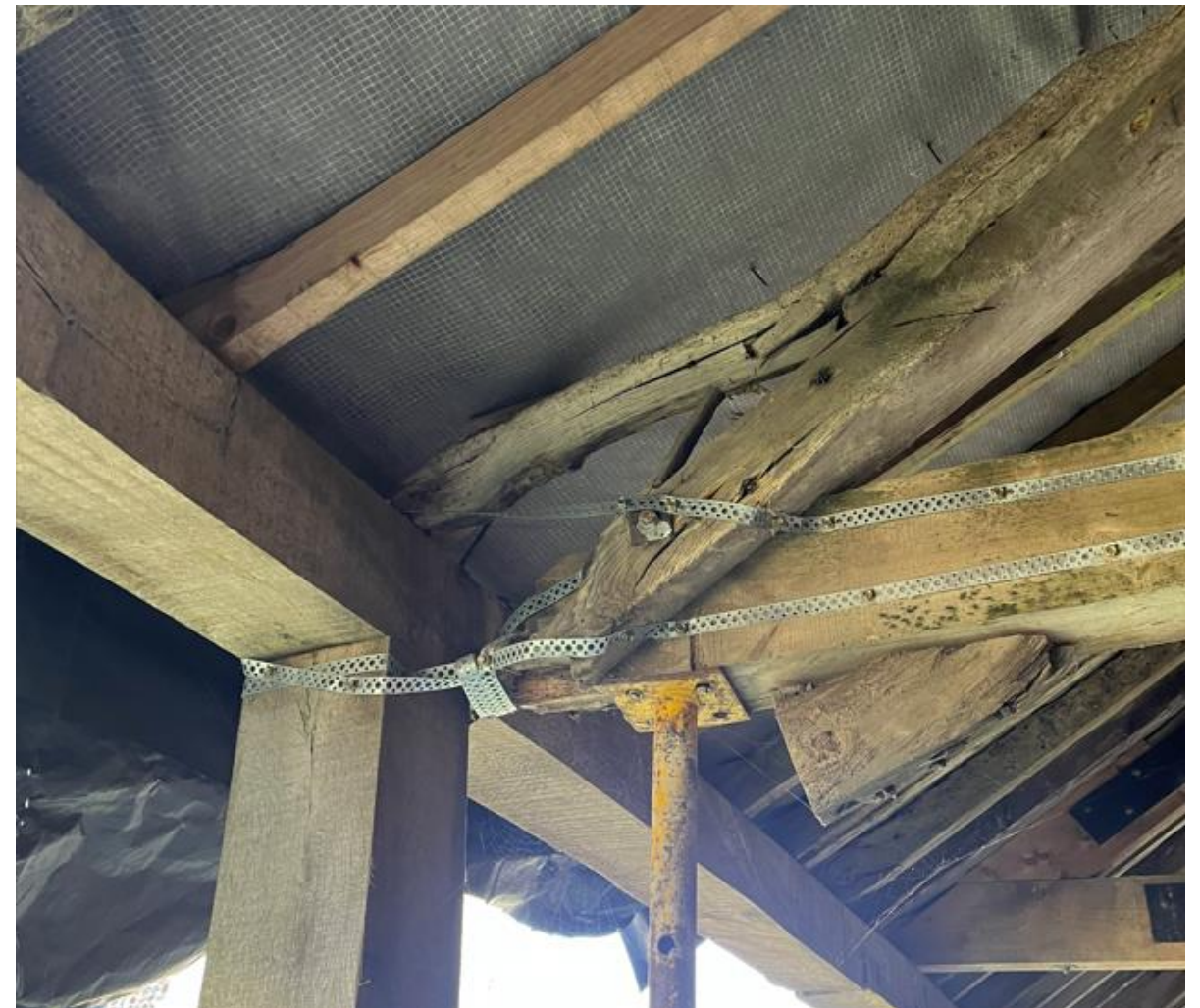
Photo 3 – Failed end of Truss I
