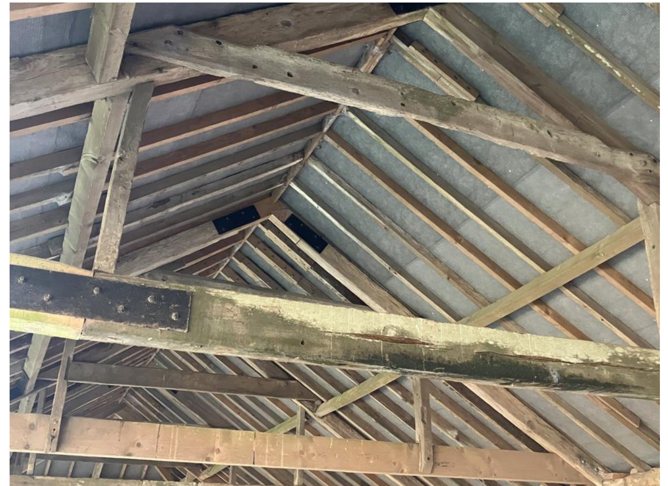
Photo 7 – Discolouration and potential decay to lower chord
