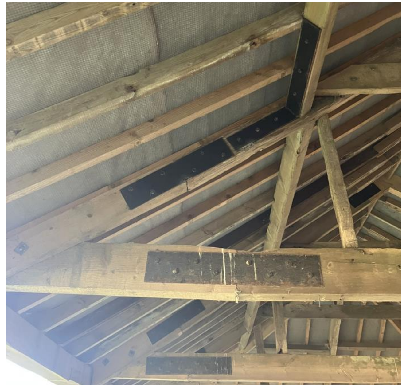
Photo 5 – Steel splices to lower and upper chords to eaves, with strengthening strap to purlin
