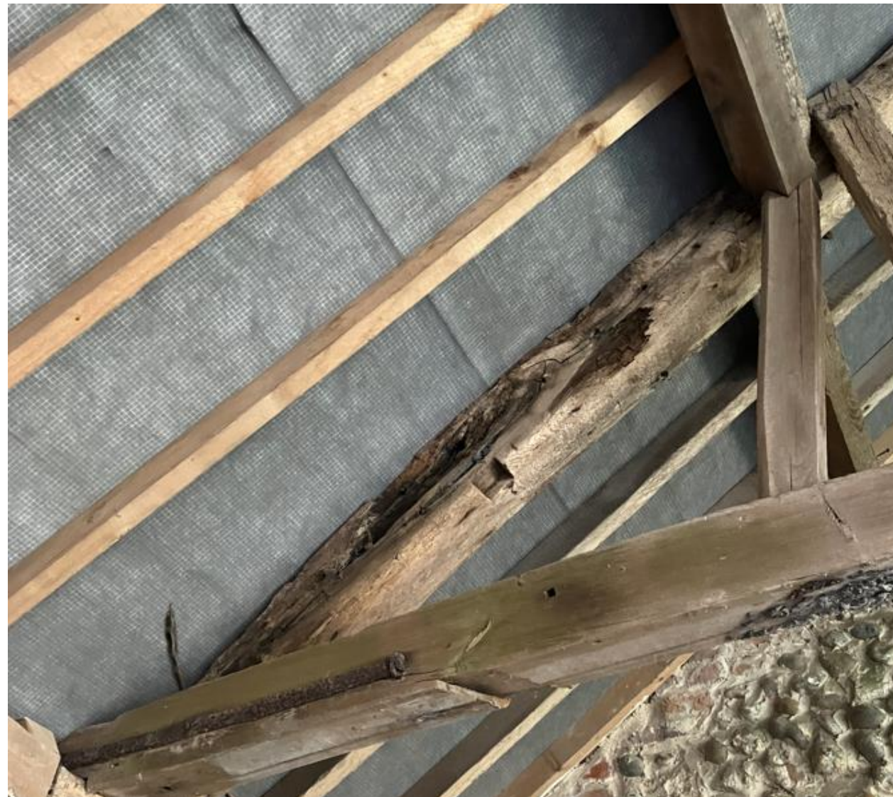
Photo 8 – Suspected decay to Truss J upper chord
