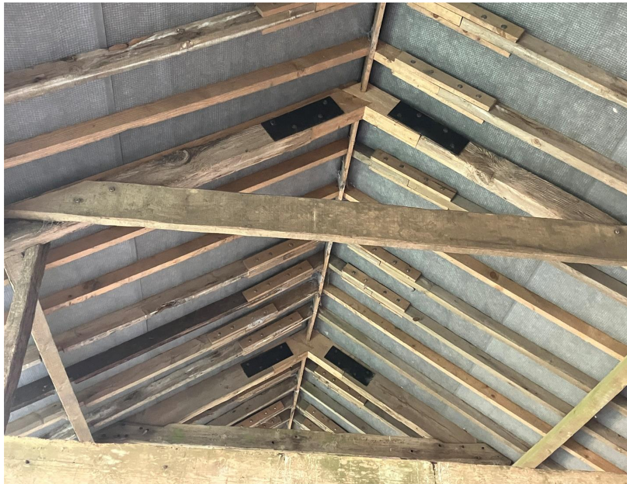
Photo 6 – Spliced ends at the ridge; in steel to the upper chords, and timber to the rafters
