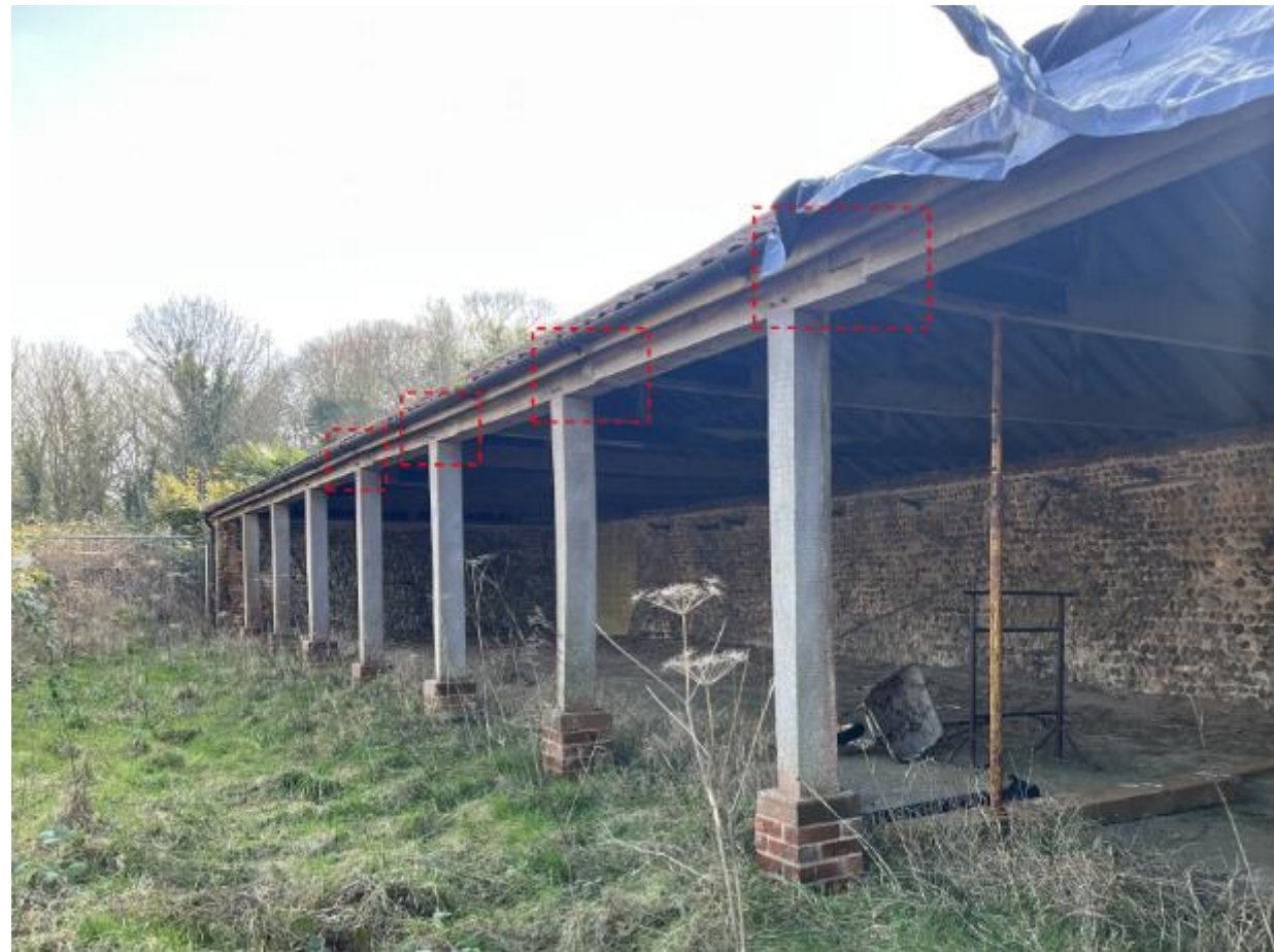
Photo 2 – overall view of the open front elevation framing, with displaced bressummer connections highlighted
