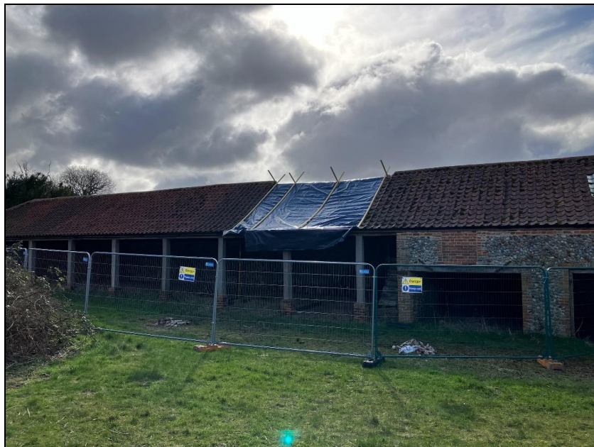
Figure 4: Temporary stabilisation and roof covering, and exclusion of public footpath from the South Range (Photo: Natural England/ Howard Jones).
