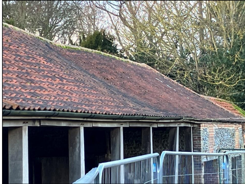
Figure 3: The South Range, looking West, showing subsidence to roof (Photo: ©Natural England/ Howard Jones).
