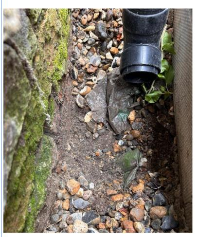
Remove all gravel to channel to allow for downpipe. See RAINWATER GOODS AND DRAINAGE FOR RECOMMENDATIONS
