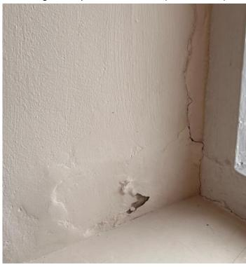
In tandem with the window overhaul and external wall works, the affected plaster should be removed internally, allowed to dry out. Once dry, lime plaster should be used to repair.
