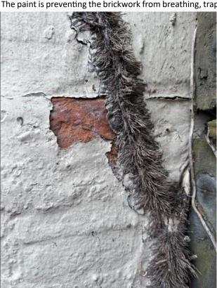
Remove paint covering and paint with fully breathable paint system. Some lime repointing of joints may be required when paint is removed.
