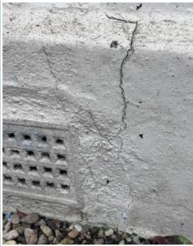
Vertical cracks throughout the plinth. Failed paint coating. Tapping slightly hollow to LHS to indicate background damp behind. Paint system flaking and bubbling throughout.
