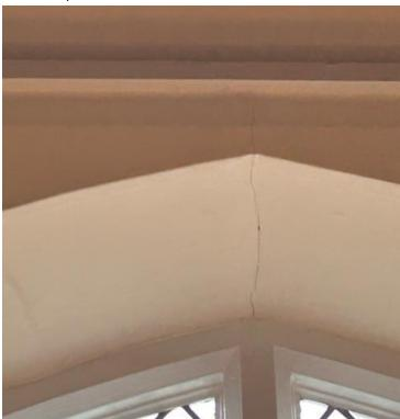
window is overhauled, the internal cracks can be raked out and made good.
