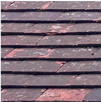
Monitor and replace significantly damaged tiles as part of routine maintenance. Likely from year 3-5
