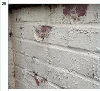
Bubbling paint and raised mortar joints. More advanced below sill and to black painted plinth. The type of brick is more resistant to moisture—as such the actions are not urgent.
