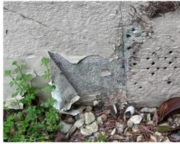
Remove paint covering and paint with fully breathable paint system. Some lime repointing of joints may be required when paint is removed.
