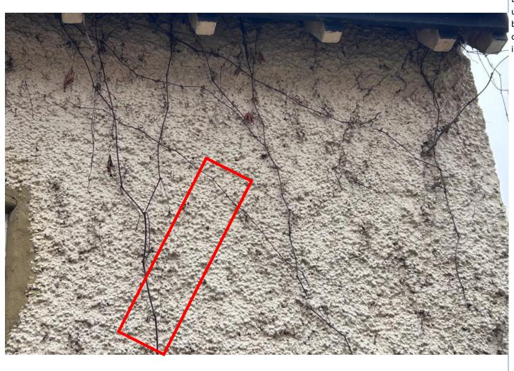
Render to be removed. Lime render should be used in replacement, to be fully designed out once the face of the wall is exposed.
