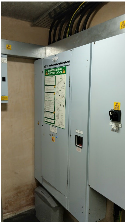
Photo 10 – Typical switchgear (main switch panel) for all halls – this photo is of Harting Hall
