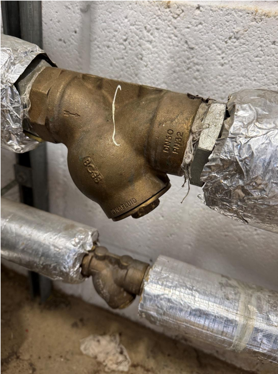
Photograph 9 – Y strainer – constantly getting blocked
