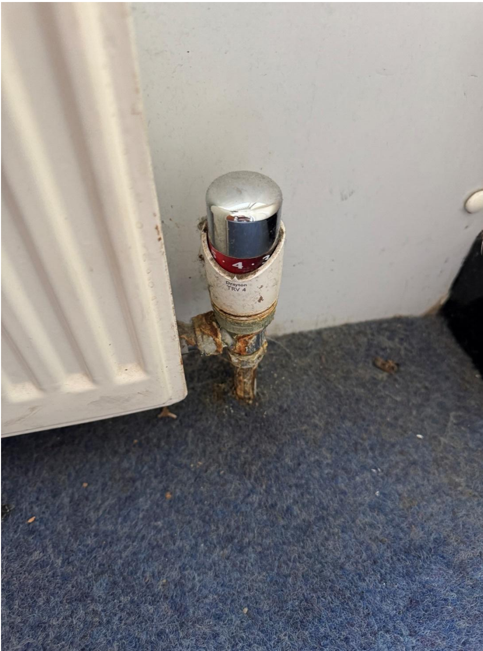
Photograph 11 – TRVS showing signs of failure.
