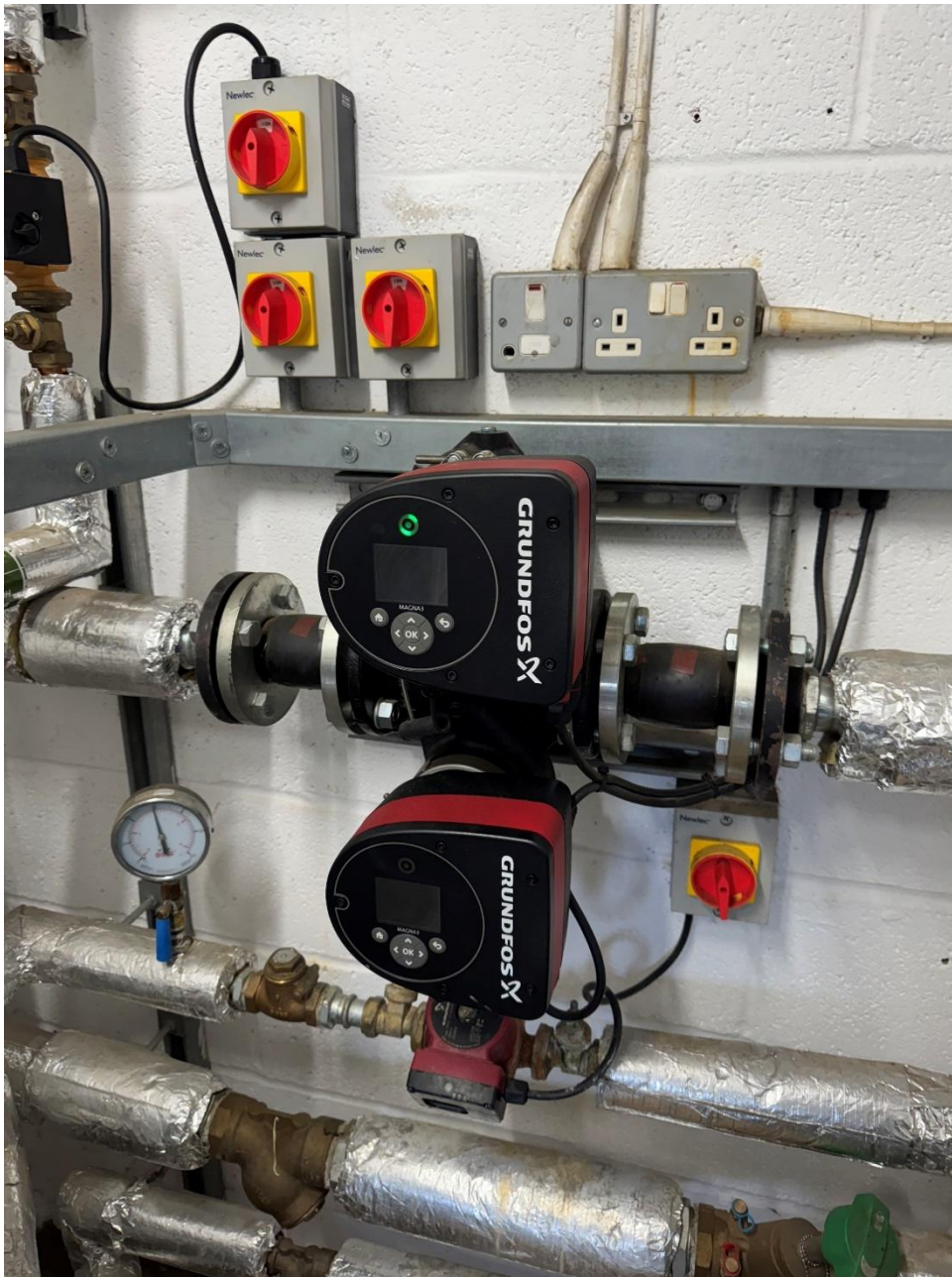
Photograph 8 – Secondary pumps
