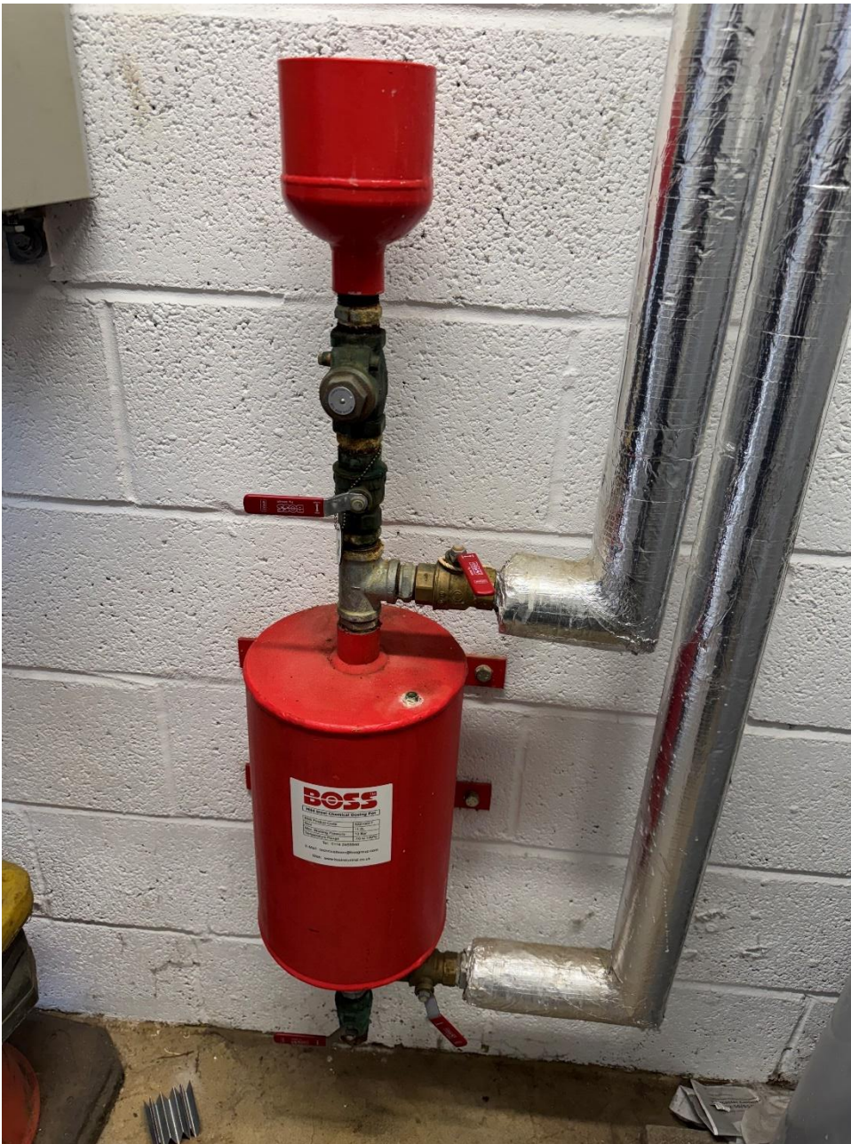
Photograph 7 – Existing dosing pot
