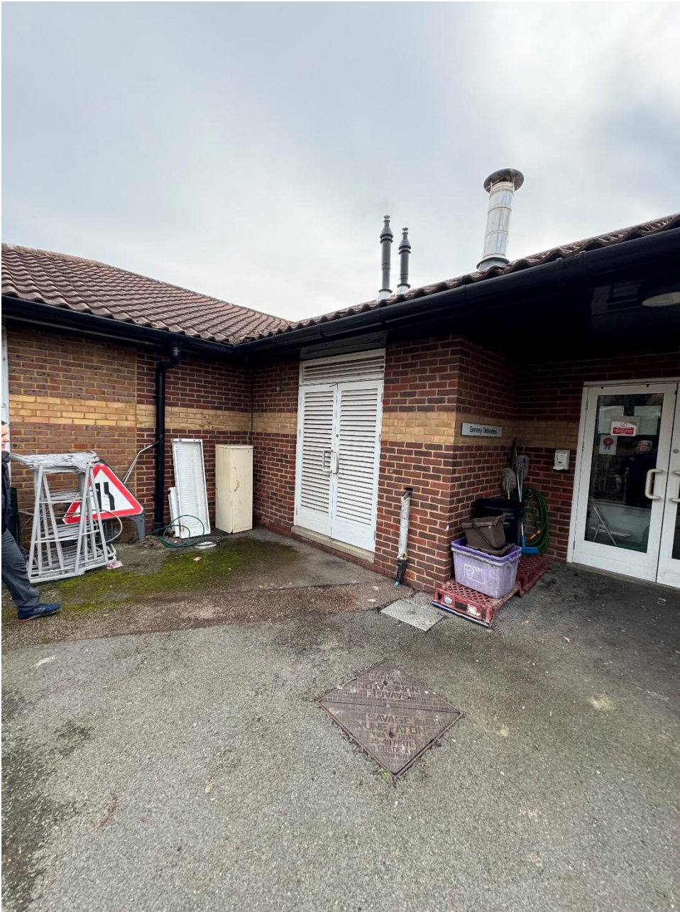
Photograph 1 – External of plant room
