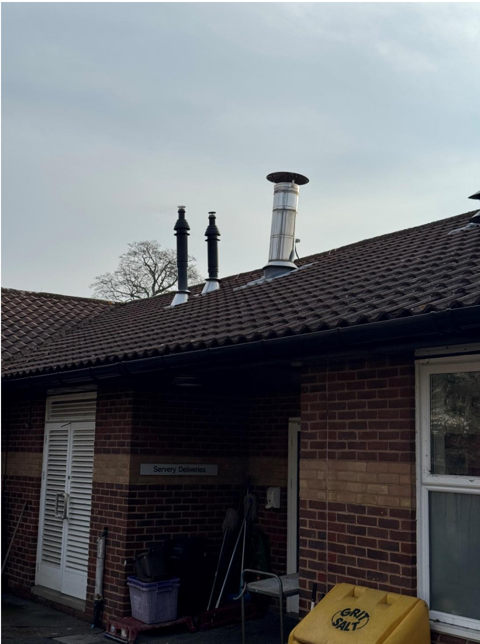
Photograph 14 - Boiler flue close-up
