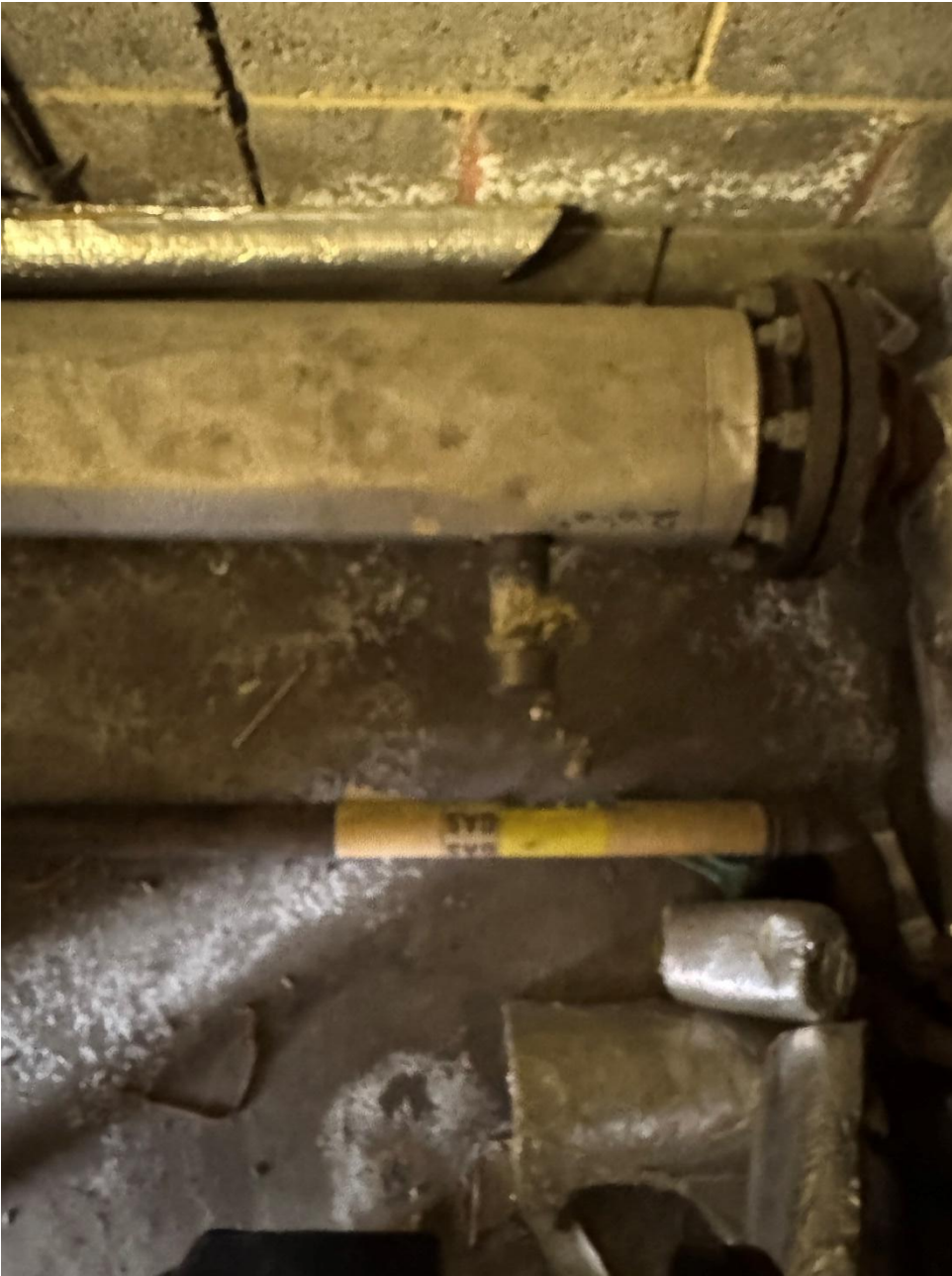
Photograph 9 - Primary supply cap
