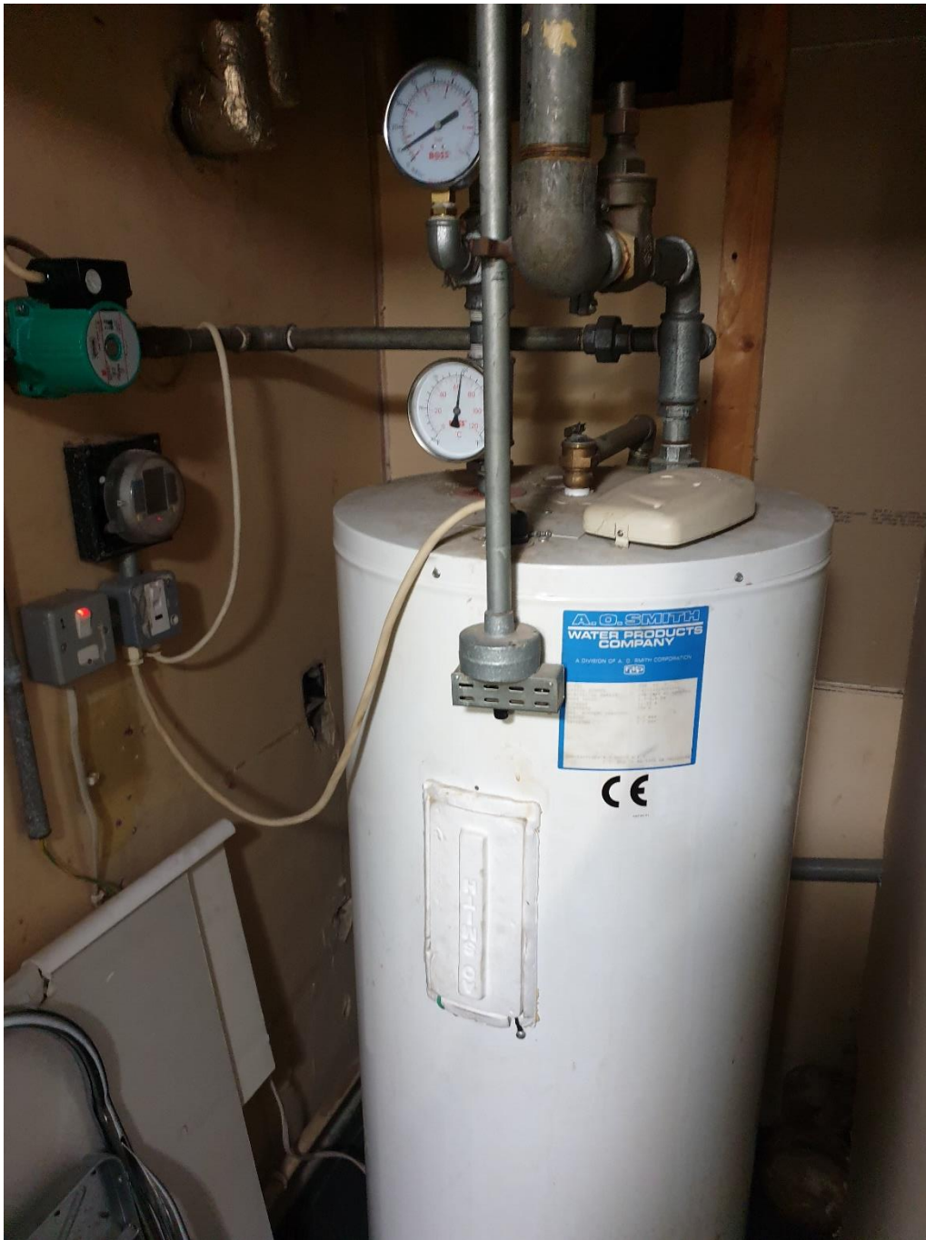
Photo 12: old HW cylinder and HW-R pump feeding right side of building
