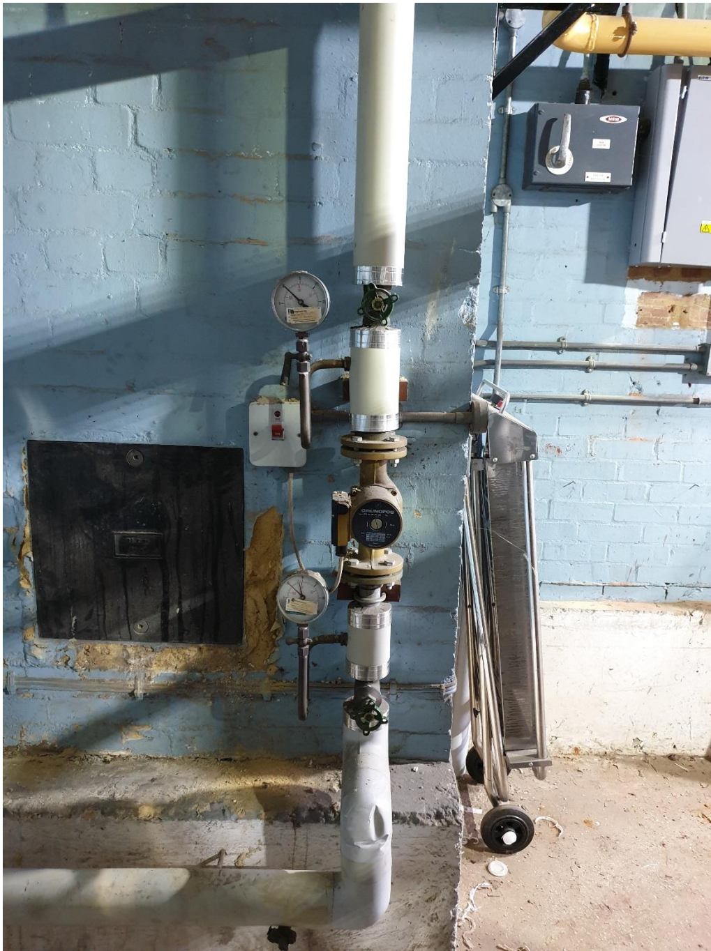
Photo 11: HW-R pump in plant room
