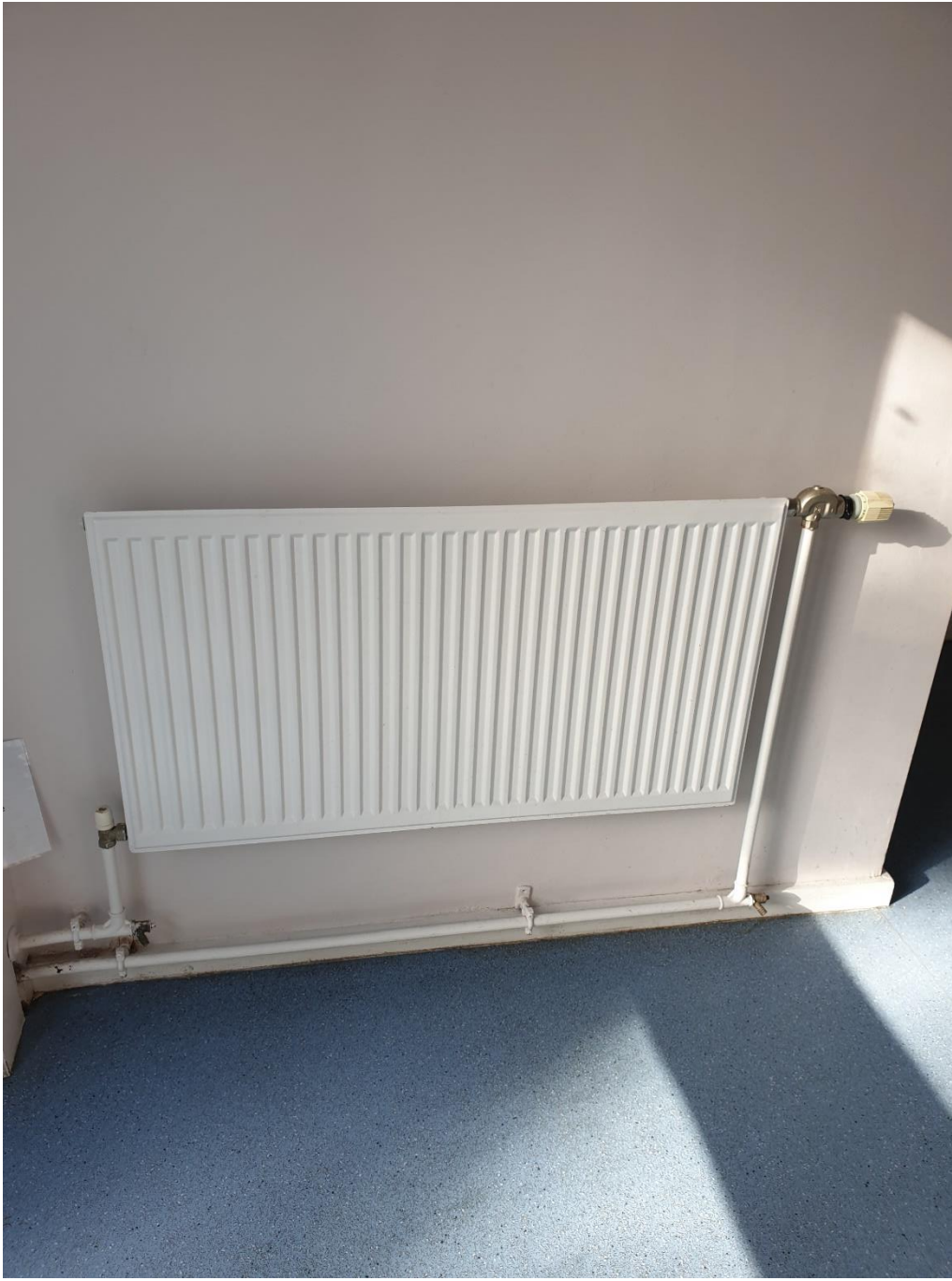
Photo 1: radiator connected to two pipe system
