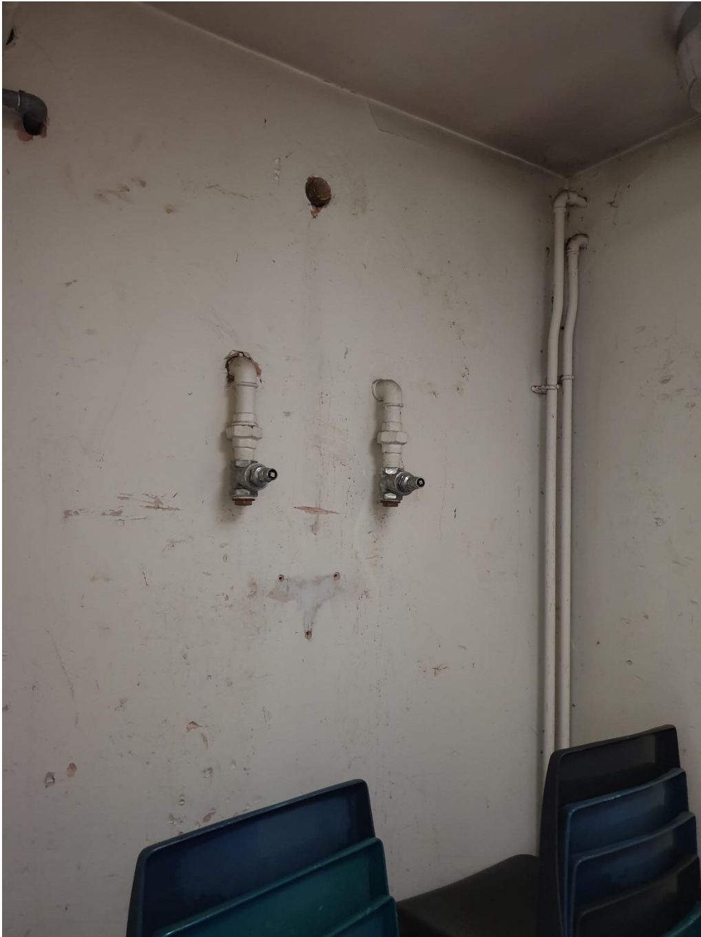
Photo 6: old shower block and domestic water dead legs
