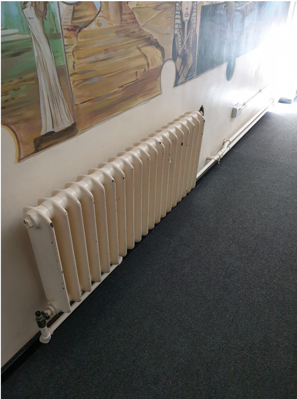
Photo 2: radiator connected to two-pipe system
