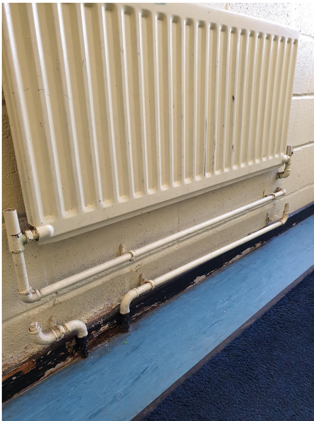
Photo 7: heating system dead legs
