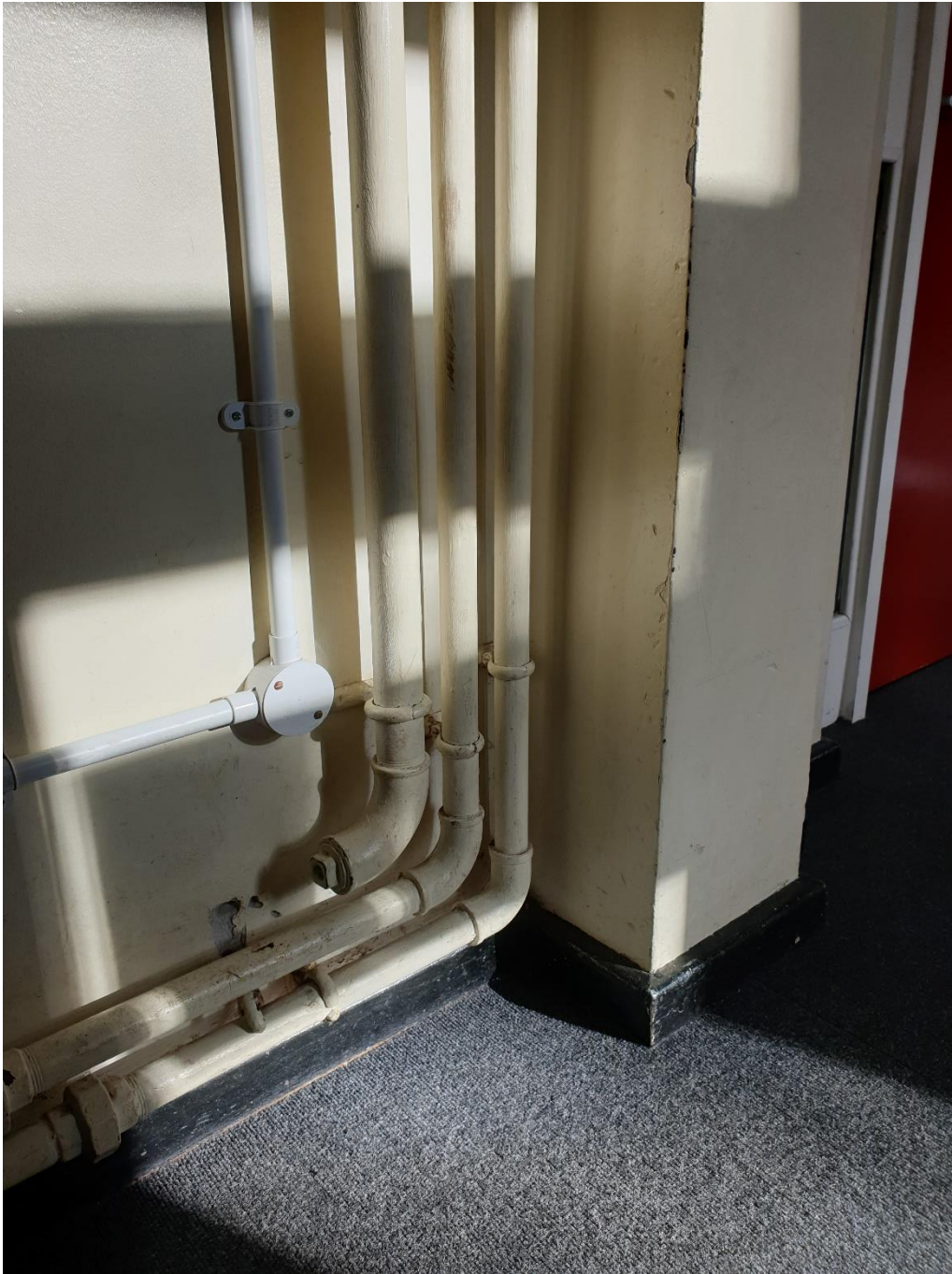
Photo 3: dead leg on heating system
