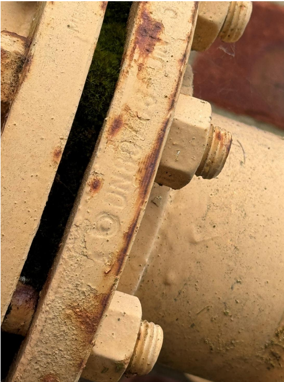
Photograph 35 – Gas supply pipe size of DN80.
