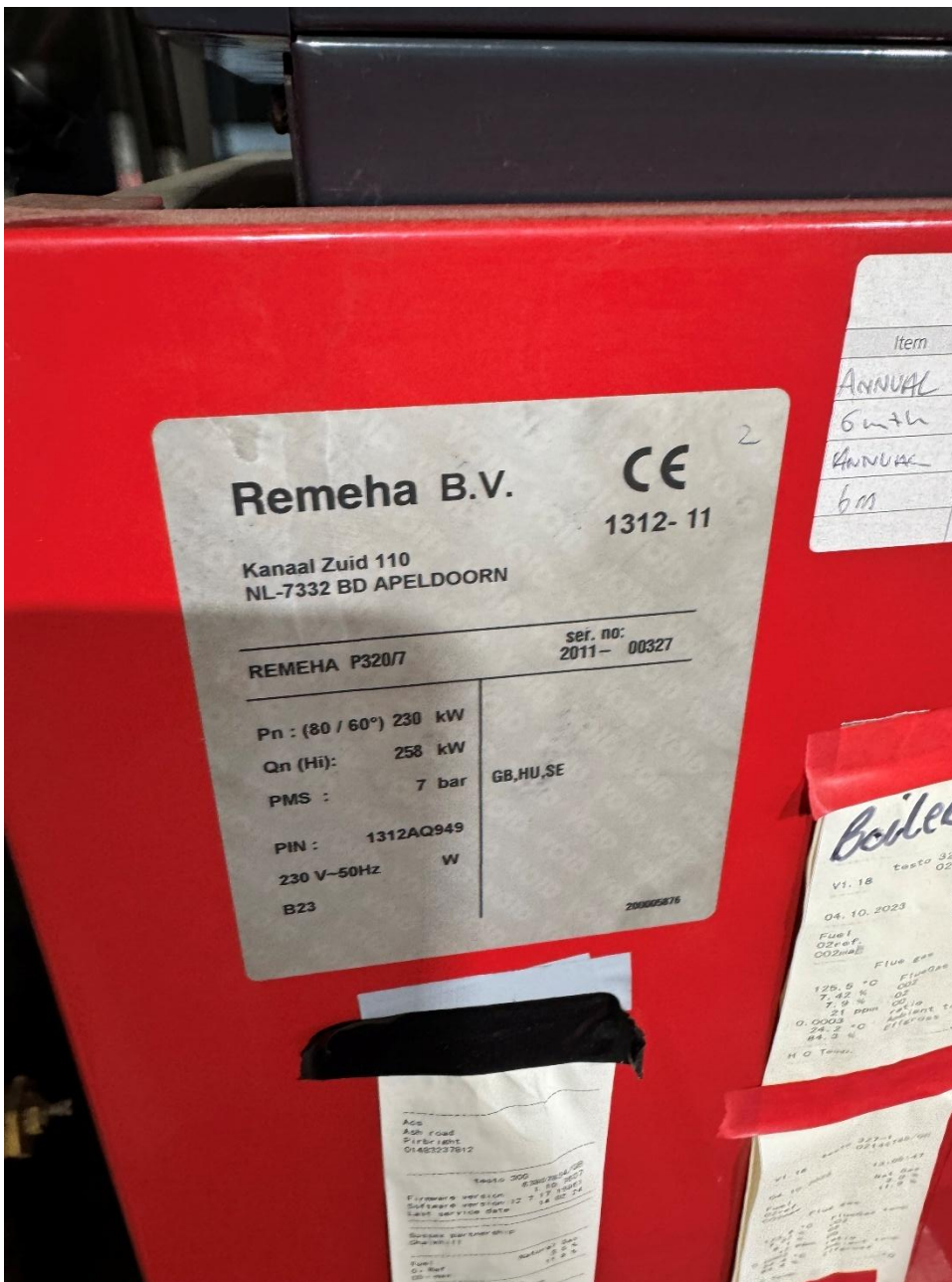
Photograph 22 – Boilers were noted as Remeha 1312- 230kW output.
