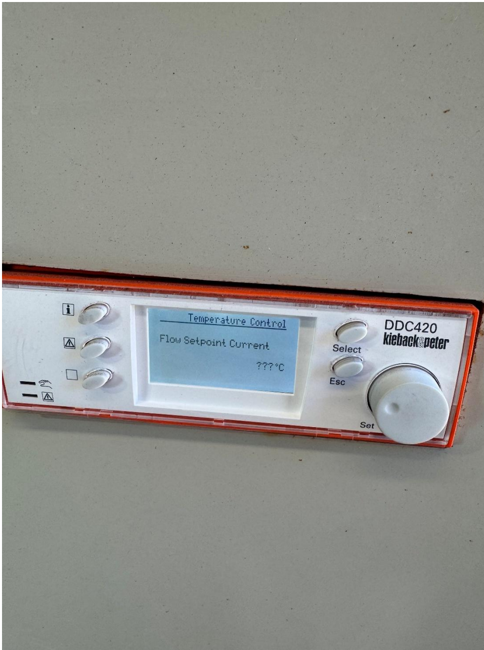
Photograph 21- Boiler controller seem to have limited control on the plant.
