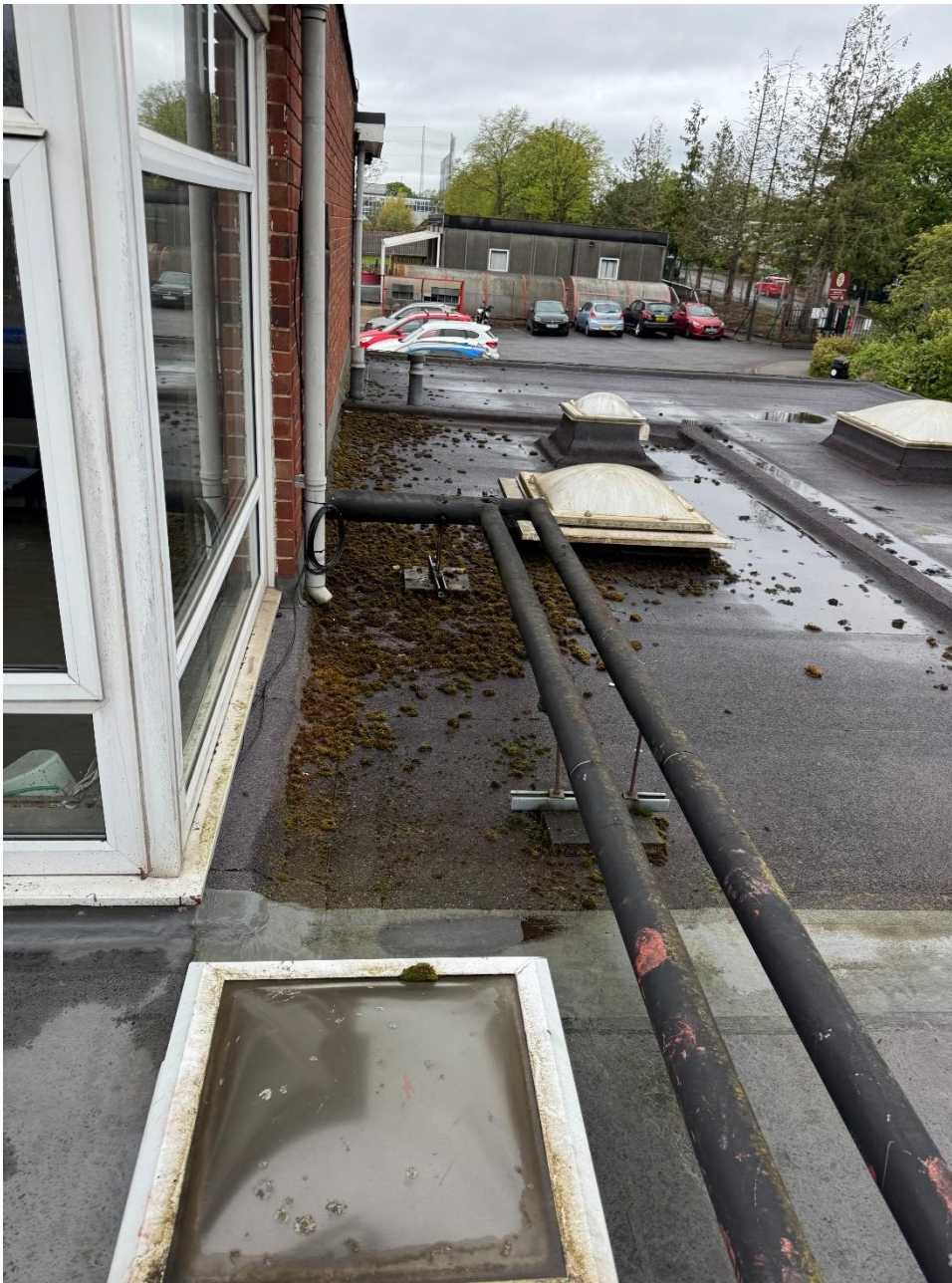
Photograph 34 – The insulation appeared to be in poor condition.
