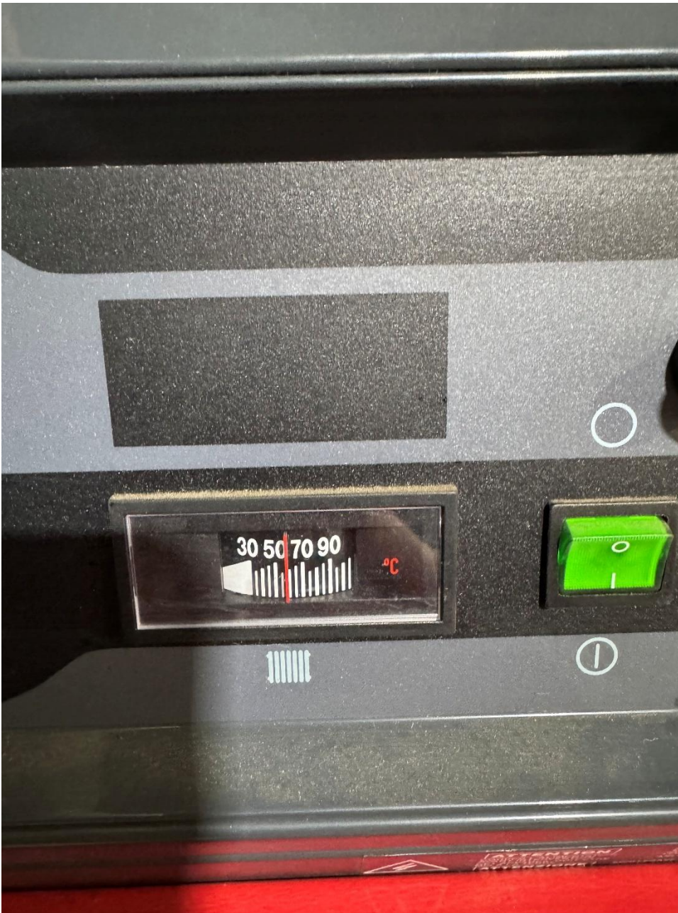
Photograph 5 - Boiler 1 flow temperature. Approximately 60°C
