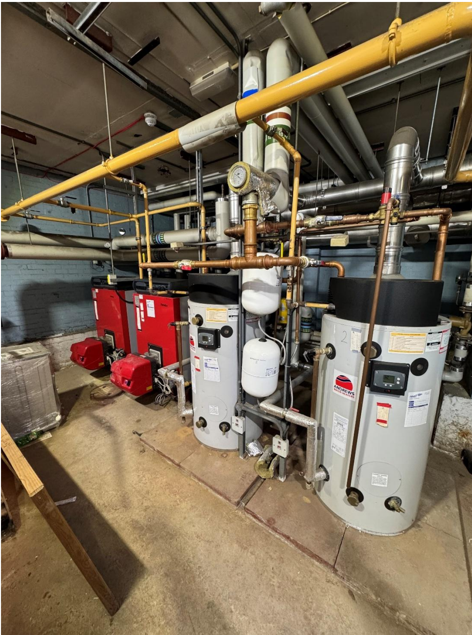
Photograph 2 - Installed plant – two boilers and two gas-fired water heaters.
