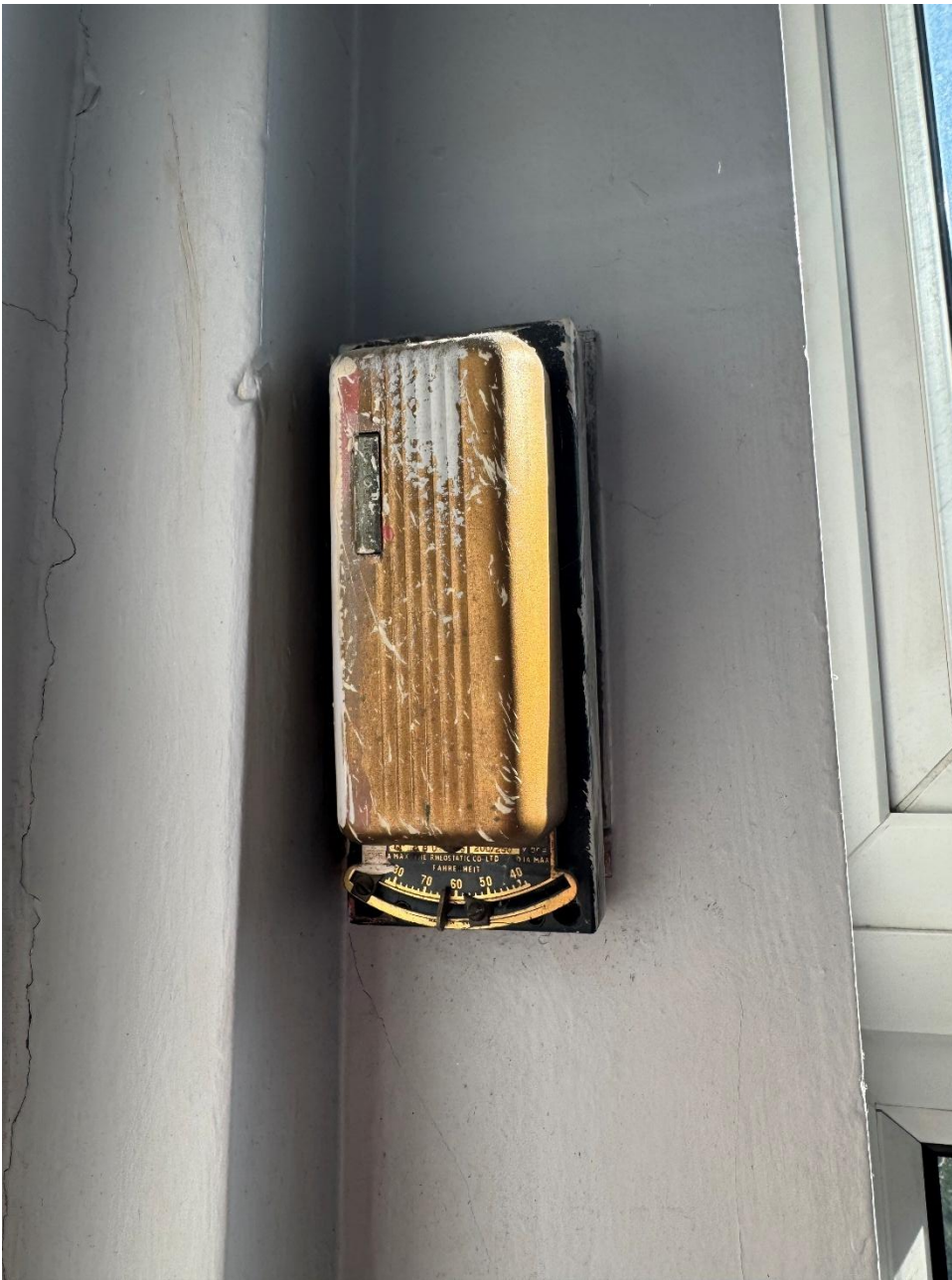
Photograph 26- Whitecode was shown, which the school believes is the heating control thermostat.
