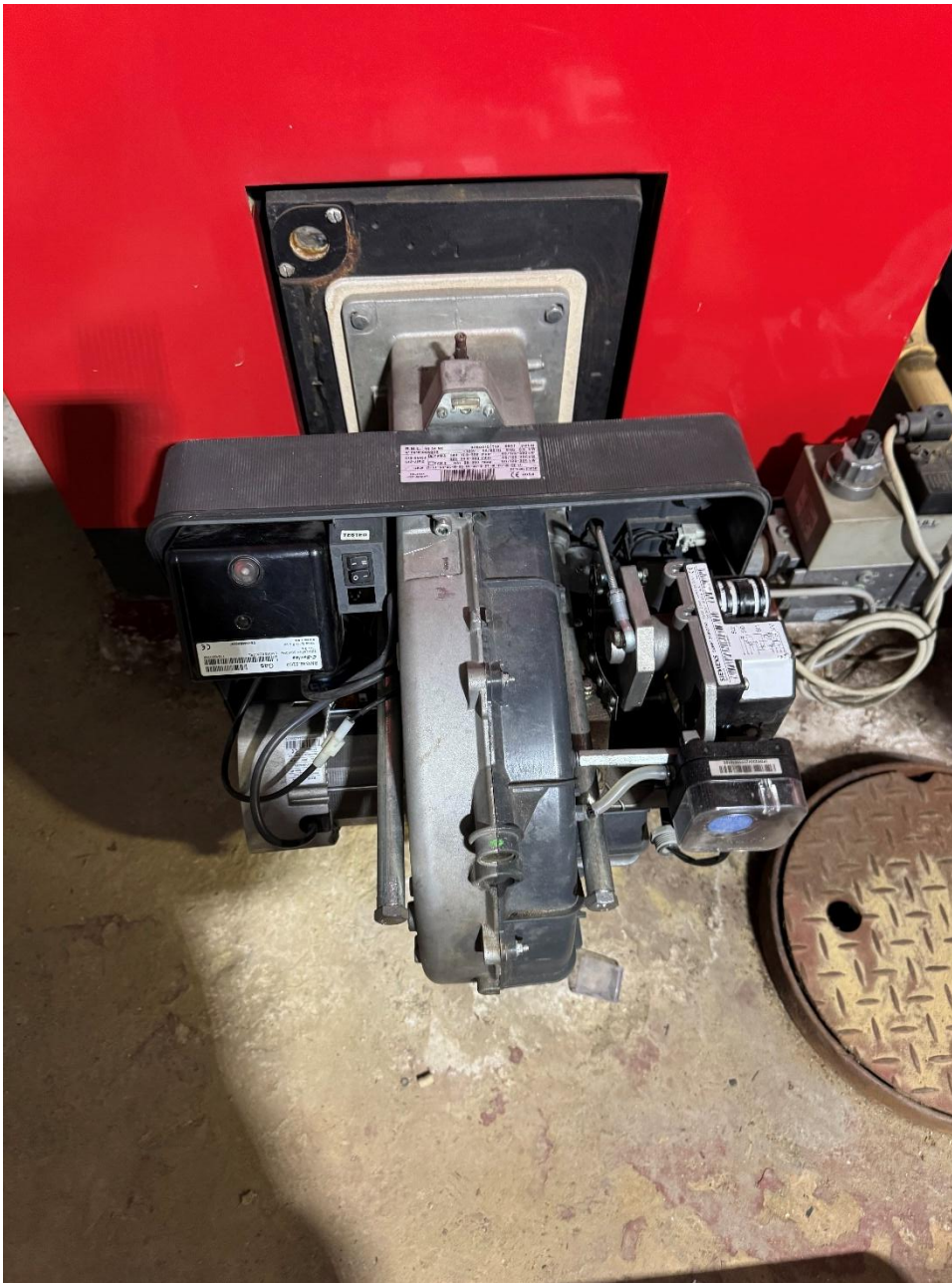
Photograph 19 - Burner 1 was set to a 2-stage fire, providing maximum output.
