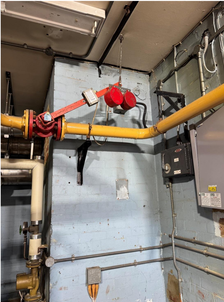
Photograph 4- Gravity gas shut-off valve. No obsolete and should be replaced.
