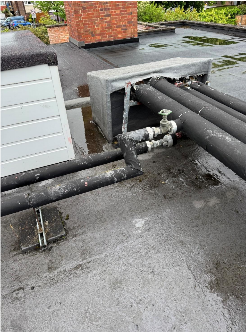
Photograph 33 - Insulated valves feeding the main hall.
