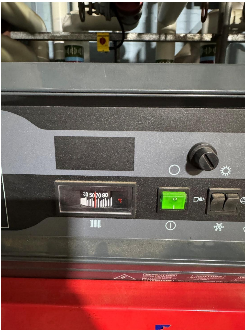
Photograph 17- Boiler flow temperature was seen to increase.
