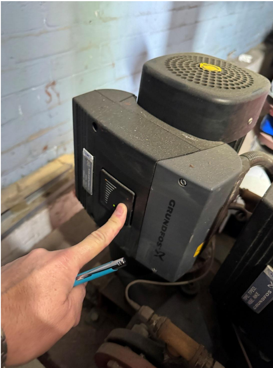
Photograph 12 - Whitecode increased the pup speed to max by holding the controller
