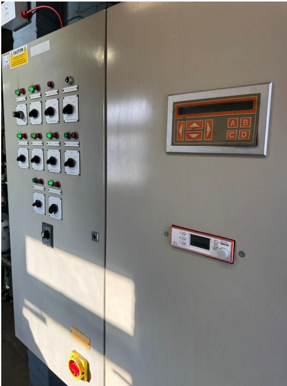
Photograph 1- The main control plant to the plant room with an obsolete Trend controller and a smaller retrofit controller.
