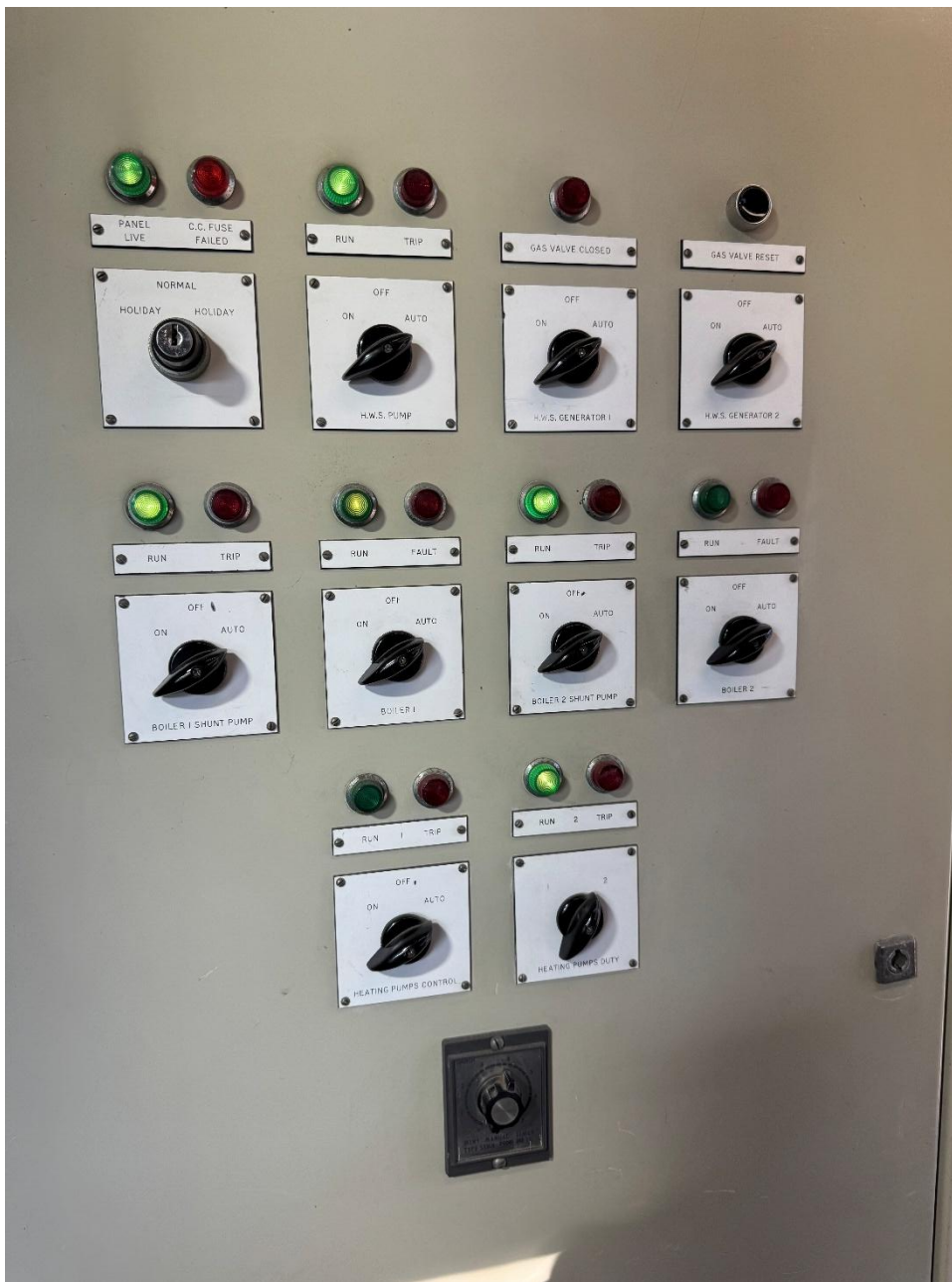
Photograph 15 - The BMS panel was noted as original to the plan room. It is beyond serviceable repair and should be replaced.
