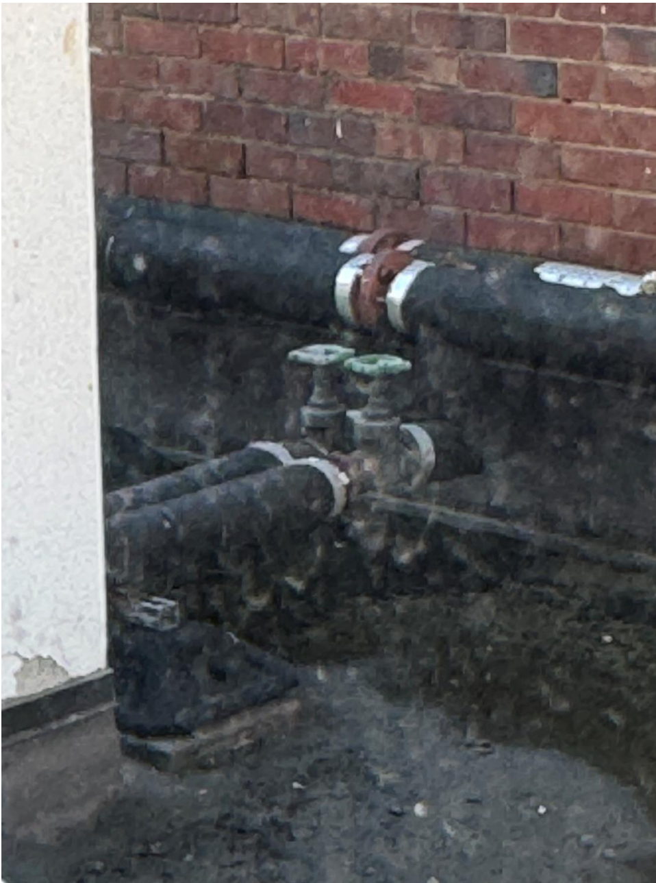
Photograph 28 - LTHW valves could be seen outside and were uninsulated.
