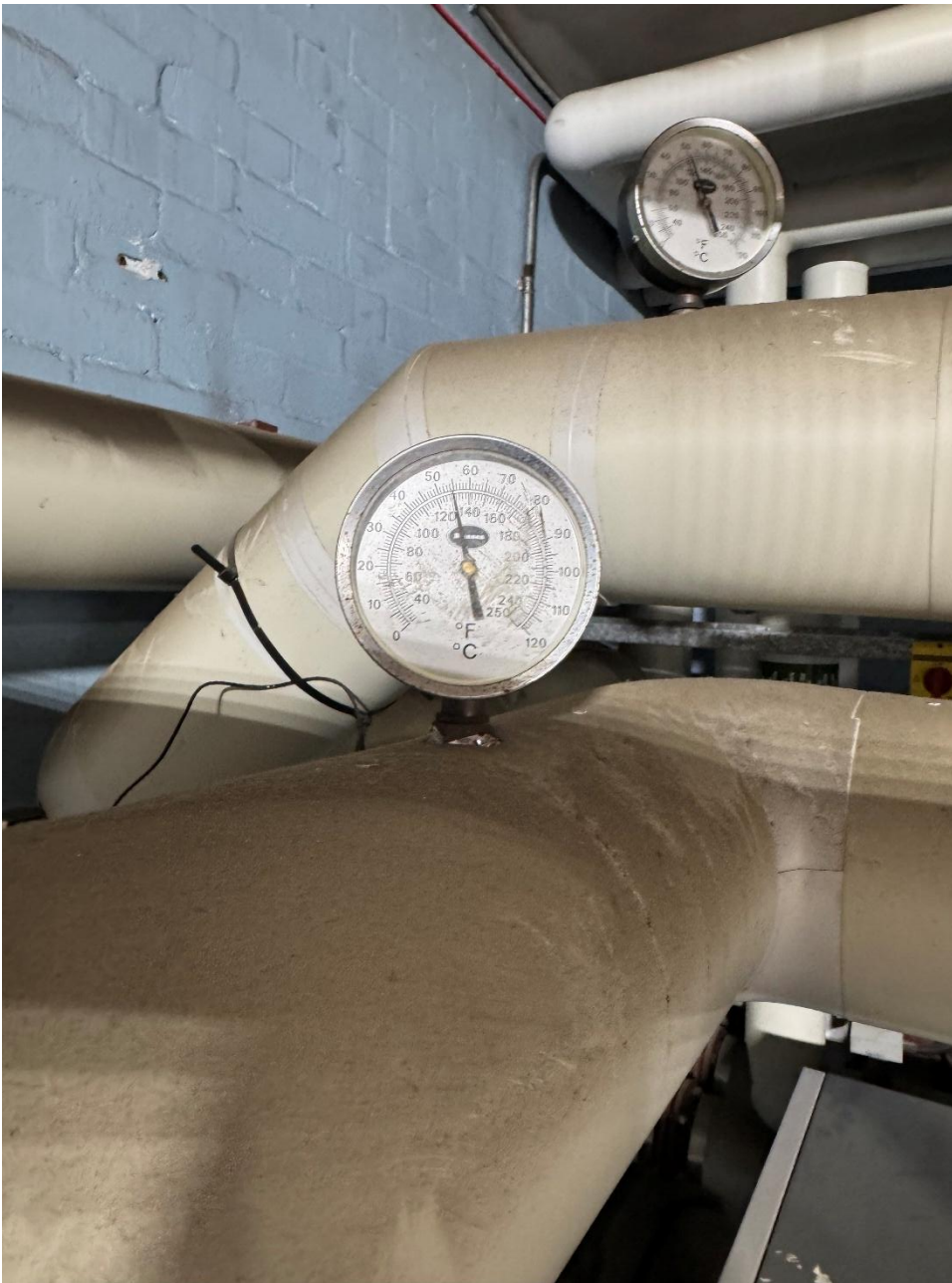
Photograph 7 – LTHW system flow temperature 55°C
