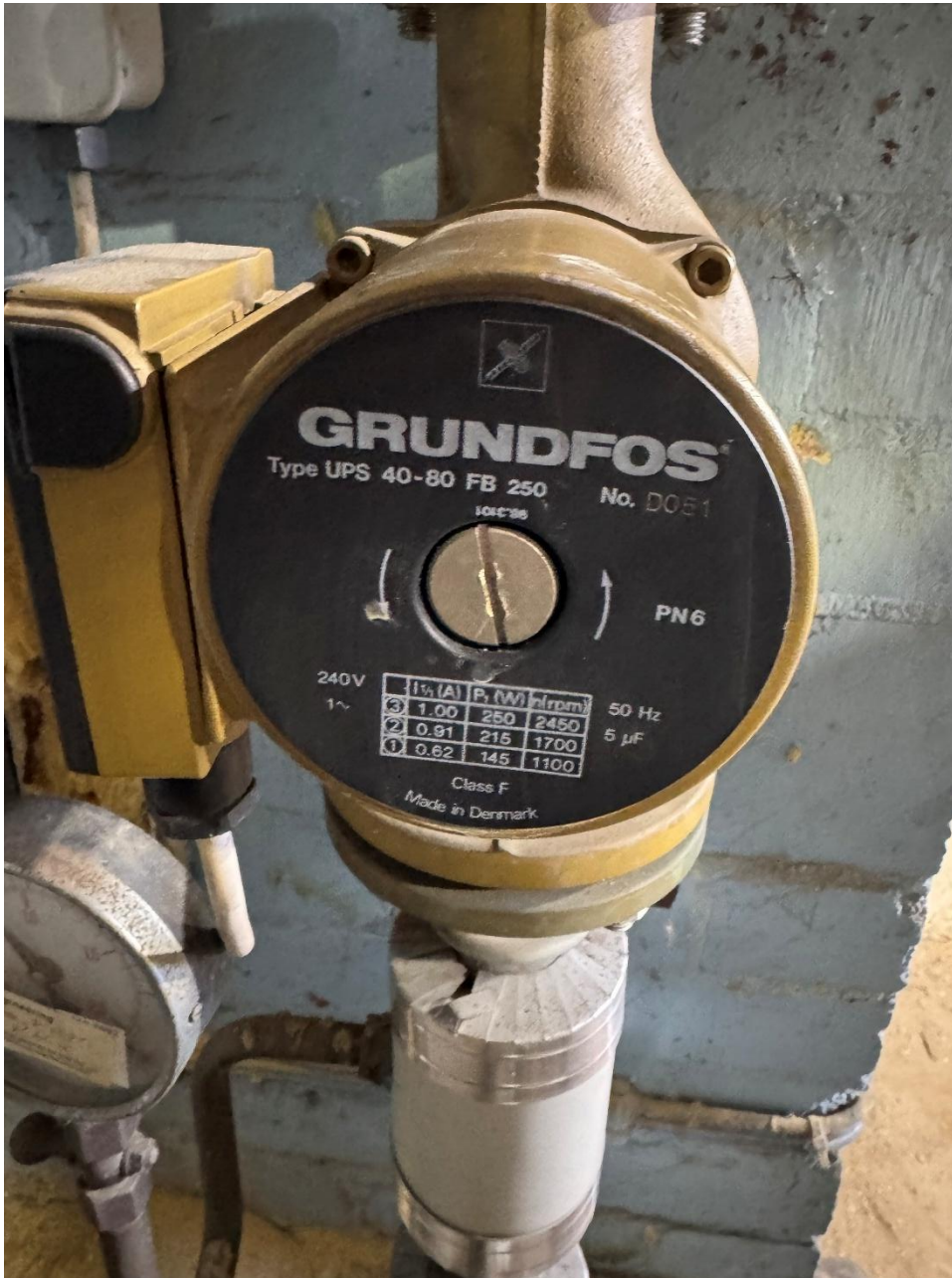
Photograph 31- Secondary return circulator was a UPS 40-80 in bronze.
