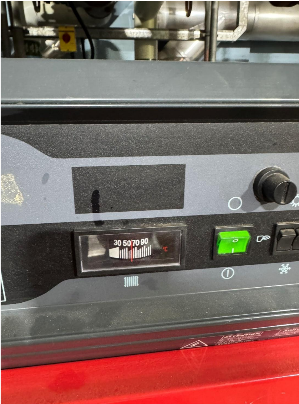
Photograph 6 - Boiler 2 flow temperature. Approximately 60°C
