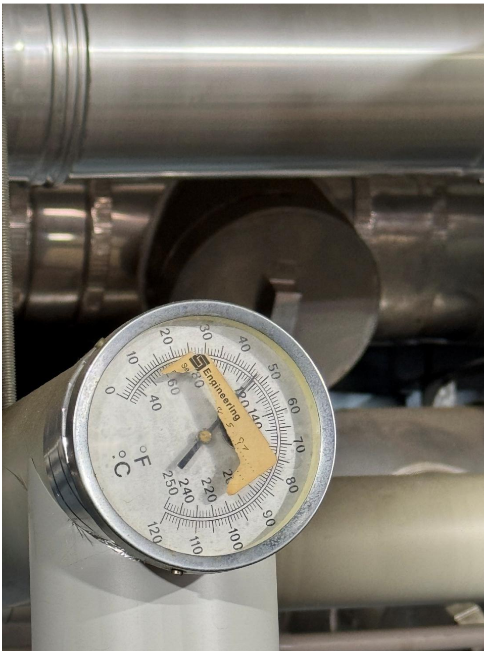
Photograph 30 - Hot water system retrain appeared to be lower the the L8 requirment of 50°C.
