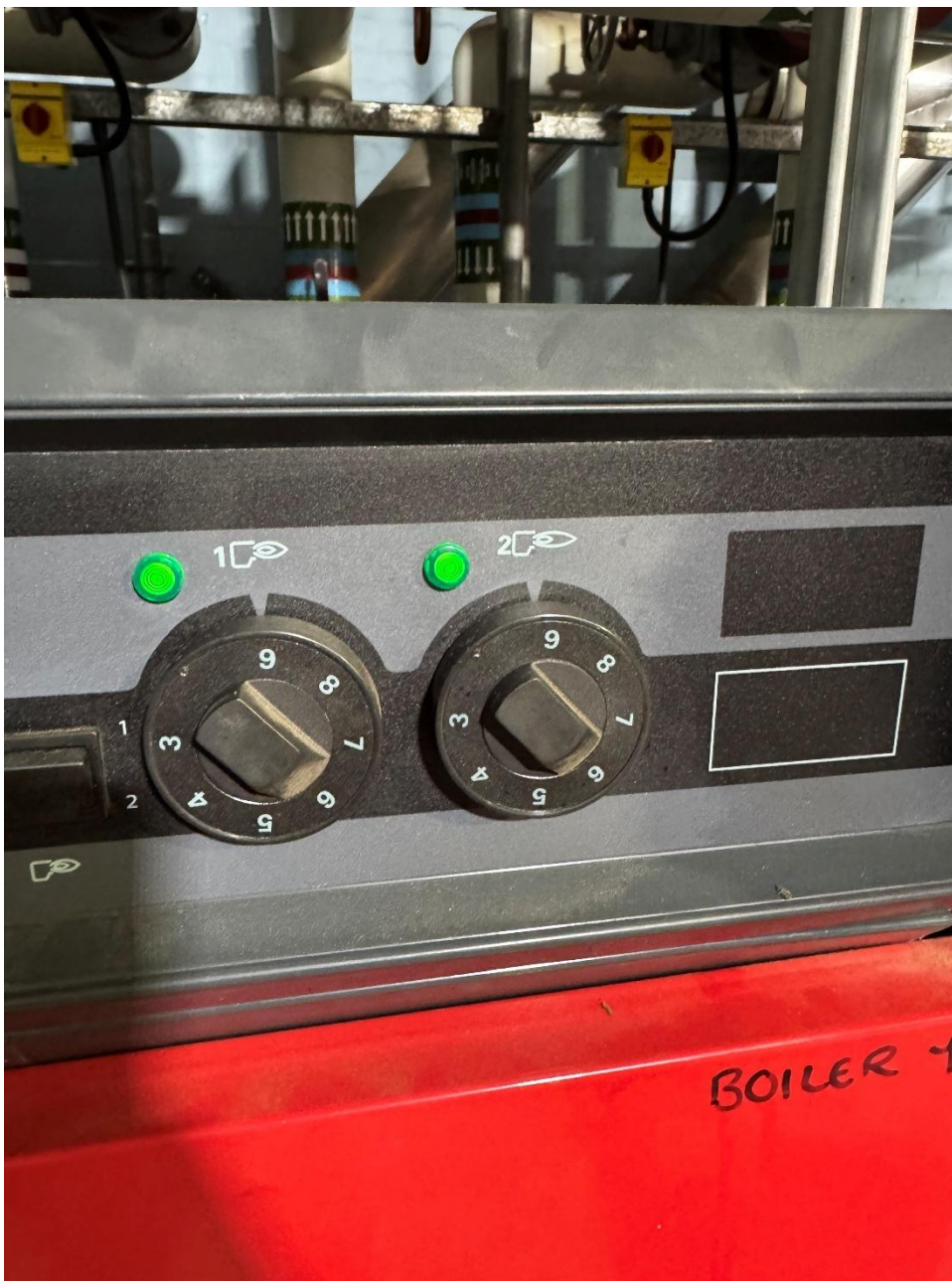
Photograph 16 - Whitecode increased the boilers' stats to 80°C
