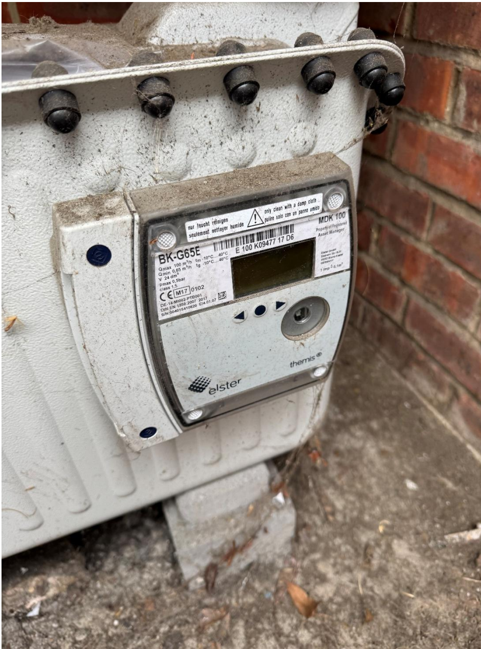
Photograph 37- Gas meter a G65.
