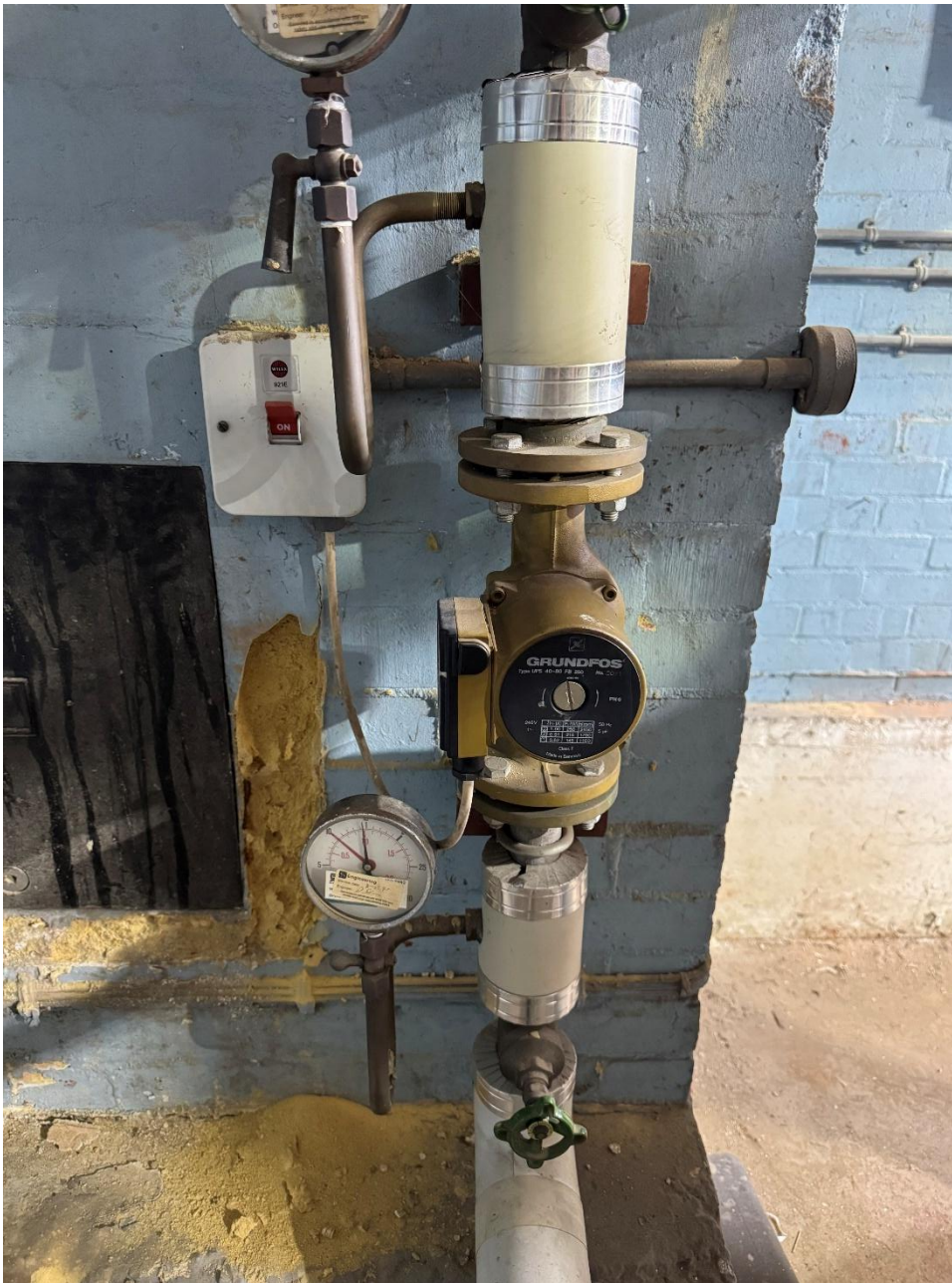
Photograph 3 – Bronze secondary return pump
