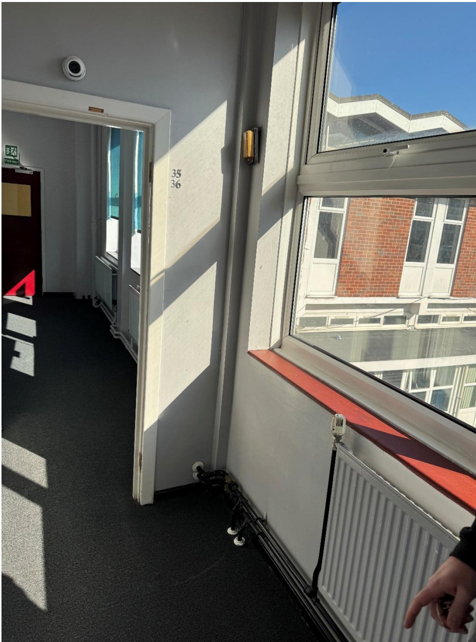
Photograph 27 - Thermostat location in sunny corridor.
