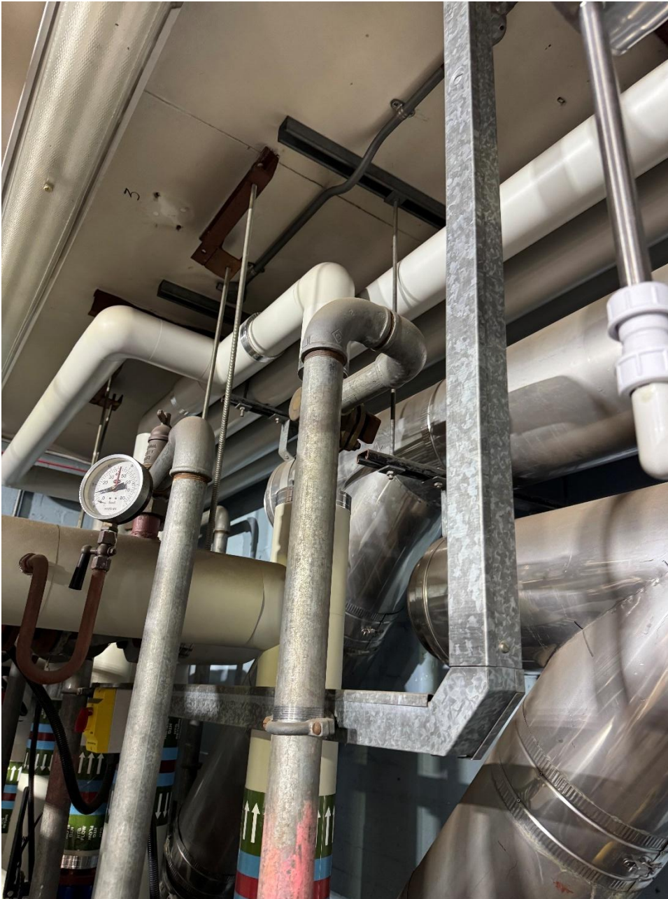
Photograph 23 - The LTHW system was open-vented.
