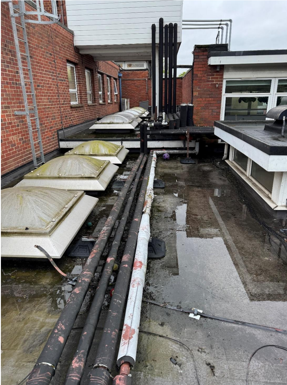
Photograph 32 – LTHW insulation appeared to be in poor condition.
