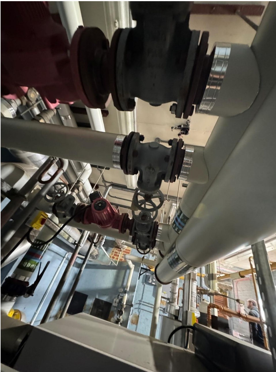
Photograph 25 – Boilers were connected in an “injection header arrangement”.
