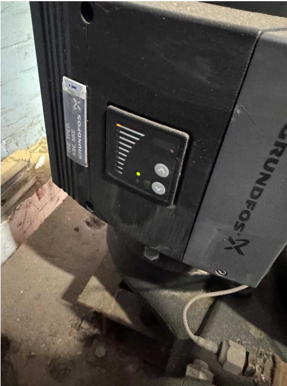
Photograph 11- Pumps were set to high speed but not on the maximum setting.
