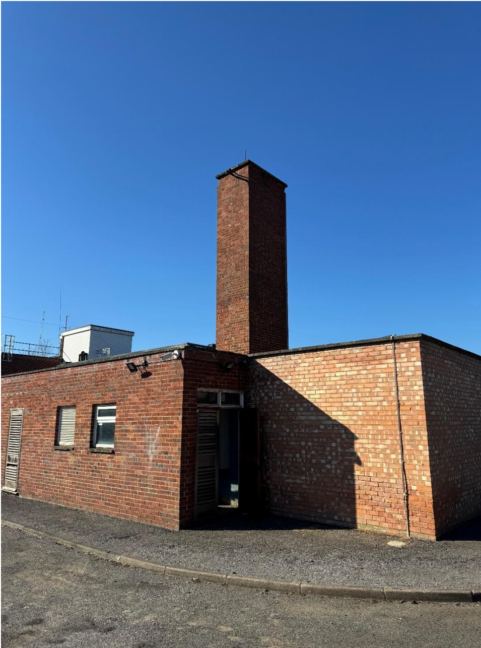
Photograph 24 - External to the plant room. Flue terminate in this chimney.
