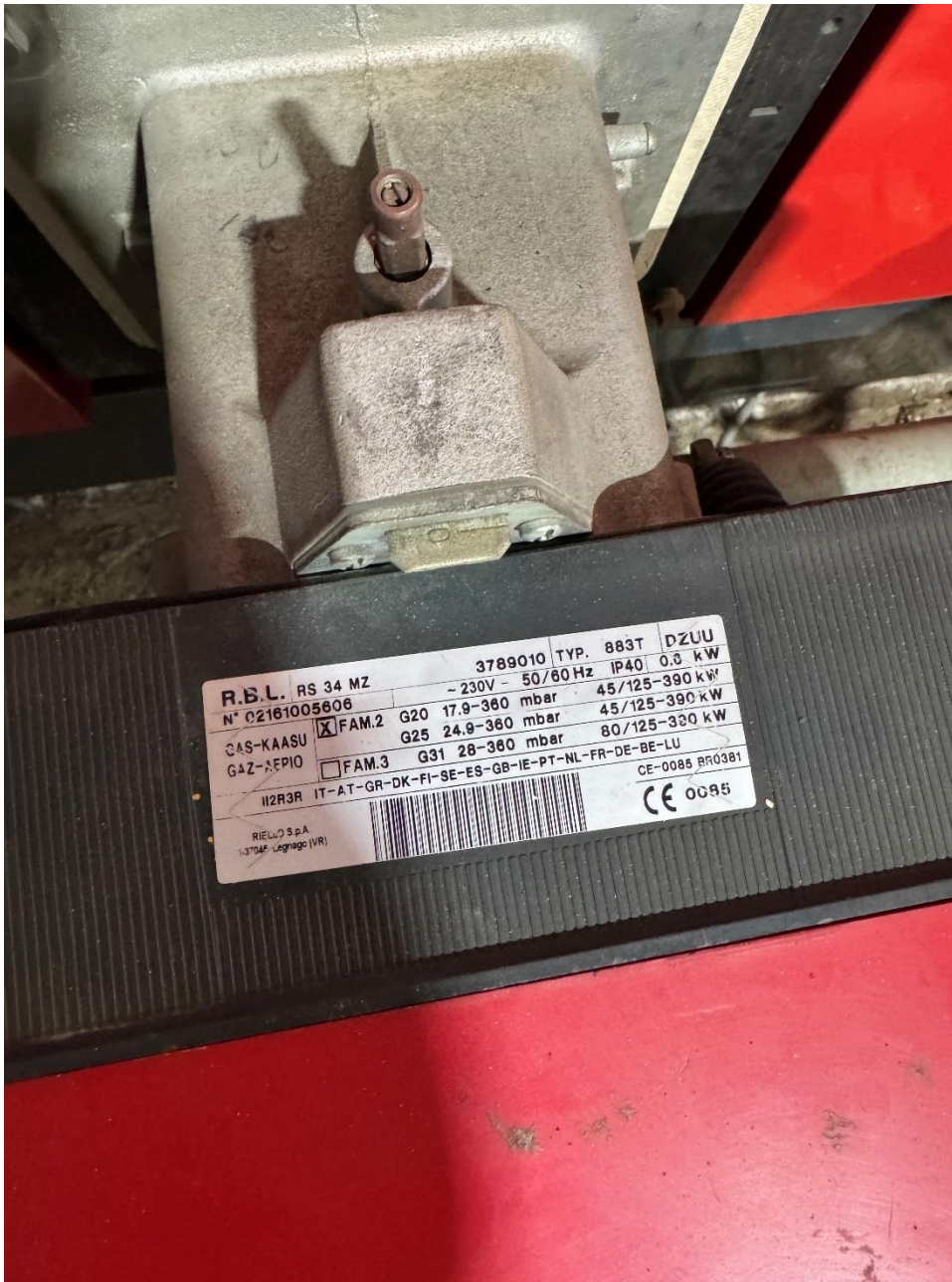
Photograph 18 – Burners are Riello RS34
