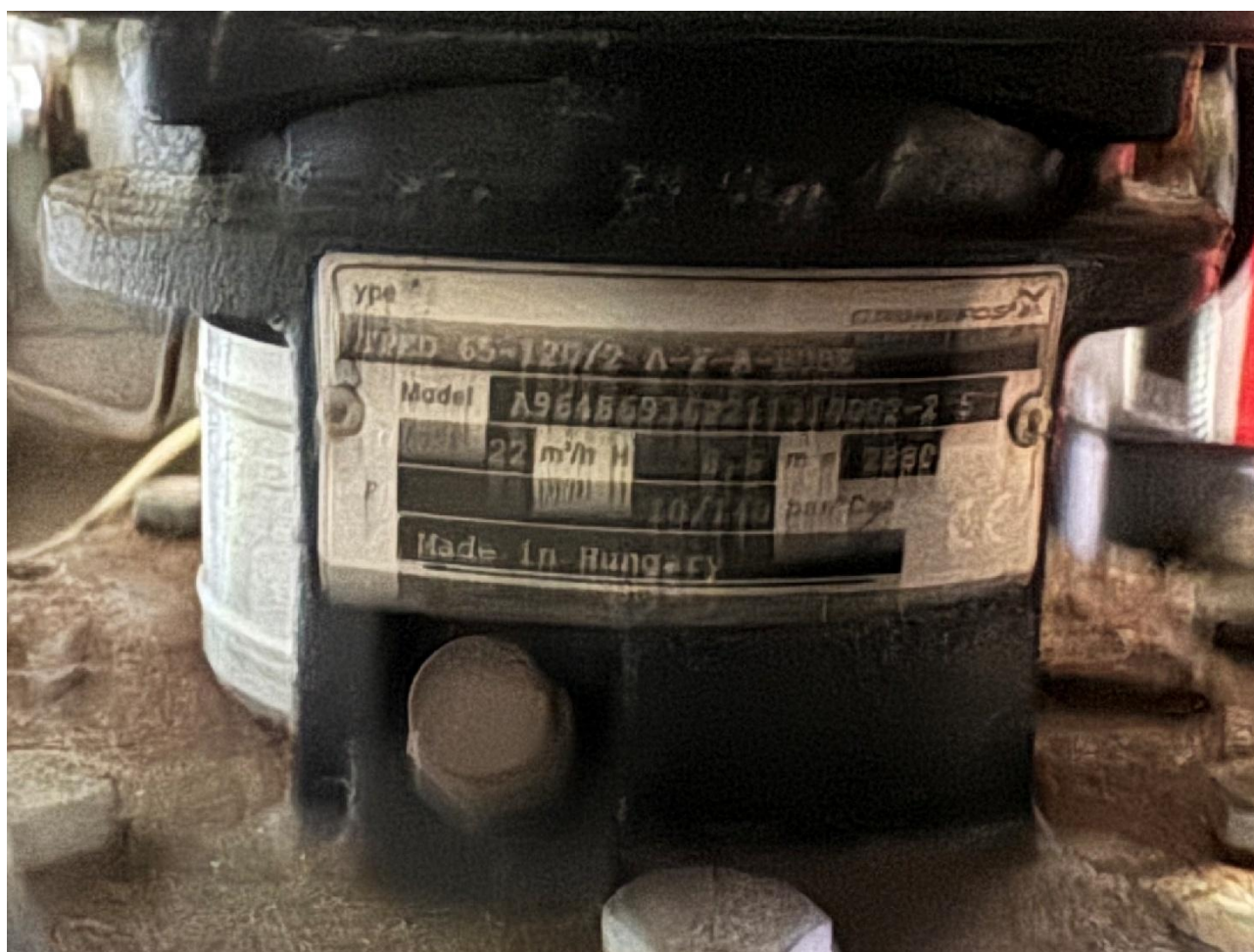
Photograph 14 – Main LTHW circulator TPED 65-120
