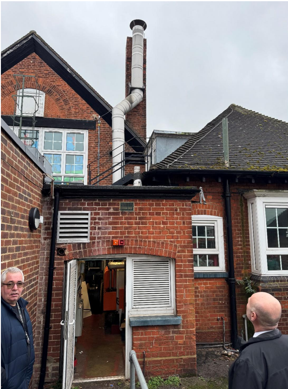
Photograph 9 – Existing open flue
