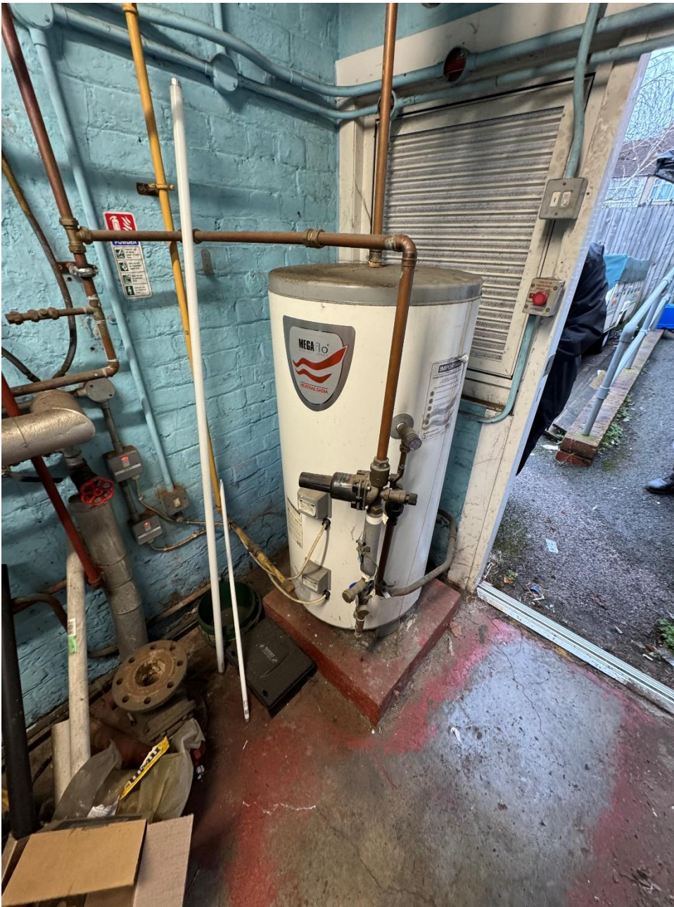
Photograph 6 – Domestic Hot water cylinder
