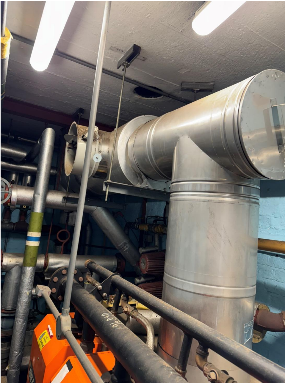
Photograph 10 – Flue internal photograph
