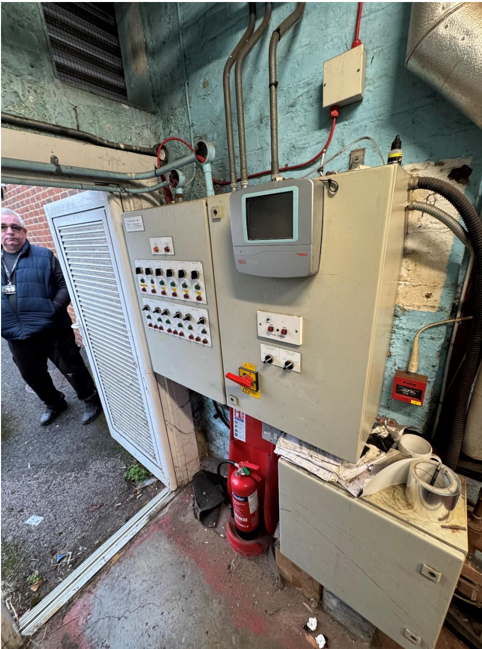
Photograph 5 – Existing obsolete Trend controls and control panel
