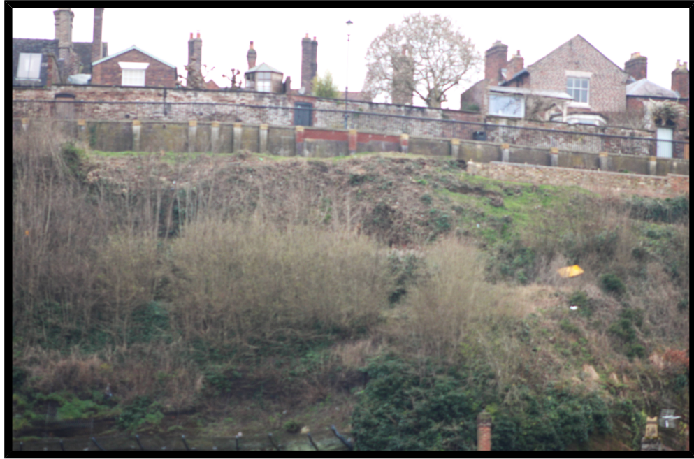
Landslip Zone Area of movement due to failed lower retaining wall
