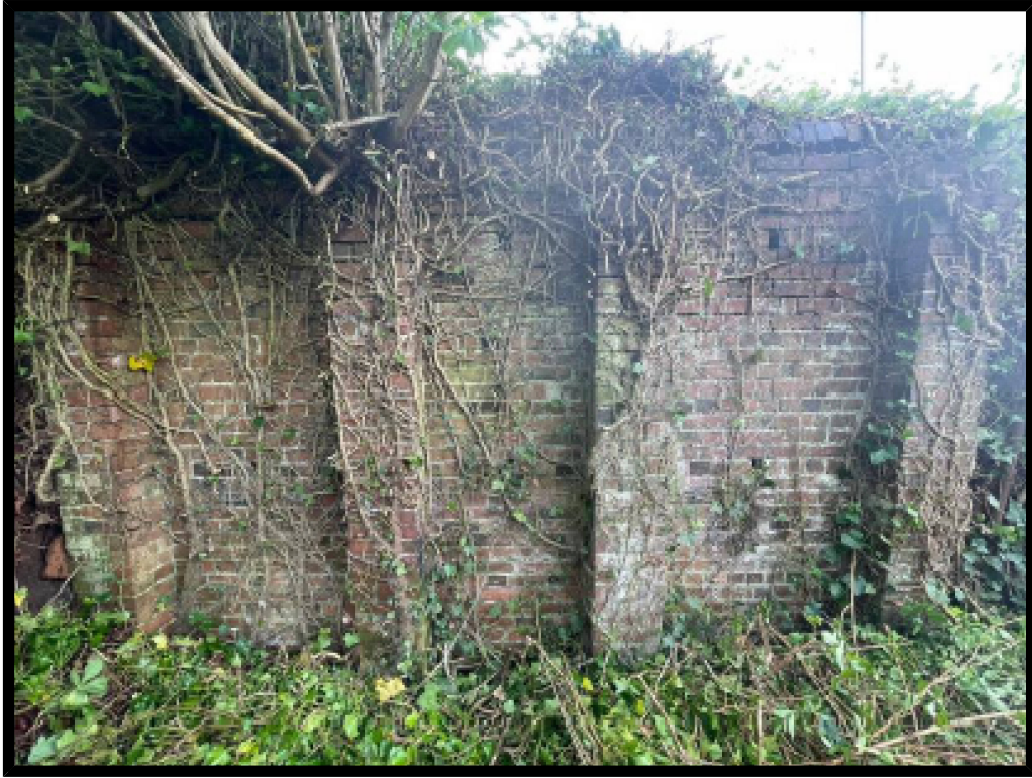
Lower Retaining Wall To be restrained
