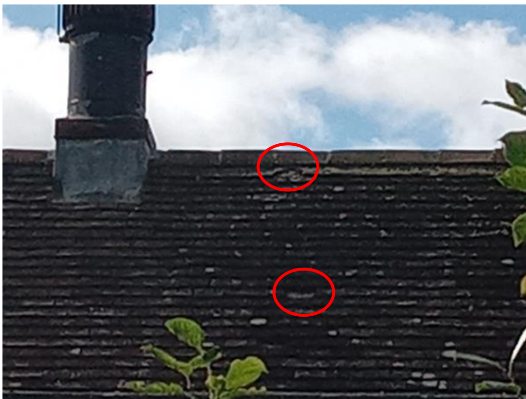
Photograph 4. Broken/misplaced roof tiles on the main building (Target Note 2).
