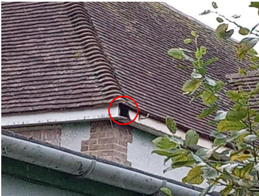
Photograph 4. Broken/misplaced roof tiles on the main building (Target Note 2).
