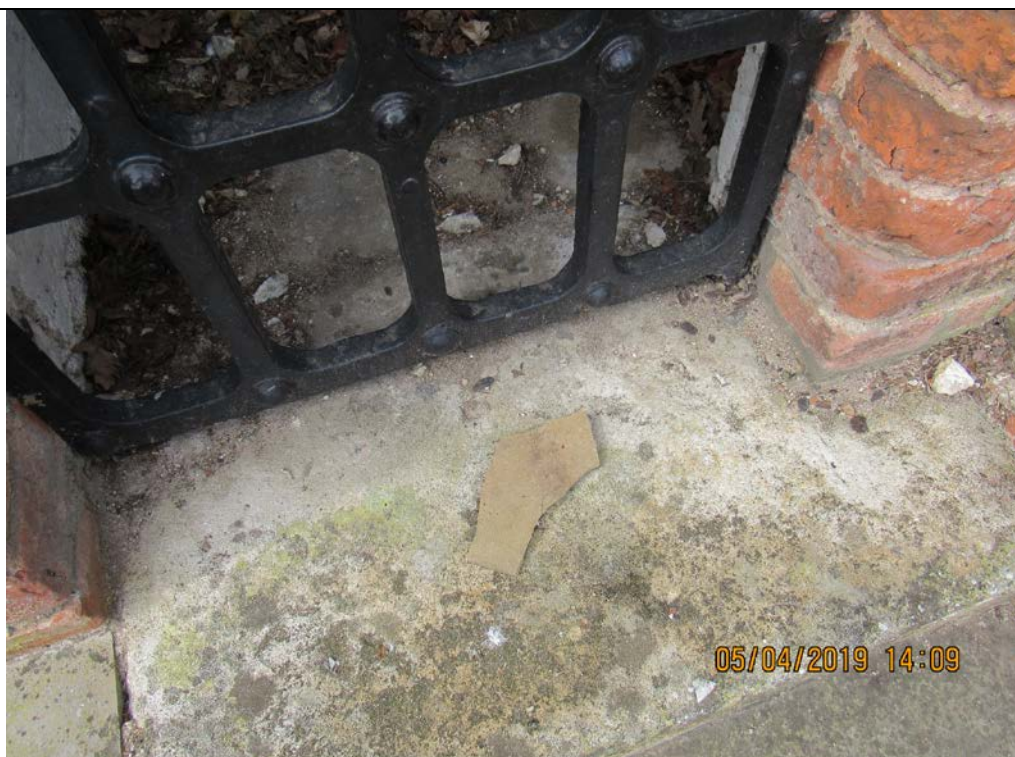
Photograph E7 Another piece of fallen masonry outside one of the front Gaols.
