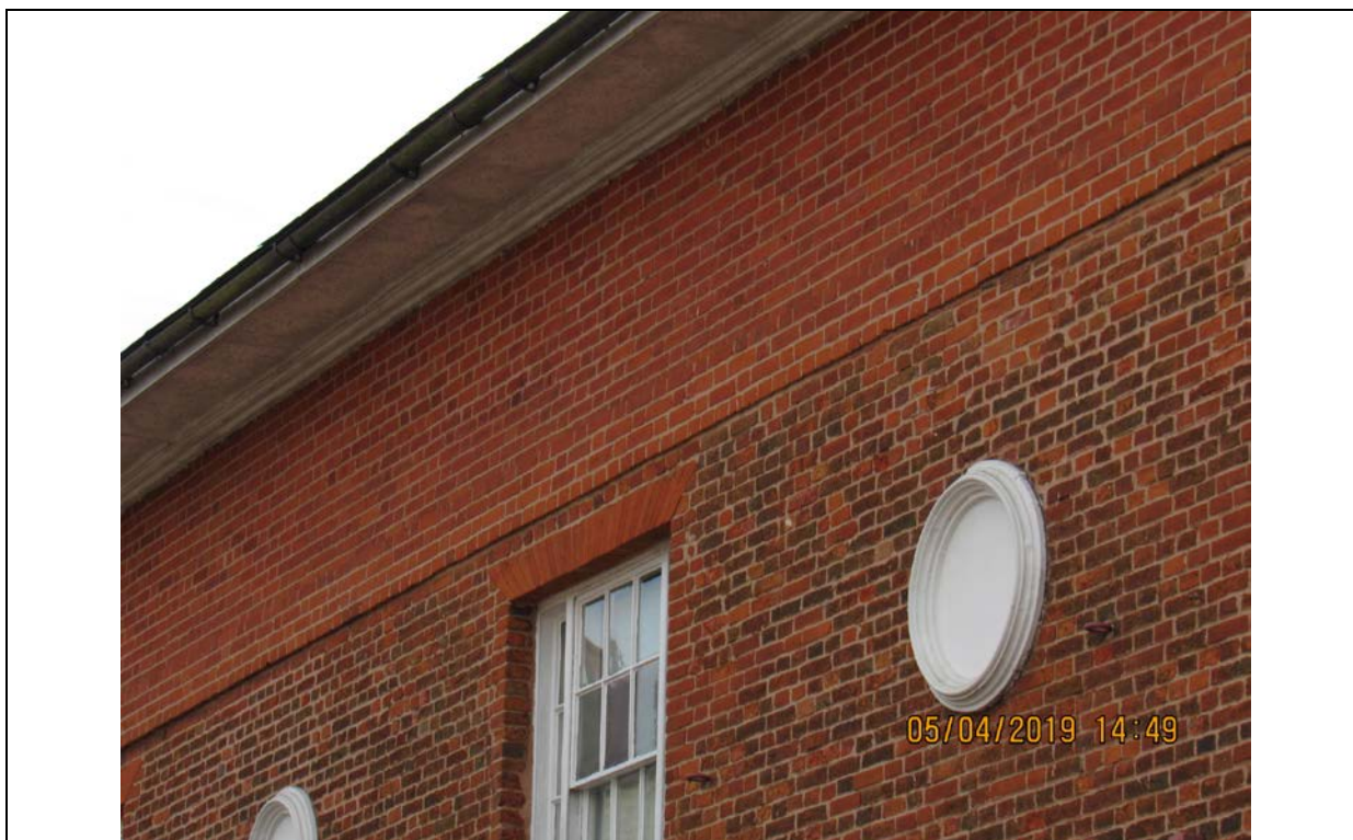
Photograph 03 Side Elevation showing band of repaired brickwork at Eaves level.
