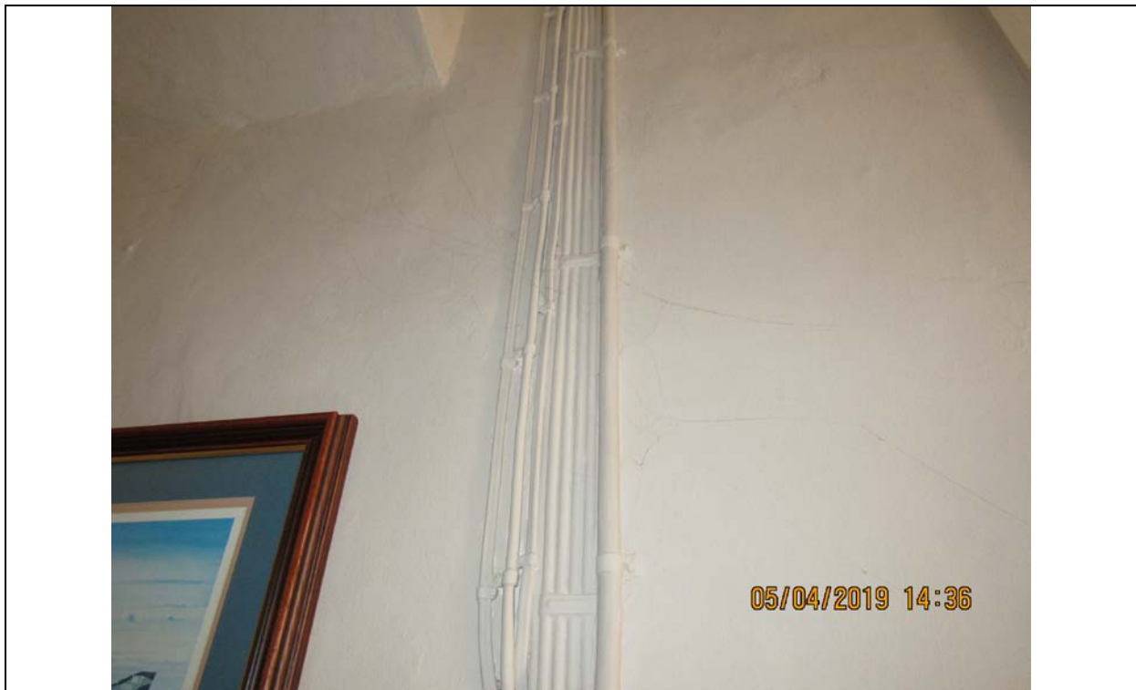
Photograph 51 Exposed internal wiring
