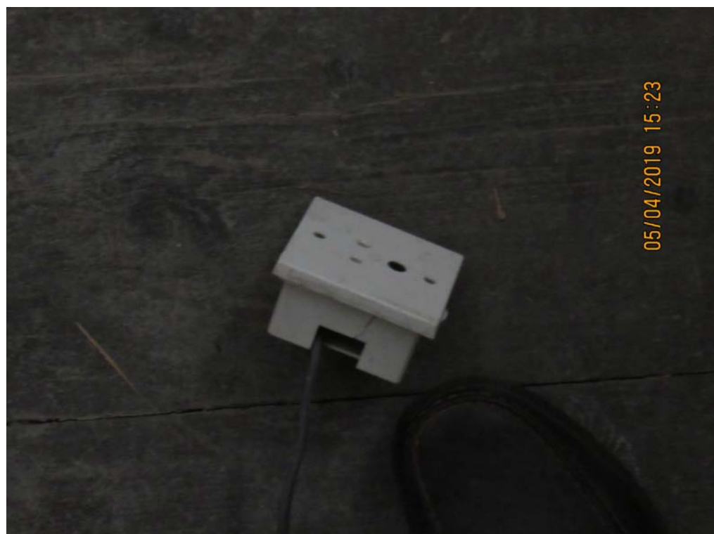
Photograph 39 Loose socket and exposed wiring
