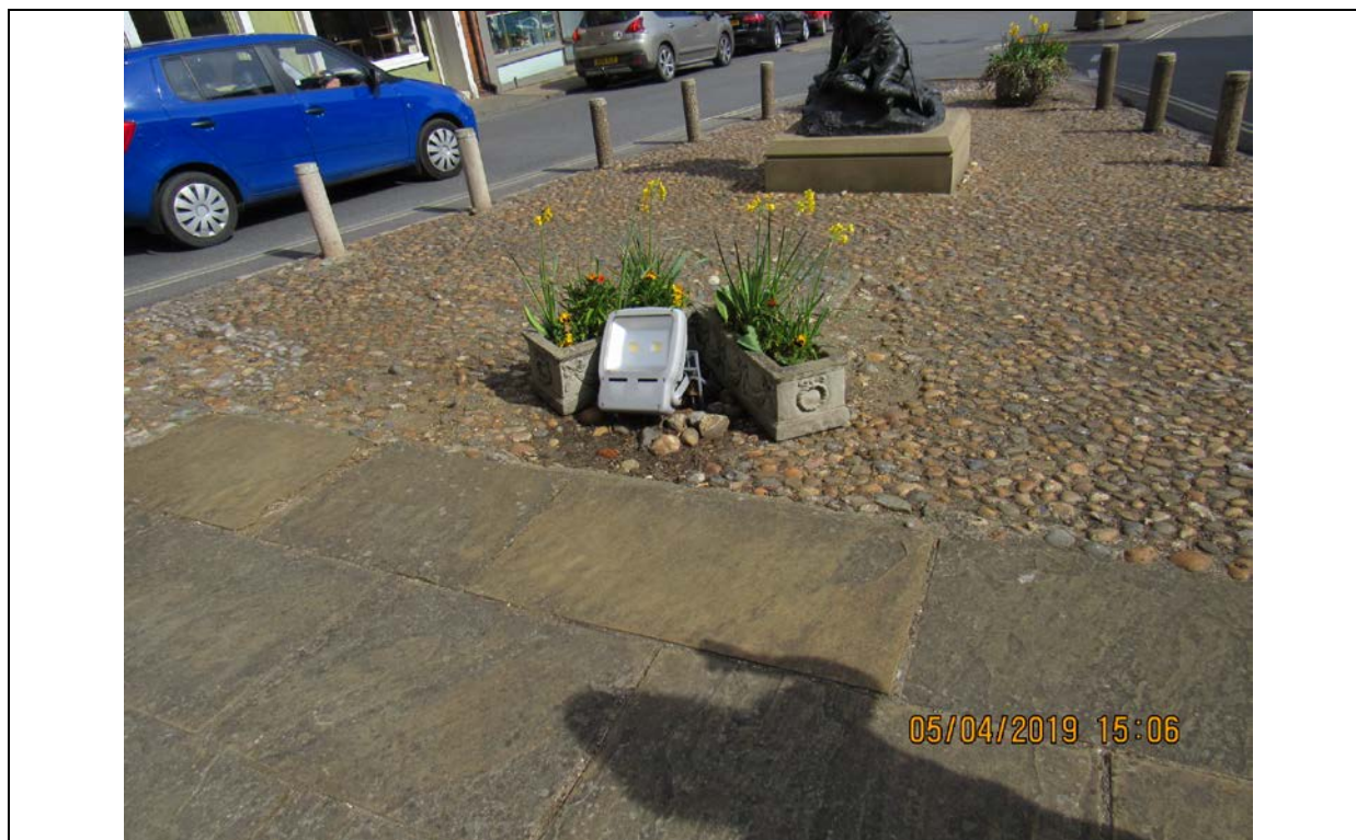
Photograph 41 Unguarded external flood lamp at Ground level
