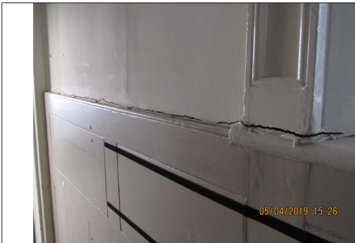
Photograph 20 Internal cracks extending along wall
