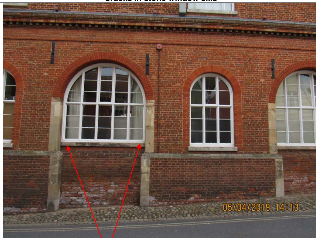
Photograph 11 Previously repaired sills
