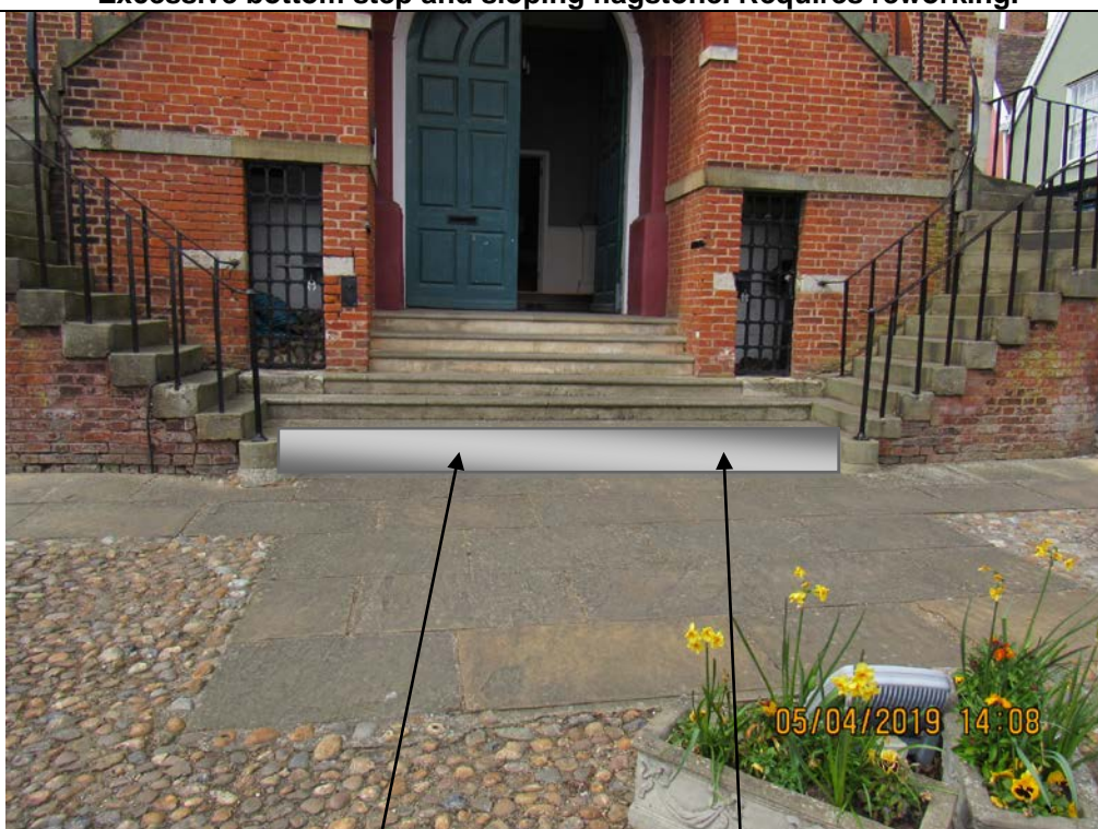
Photograph E4 Suggest full width infill.
