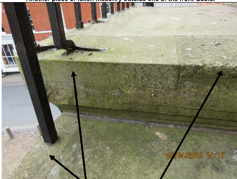
Photograph E8 At least 2 no separate repairs visible to Balcony Stonework.
