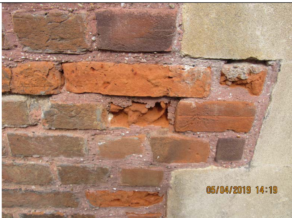
Photograph 47 Delaminating brickwork to south elevation.
