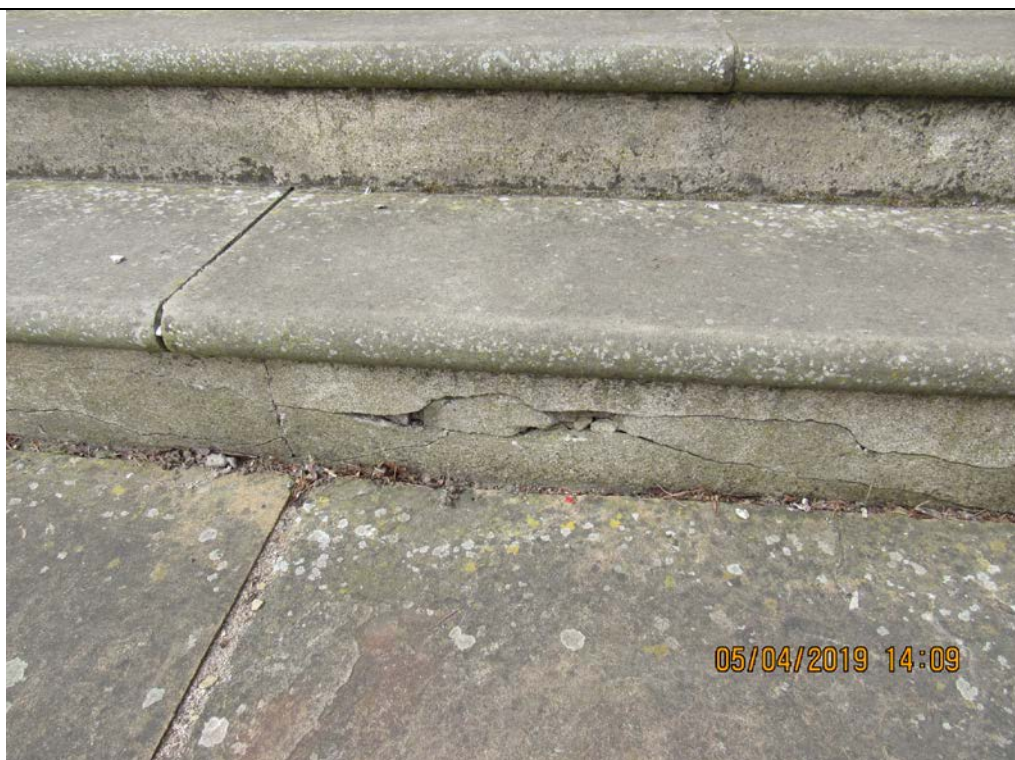
Photograph E5 Cracked and loose render.
