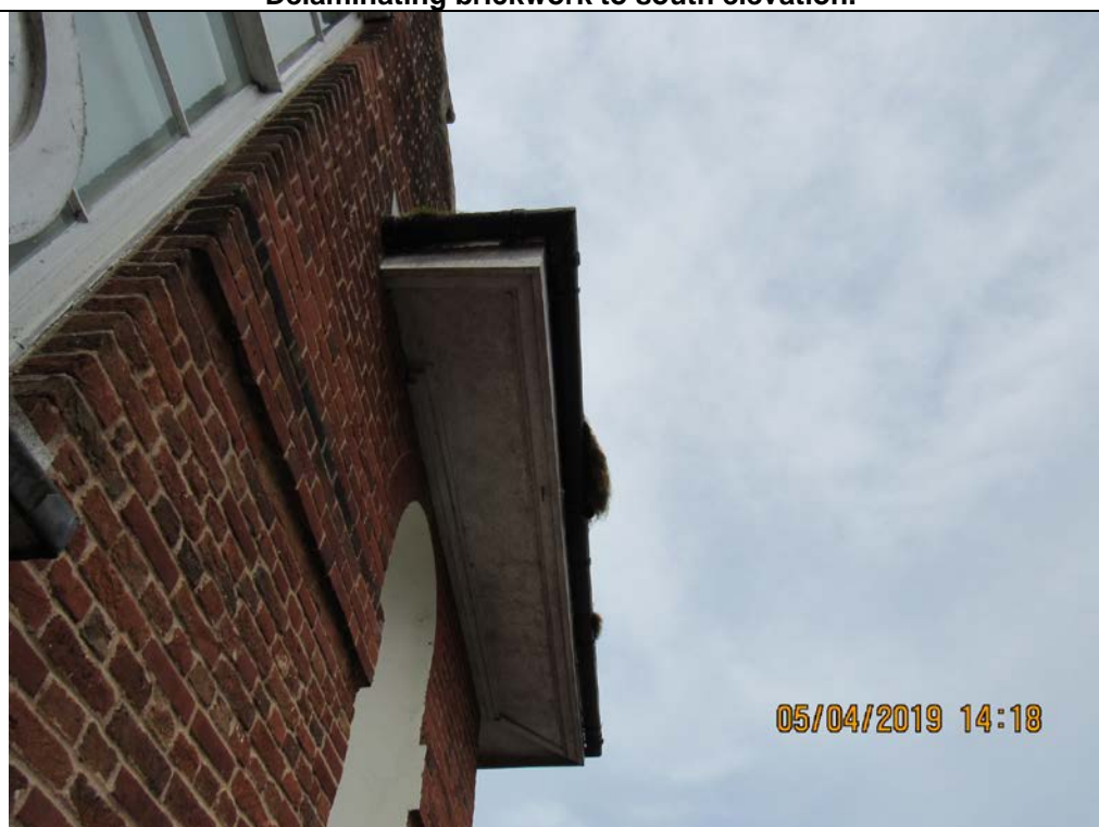
Photograph 48 Clear gutters of vegetation.
