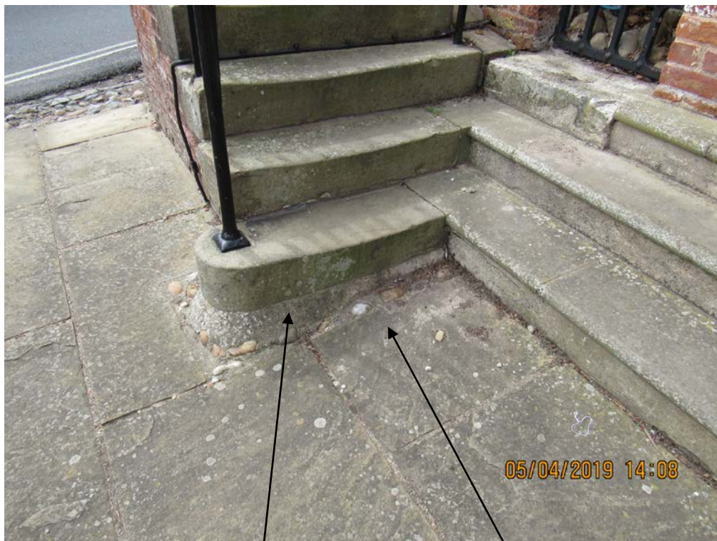
Photograph E3 Excessive bottom step and sloping flagstone. Requires reworking.
