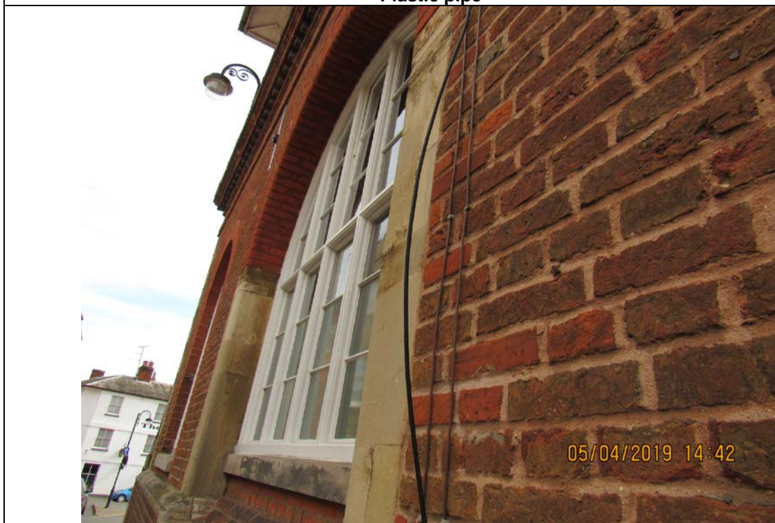
Photograph 27 External loose wiring
