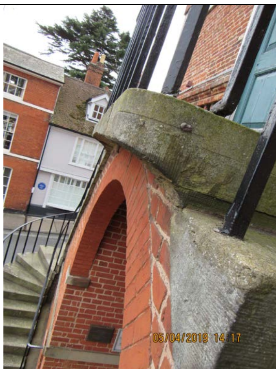
Photograph E9 Stone balcony spanning onto brick arch.
