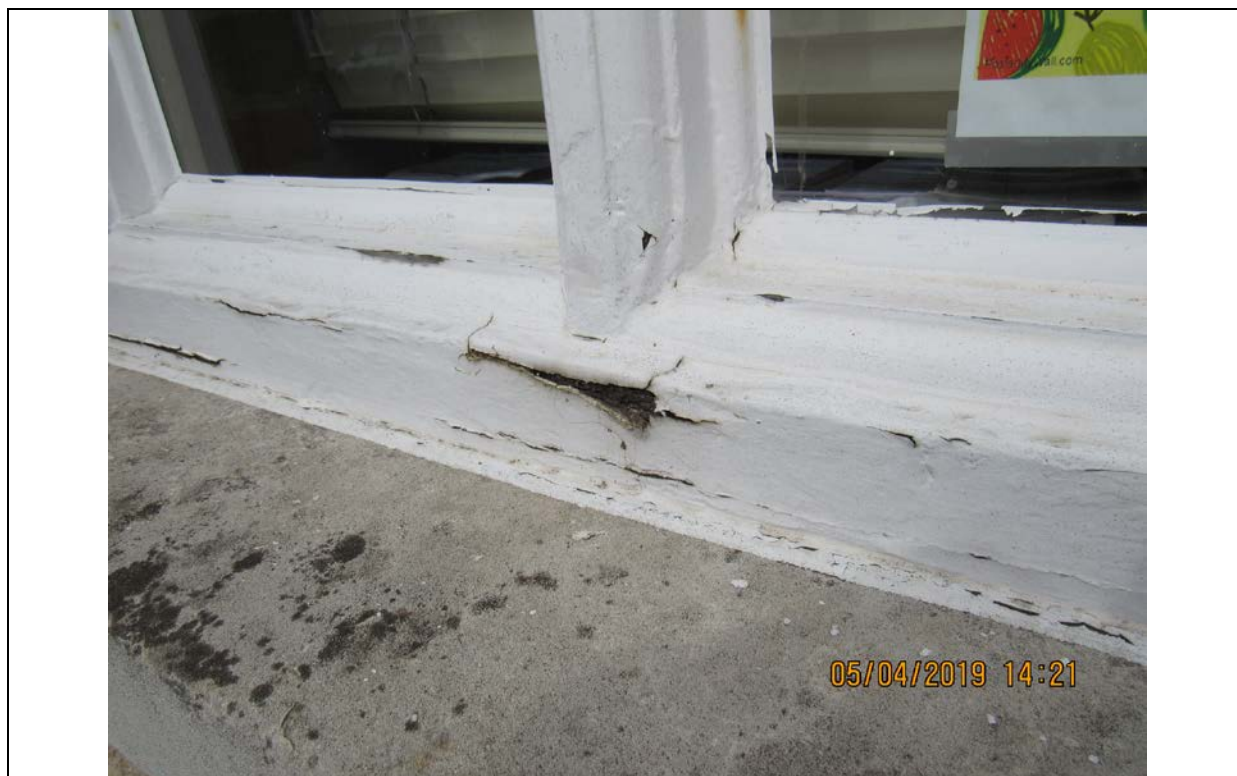
Photograph 31 Window frame beginning to decay
