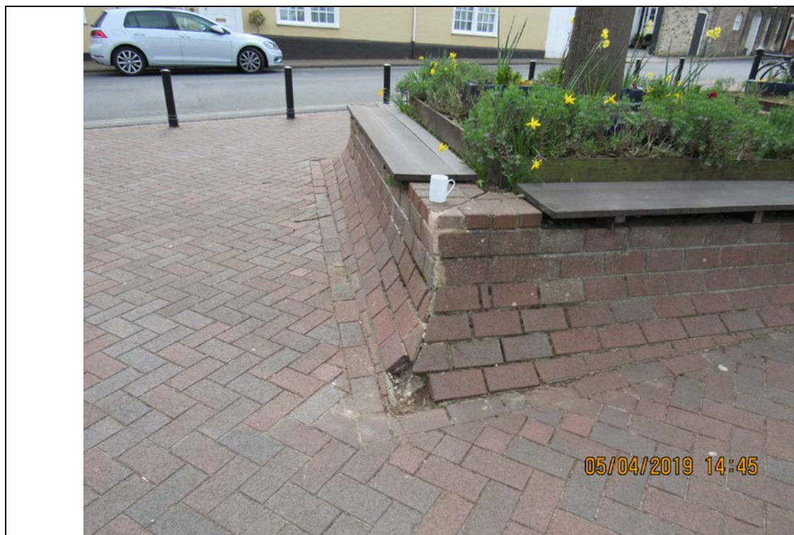
Photograph 45 Missing block paving exposing sharp point.
