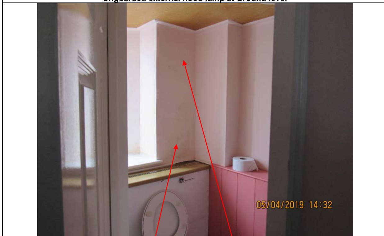
Photograph 42 Damp patches
