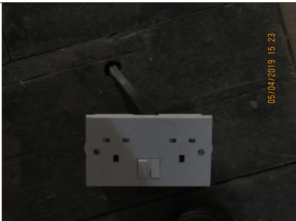
Photograph 39 Loose socket and exposed wiring
