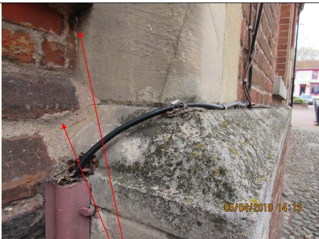
Photograph 05 Infill brickwork butting up to original stone quoins
