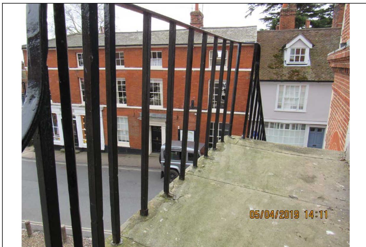
Photograph 18 The existing balcony is only 900mm (3feet) high and not 1100mm
