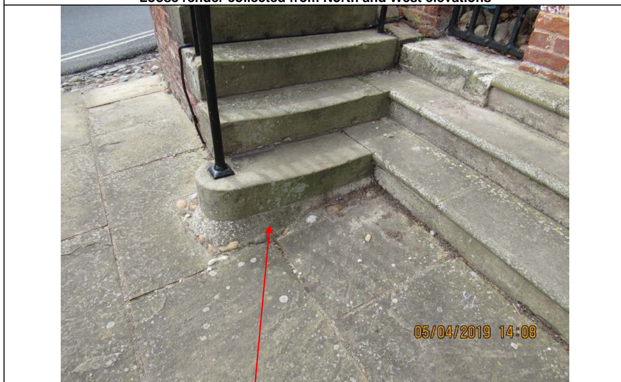
Photograph 36 Excesses bottom step compared to others
