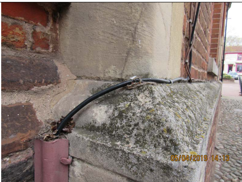
Photograph 28 External wiring
