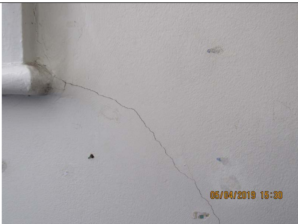
Photograph 24 Diagonal Cracks leading from corner of window
