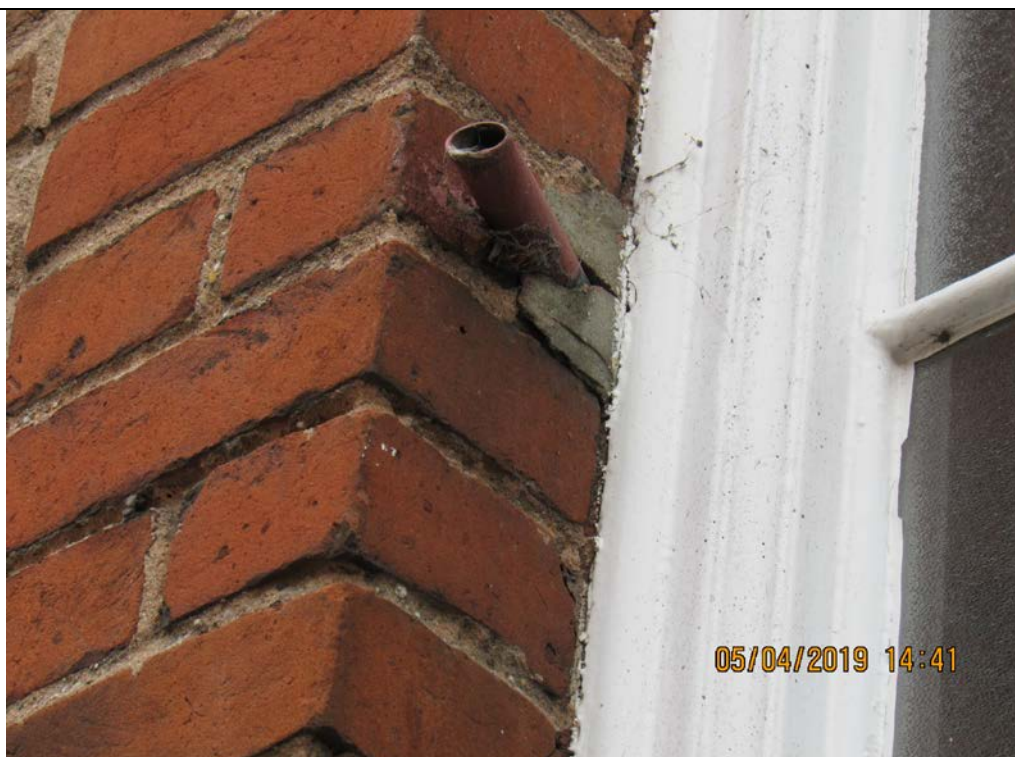
Photograph 43 Pipe outside corresponding to damp patches
