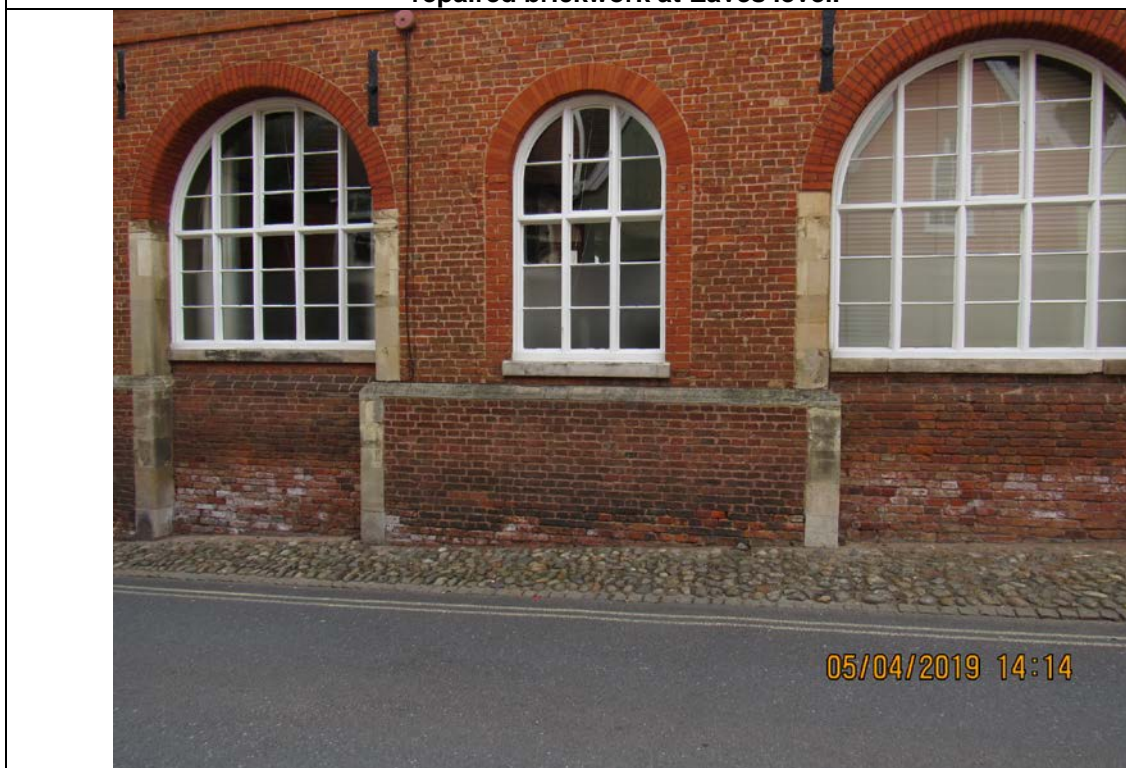
Photograph 04 Original Stone quoins either side of brick infills.
