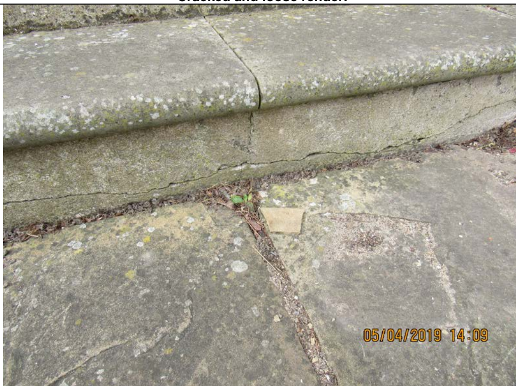
Photograph E6 Fallen masonry seen at time of visit on ground outside of front entrance.
