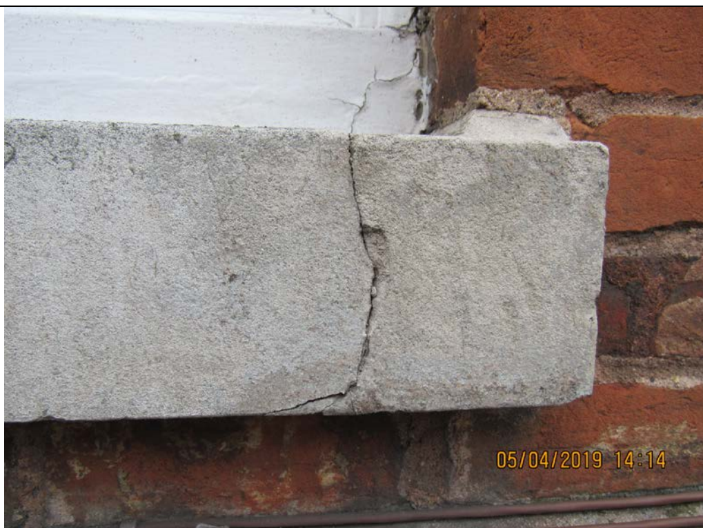
Photograph 10 Cracks in stone window sills
