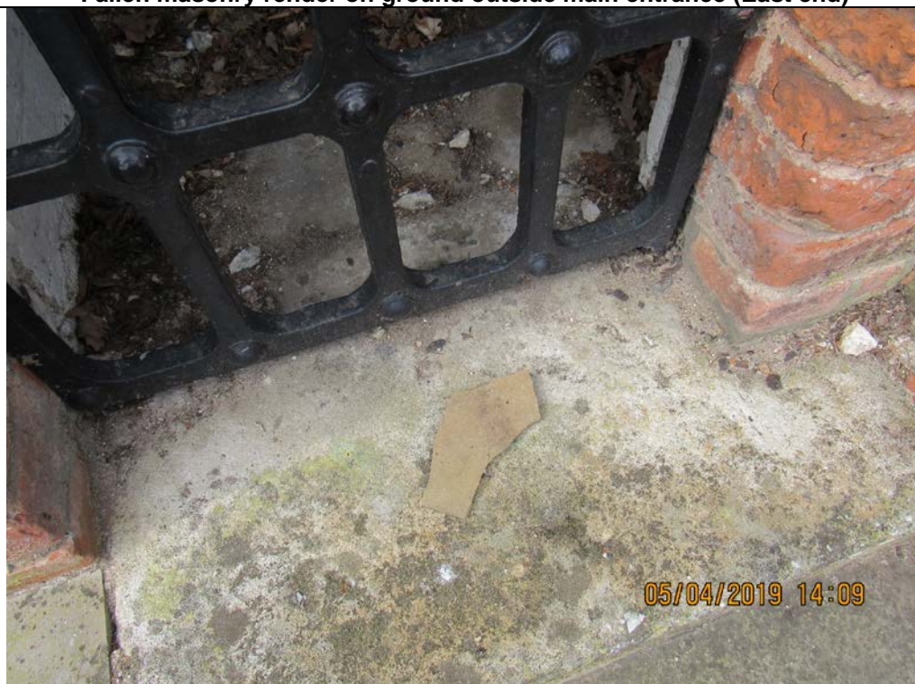
Photograph 34 Piece of render on floor (East end)
