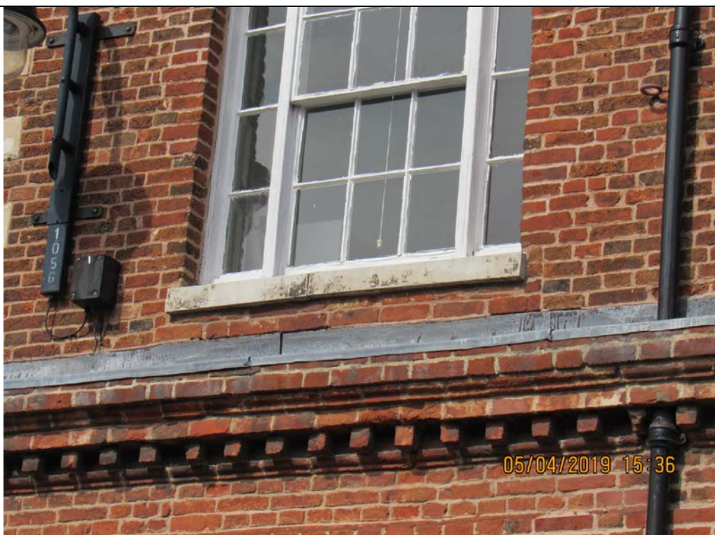
Photograph 12 Cracked window sill on upper floor.
