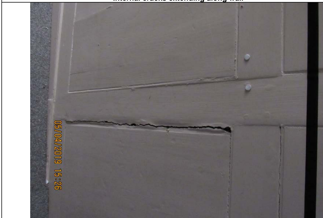
Photograph 21 Cracks in panelling
