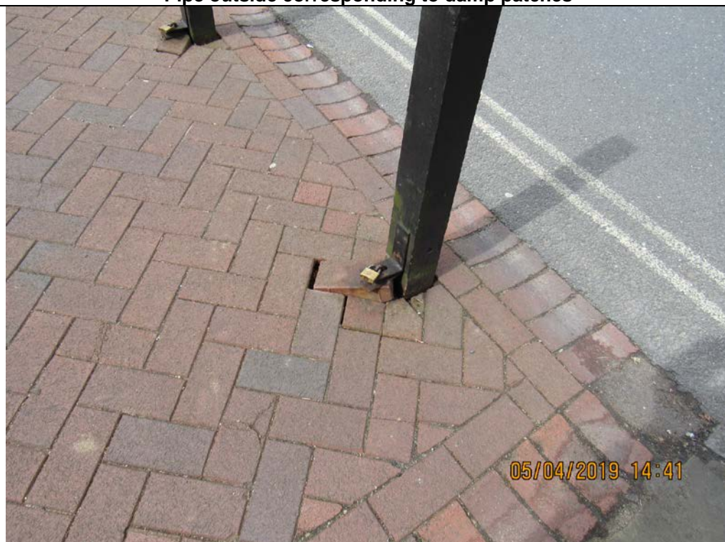
Photograph 44 Protruding paving block (over 50mm protrusion)
