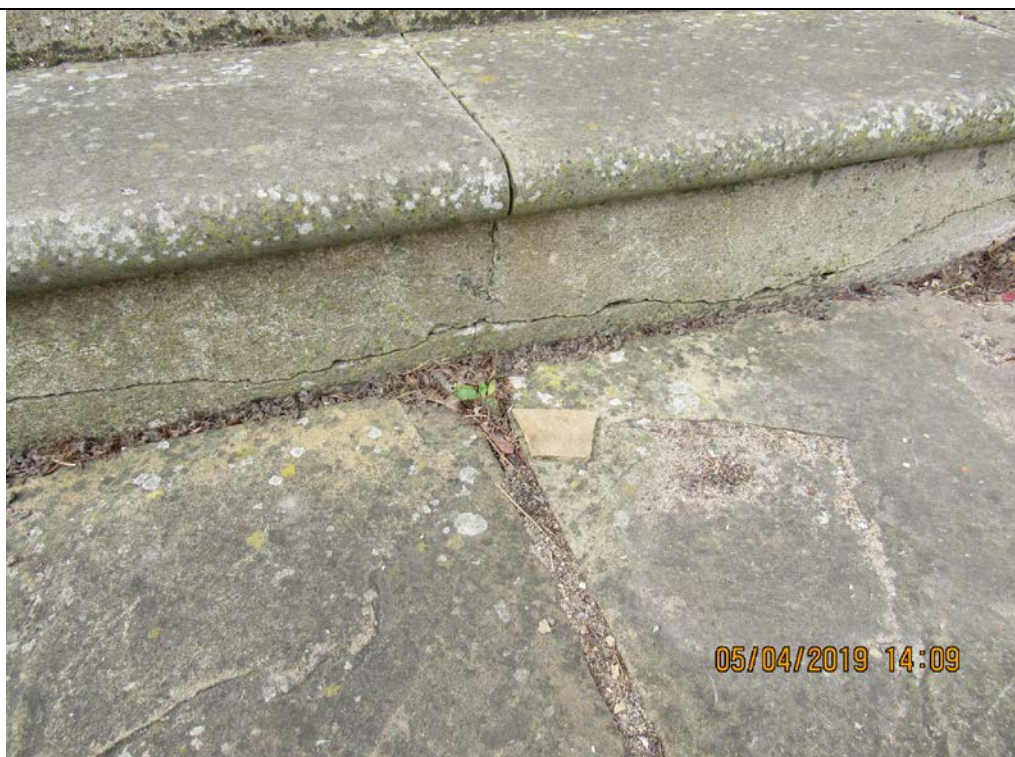
Photograph 33 Fallen masonry render on ground outside main entrance (East end)
