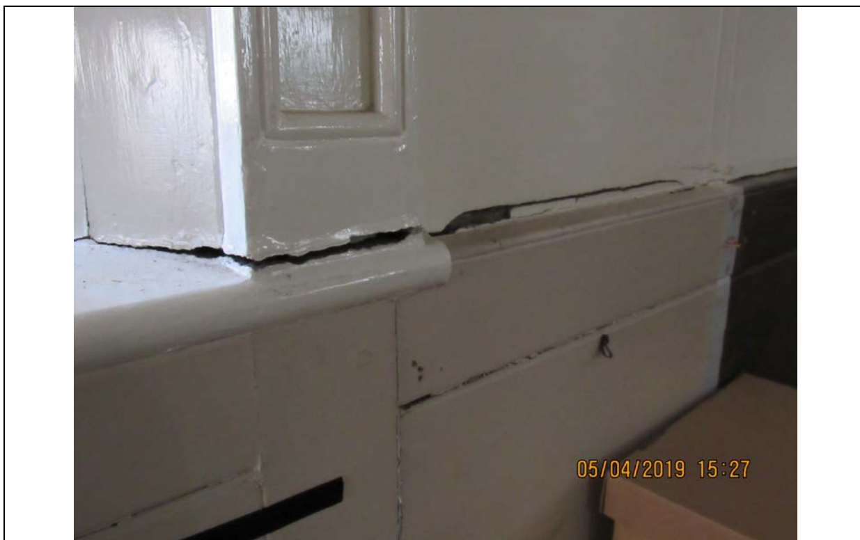
Photograph 22 Similar Cracks the other side of the window.
