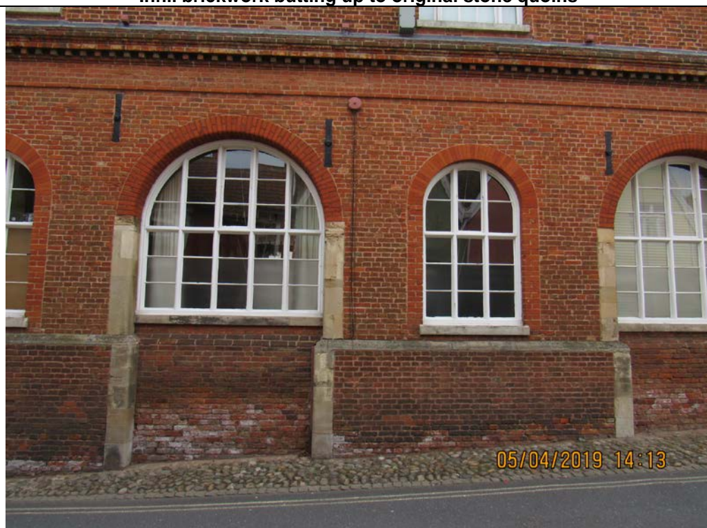
Photograph 06 Larger brick arches springing off original stone quoins. Smaller windows clearly cut in later.
