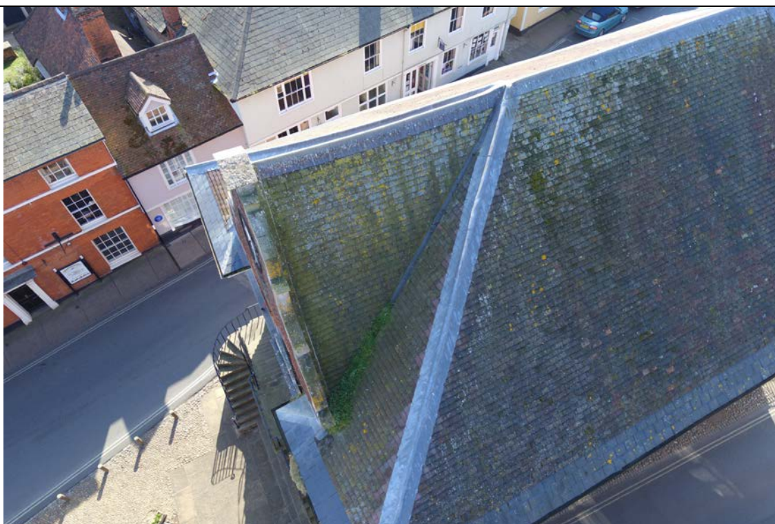
Photograph 49 Vegetation in valley gutter.
