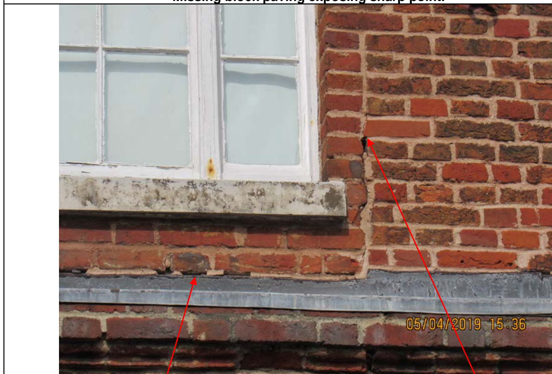
Photograph 46 Poor brickwork around upper windows and missing mortar (North wall)
