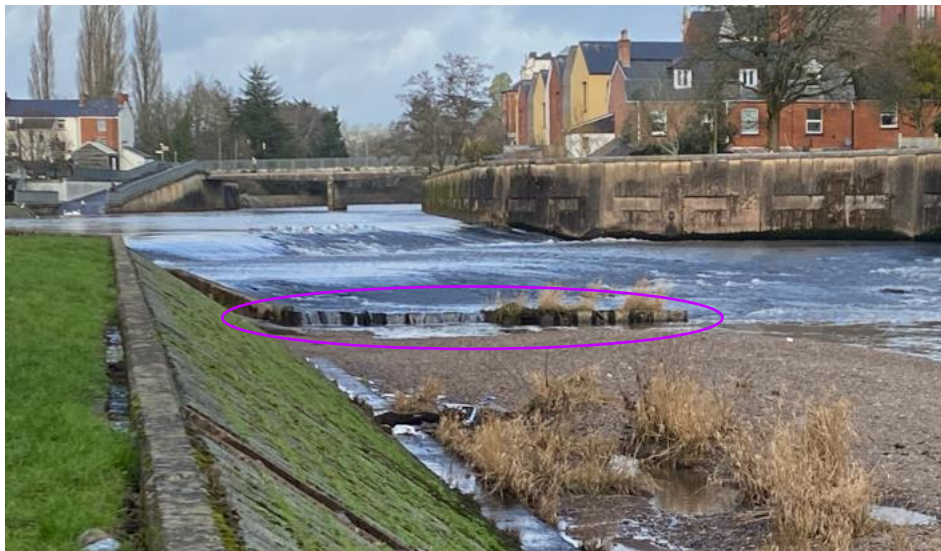
Figure 4 - Photograph looking upstream showing the section of sheet piling downstream of the weir, encircled in pink
