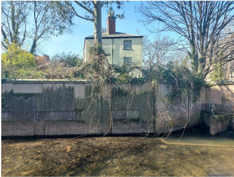
Figure 11 - View of flood wall 3, with the flap valves at Heathcoat Mill visible on the left
