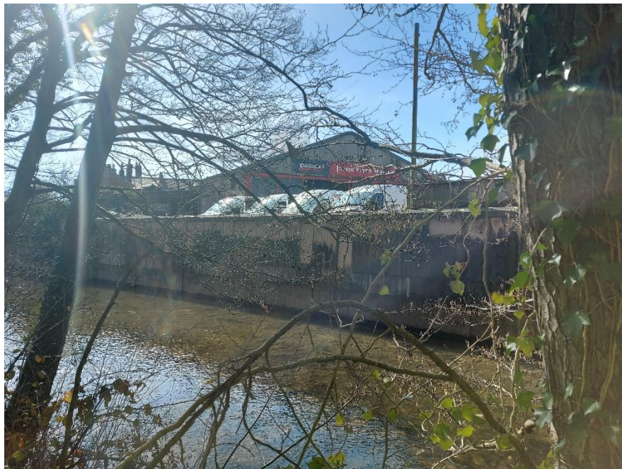
Figure 12 - View of flood wall 2
