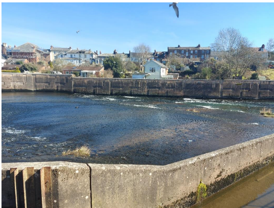
Figure 14 - View of River Exe, just downstream weir looking across stop log structure at flood wall 4
