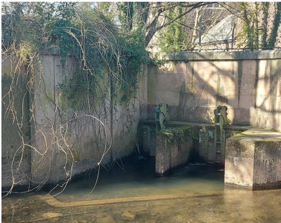
Figure 8 - Photograph showing two sluice gates on Heathcoat Mill leat
