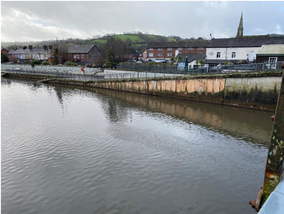
Figure 15 - View looking downstream at flood walls 1, 2 (no river frontage) & 3, and at the slipway into the river
