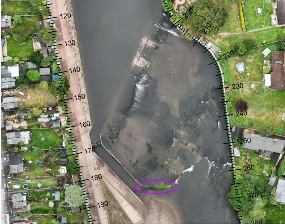
Figure 3 - Extract from chainage drawing 01 showing the section of sheet piling downstream of the weir, encircled in pink.
