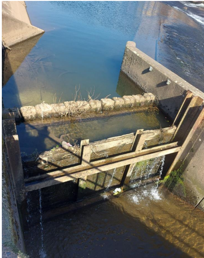
Figure 6 - Photograph of stop-log structure adjacent to weir
