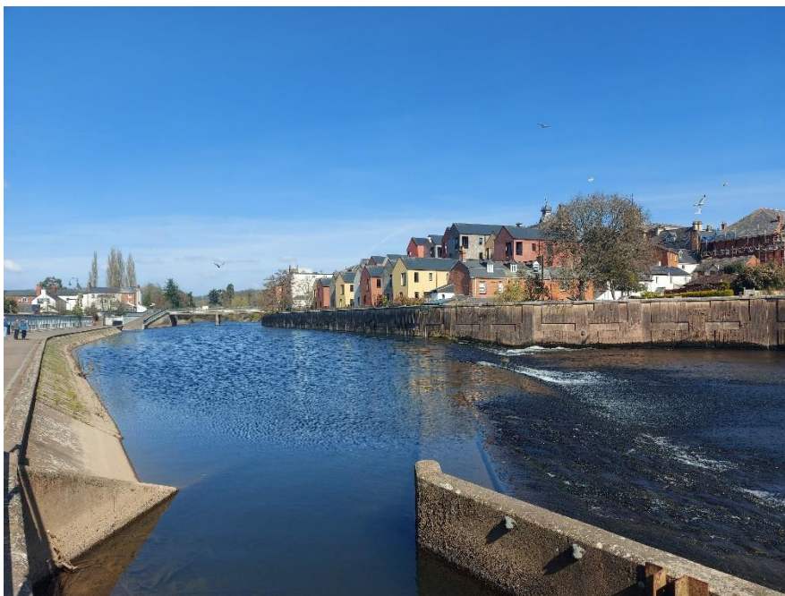
Figure 13 - View of River Exe looking upstream, across the weir and at floodwall 4
