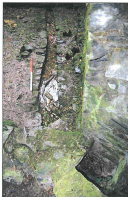
Plate 14: Drain in north wing and garderobe drain of Betsy Grimal's Tower, looking northeast. (1m scale)
