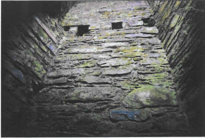
Plate 24: Joist sockets in north turret for first-floor of Betsy Grimal's Tower, looking west-southwest
