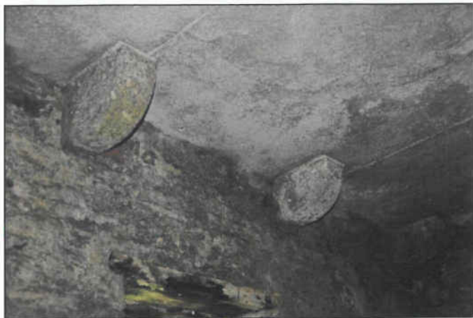
Plate 39: Detail of first-floor corbels on west elevation of the Still House, looking east. (1m scale)
