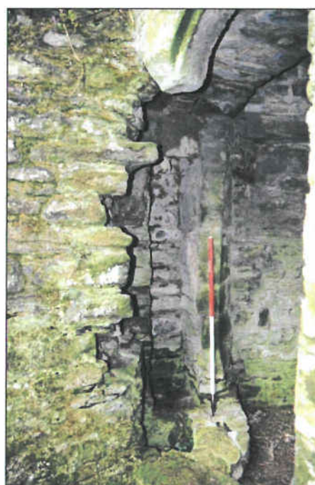
Plate 16: Exposed drain of first-floor Garderobe in ground floor garderobe of Betsy Grimal's Tower. (1m scale)
